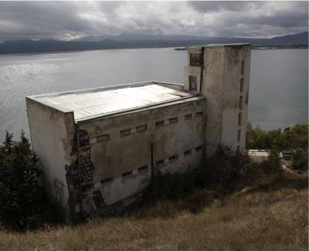
Picture 92. Northern elevation of the Residence Hall building, 2016.
