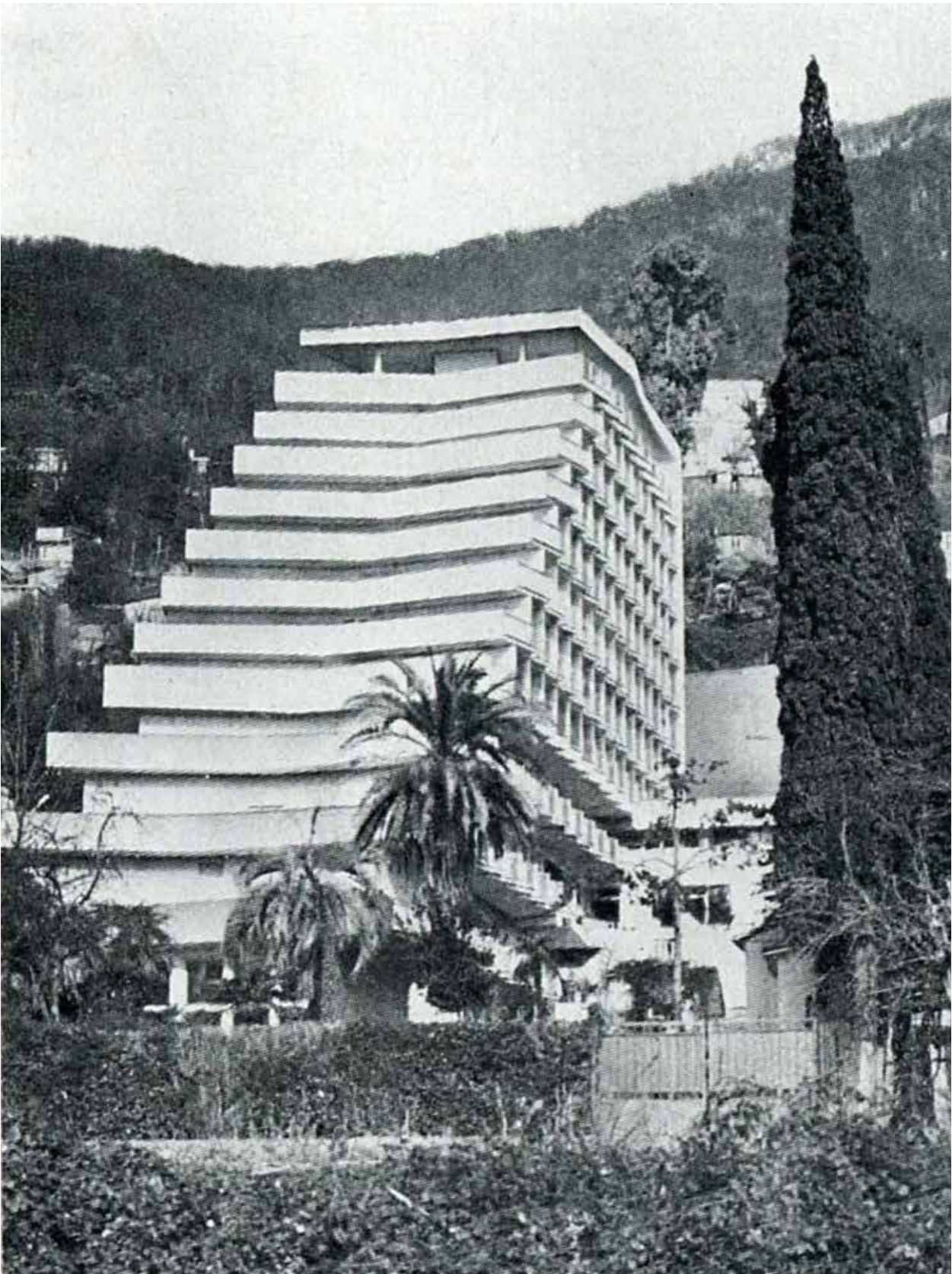
Picture 11. Resort of the Union of Architects in Gagra, 1980
