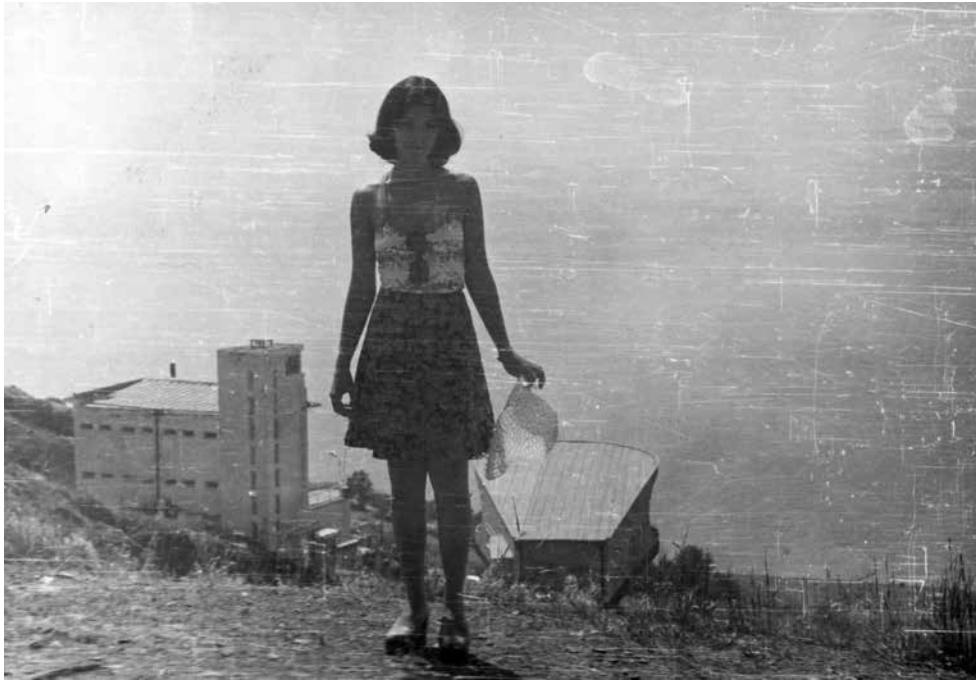
Picture 59. View of the resort from the monastery
