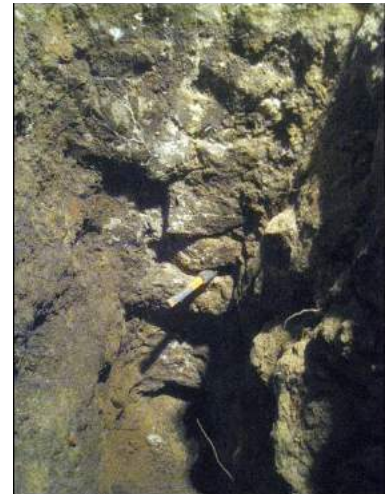
Pit 1. Lower footing. A chisel points out depth of the washed out mortar
