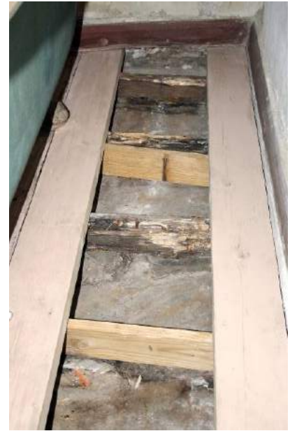
Opening behind the bath. Visible rotten battens and new battens, temporarily replacing them.
