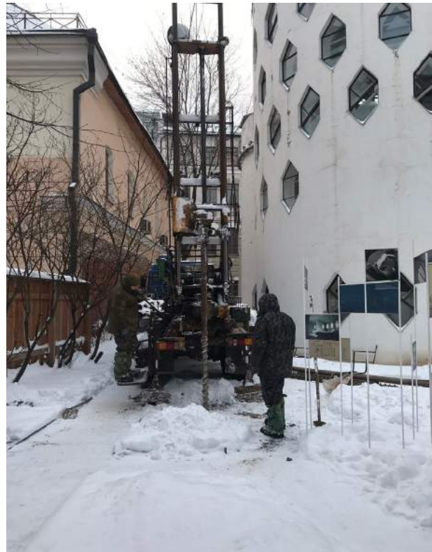
Well 1 in process of drilling. North-east from the House, 2018
