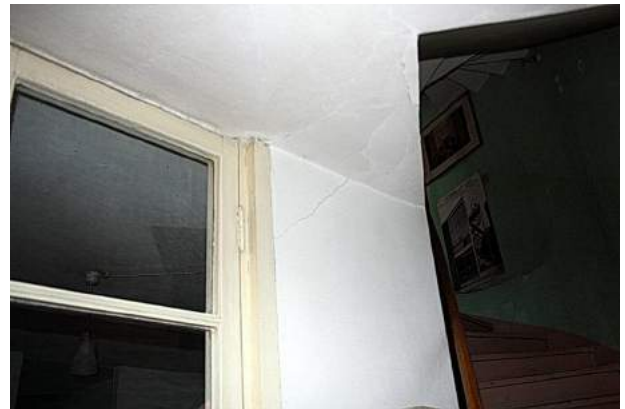
Cracks in the plaster layer of the wooden partition and ceiling
