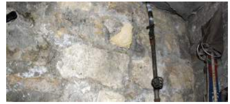
Surface of the exterior walls of the basement. Traces of efflorescence on masonry
