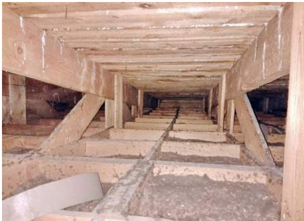
Roof of the large cylinder, general view of structures Unevenness of insulation in the cells of the attic floor, presence of construction debris (scraps of tinplate).
