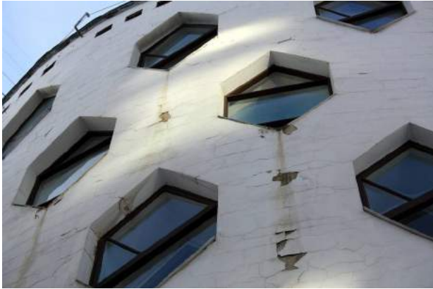
Water stains under windowsills, cracks, damage to the finish, traces of repairs. It is clearly visible that exterior windowsills differ in shape and width of their projection
