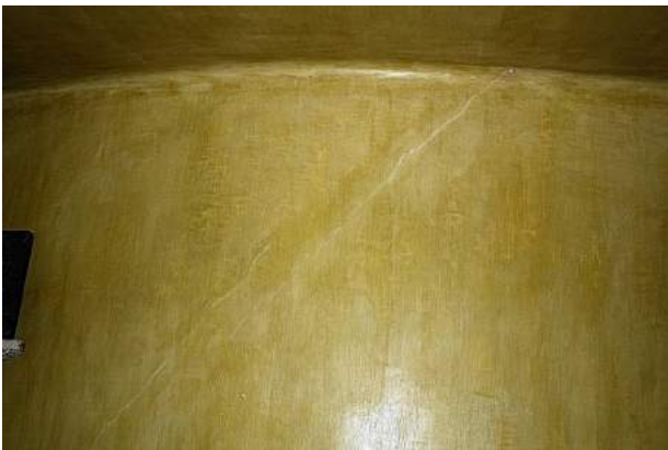
Diagonal cracks in the semicircular partition of the bedroom
