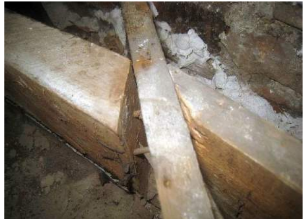
Inaccurately cut rim joist. Loosening of nailing.
