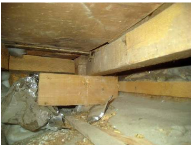
Space under the tread. There is a supporting board between the tread and the floor boards on the right
