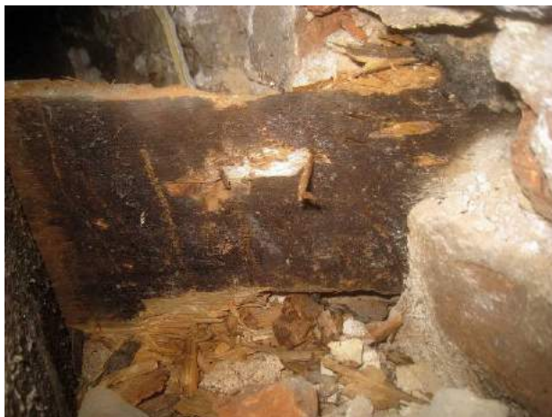
Damage by rot of the supporting ends of joists of the ground floor grid. The only joists damaged are those, that are built in the masonry of the walls. In the photo: the joist is mostly peeled off from weak wood.
