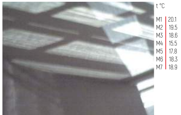
Thermal image. Fragment of the upper part of the southeast wall. 1st floor, the living room
