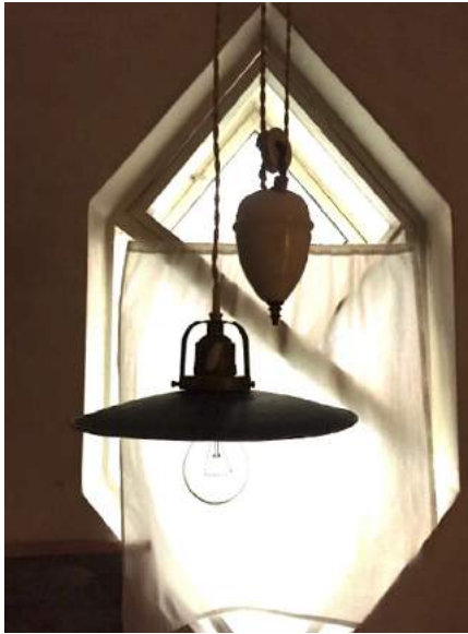
Lamp of 1920s with load and block system. Utility room. Ground floor
