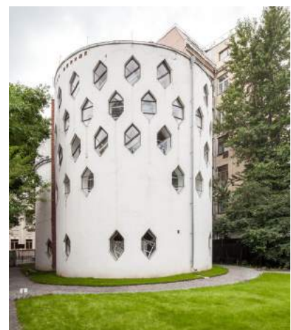
View of the northeast façade. 2016. Photo by D. Esakov
