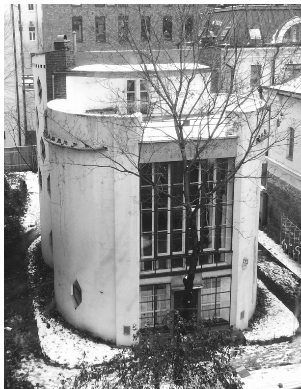
The Melnikov House. Street facade, view from the southwest
