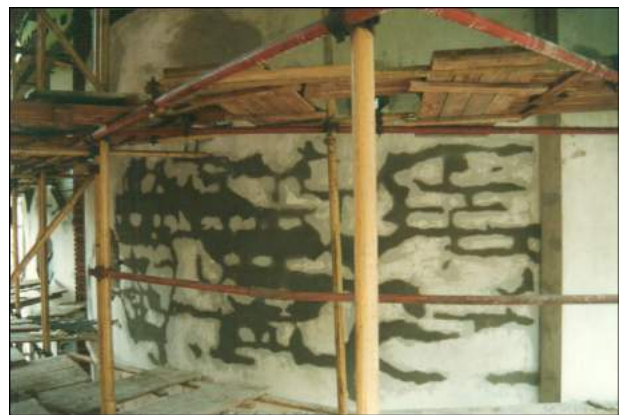
Restoration of façades. 1996
