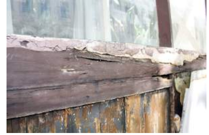
Rot on the lower frame of the large window (in some places it can be pierced with an awl), on the frame under the large window. Surface rot on the wooden filling of the frame under the large window.
