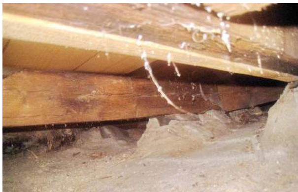
Place of the opening of the inclined reinforced concrete screed is seen between the battens.
