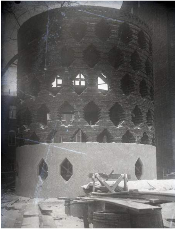
View of the large cylinder from the northeast. 1928
