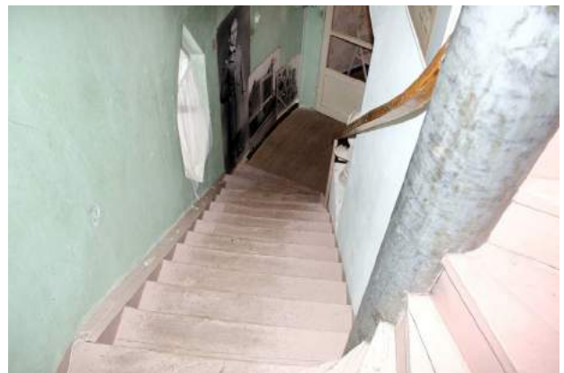
Main staircase between the ground and the first floors. Deflection and deterioration of steps in passing places, wear out of the paint layer, insufficient rigidity of the handrail
