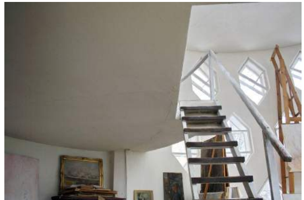
Second floor. Studio. Cracks in the finishing layers of the ceiling under the mezzanine. The stairs to the mezzanine don't have enough posts (insufficient rigidity of the handrail) and have severe wear of the treads
