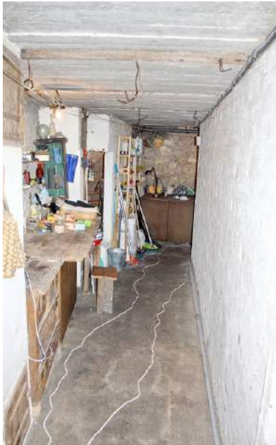
Basement, general view from east to west. Cable hooks made from reinforcing bars are visible under the ceiling. There are cracks in the floor.
