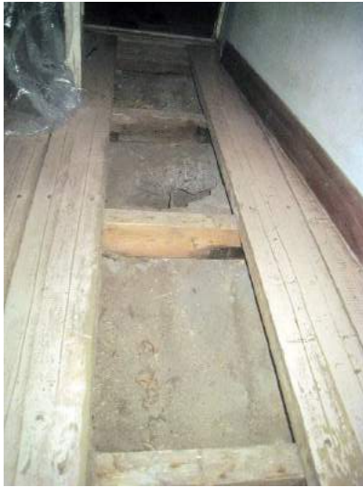
Place of the opening of the inclined reinforced concrete screed is seen between the battens.
