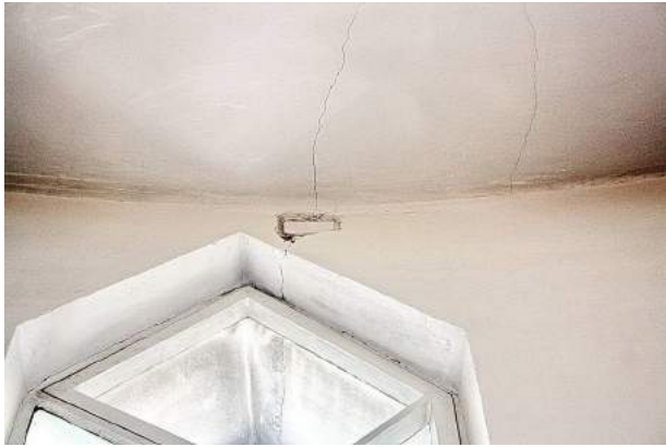
Through-wall diagonal crack under the upper window of the studio. Northwest wall
