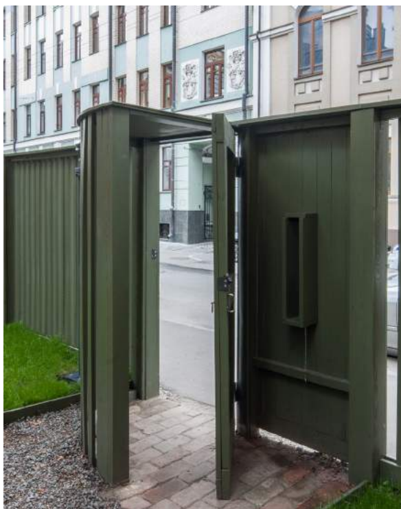
View to the House and the street fence from Krivoarbatsky Lane. Photo D. Esakov. 2016
