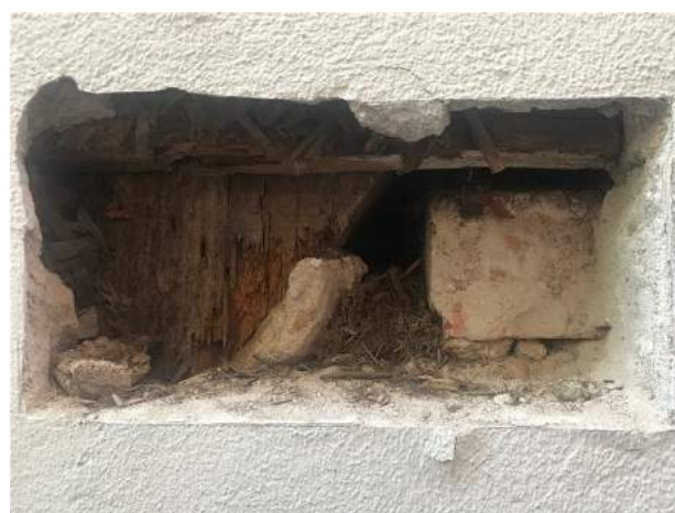
Rotten wooden shield covering hexagonal aperture in the outer brick wall. West façade of the small cylinder.
