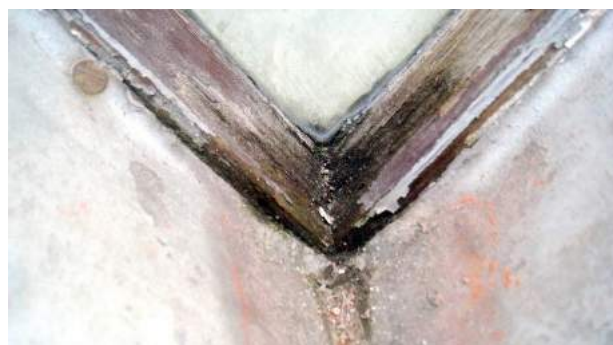
Bottom of the studio window (top row). Destruction of the paint layer, the wood is damaged by surface rot.
