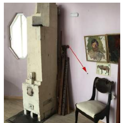
Exit point of the emergency water supply near the stove in the wall of the living-room. 1st floor
