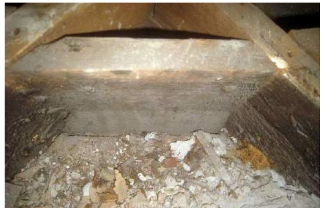
Thin rim joist is broken, probably because of the intermediate floor shift relative to the base.
