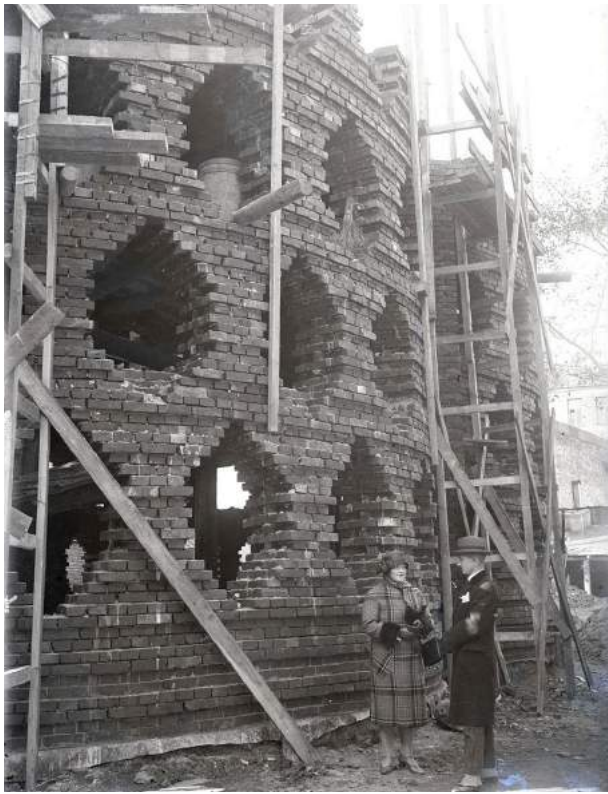
K. Melnikov and his wife Anna at the house during construction. View from the southeast. 1927
