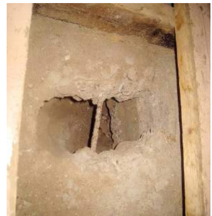
Opening of the inclined screed. The screed adjoins the reinforced concrete foundation of the partition, which partially extends on the brick wall of the basement, and at the same time is based on a sand pad.
