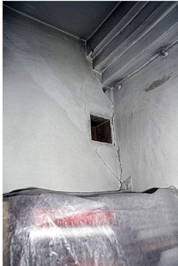
Cracks in the partition and where the partition meets the exterior wall
