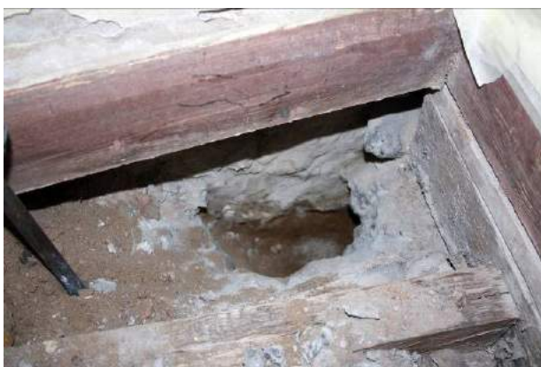
Inclined screed under the bathroom floor. The battens rest on the brick and mortar projections through the waterproofing pads. There are battens affected by rot.
