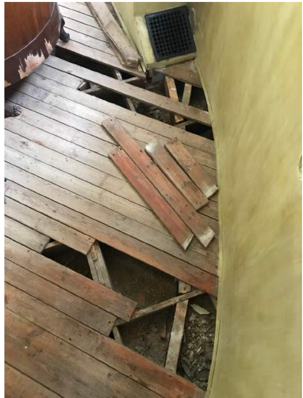
Opening of the floor. Bedroom. 1st floor
