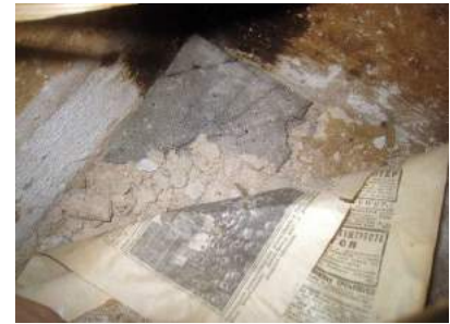
Opening of the filling. Tar paper layer on sheathing, mortar, two layers of newspapers with sand filling
