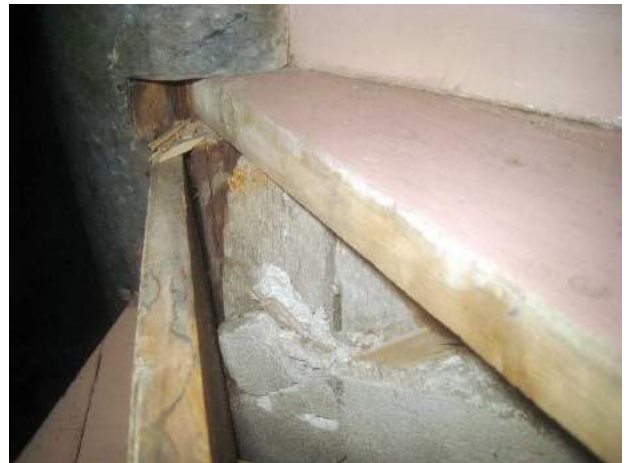
Central pillar supports the tread and the riser – leveling strips are left on the riser. The pillar has shrinkage cracks. A partition under the right side
