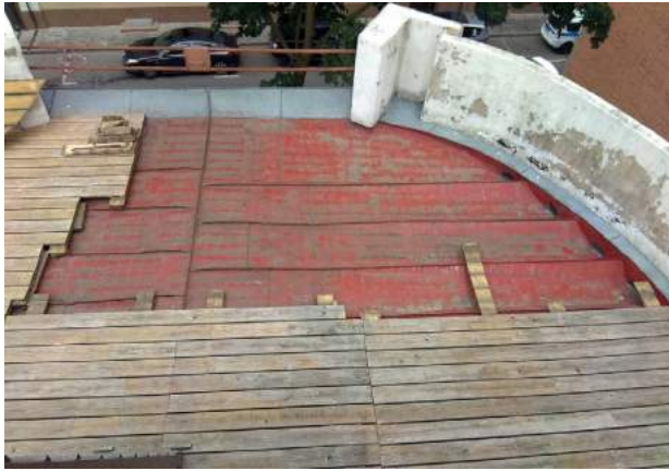
Roof of the small cylinder. Dirtiness of the roofing. The decking does not correspond to the author's design and the restoration project of the 1990s. Damage to the paint layers of the parapet.
