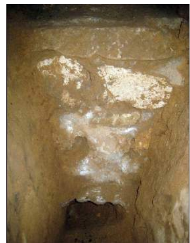
Pit 2. Lower footing
