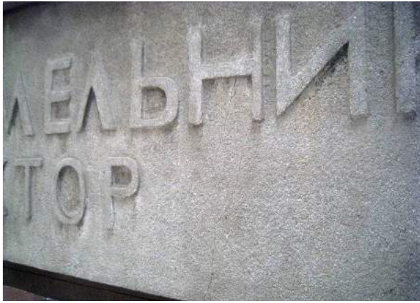
Crack in the façade inscription
