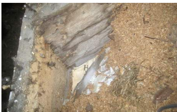
Attic floor filling. The original element is seen above – a rim joist with traces of moisture and more soft surface of wood.
