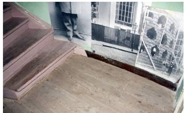
Physical deterioration of the stairs, there is a crack where the string meets the wall. Dirtying and loss of plaster layer
