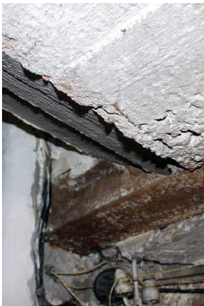
The eastmost beam of the intermediate floor rests on the wall. The beam corrosion, porous surface of concrete and corrosion of reinforcement.
