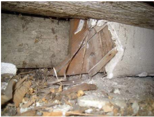
View of the lower part of the truss. Its bottom chord, diagonal sheathing boards and plaster over lath are visible
