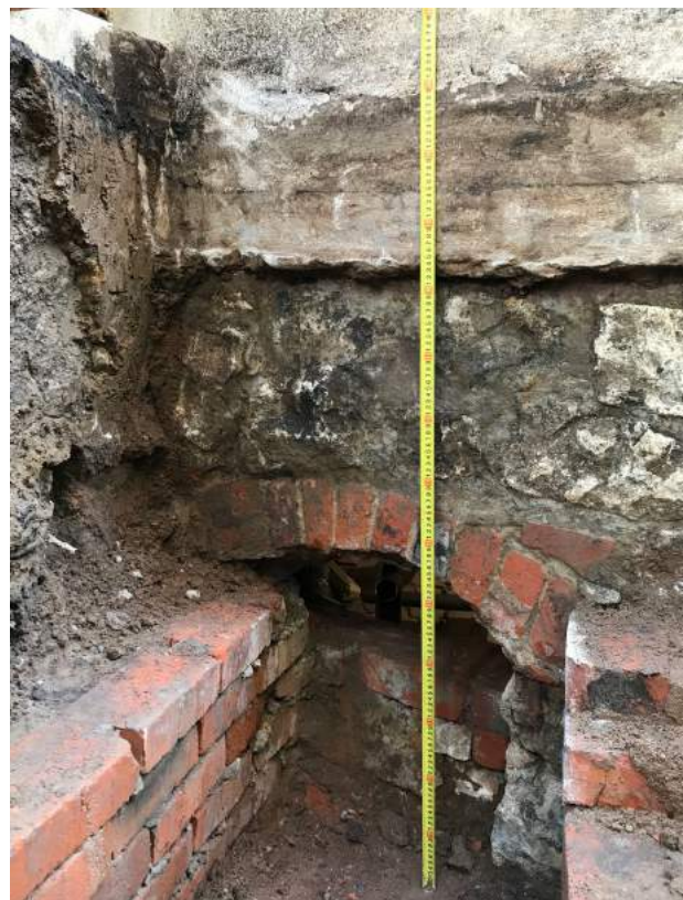
West facade. Foundations at the central heating entry point (former coal storage). 2017
