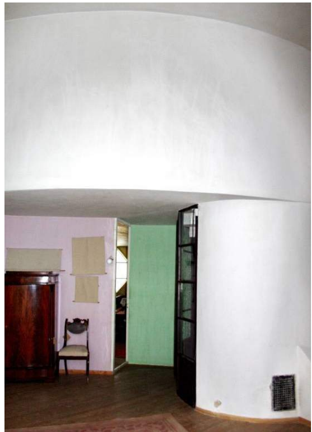
Living room on the first floor, view to the staircase. Loss of plaster on the staircase enclosure.
