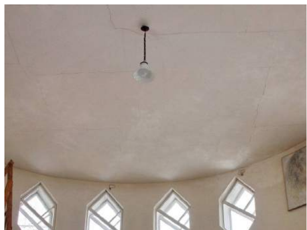
Second floor. Studio. Cracks in the plaster layer of the ceiling
