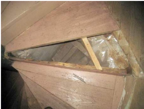
General view. A reinforcing board is seen near the center of the tread, running from the partition under the stairs to the riser. The insulation of the heating air duct is on the
