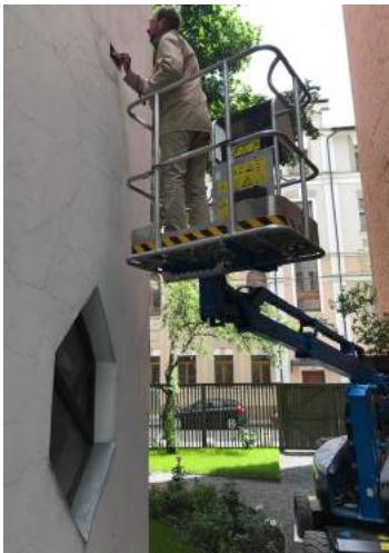
Checking the opening on the west façade
