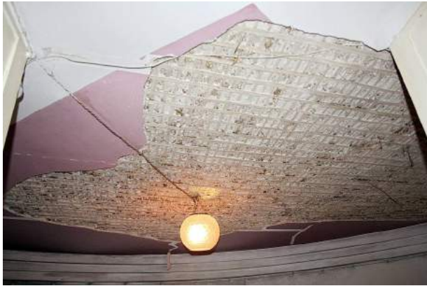
Falling away of the plaster layer from the ceiling, cracks in the rest parts
