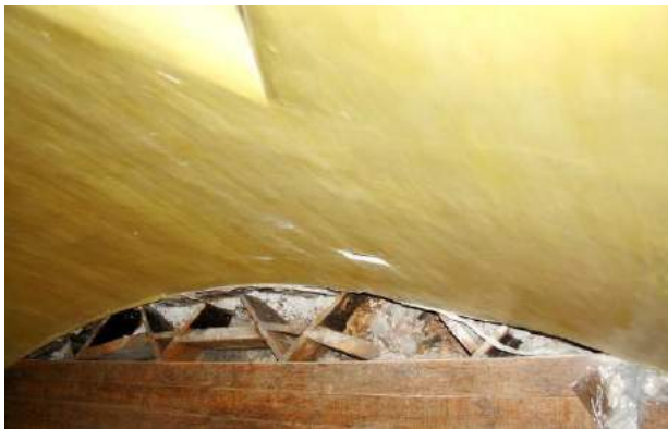
General view. Short rim joists are made of thinner boards. Rim joists are above the inner brick cornice of the ground floor wall.
