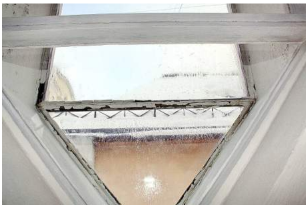
Condensation in the gap between the frames in the studio. Destruction of the finishing layers of the frames and the walls between the frames
