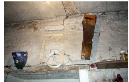
Crack in the brick wall of the basement, the wall remained from the former building. The crack width is 2.5 – 3 mm, it continues on the floor joists up to 2.5 mm wide between a joist and reinforced concrete filling
