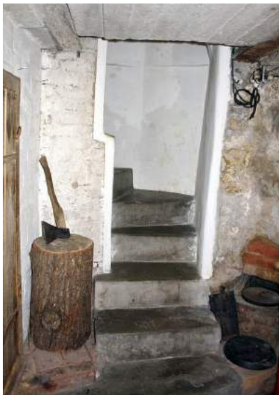
Basement, general view to the north. Cracks and detachment of the steps covering.
