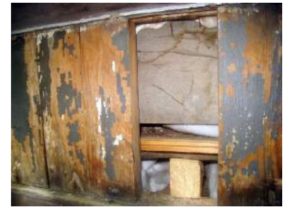
Rot on the lower frame of the large window (in some places it can be pierced with an awl), on the frame under the large window. Surface rot on the wooden filling of the frame under the large window.
