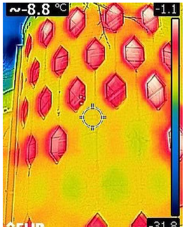
Thermal image of the northeast façade
