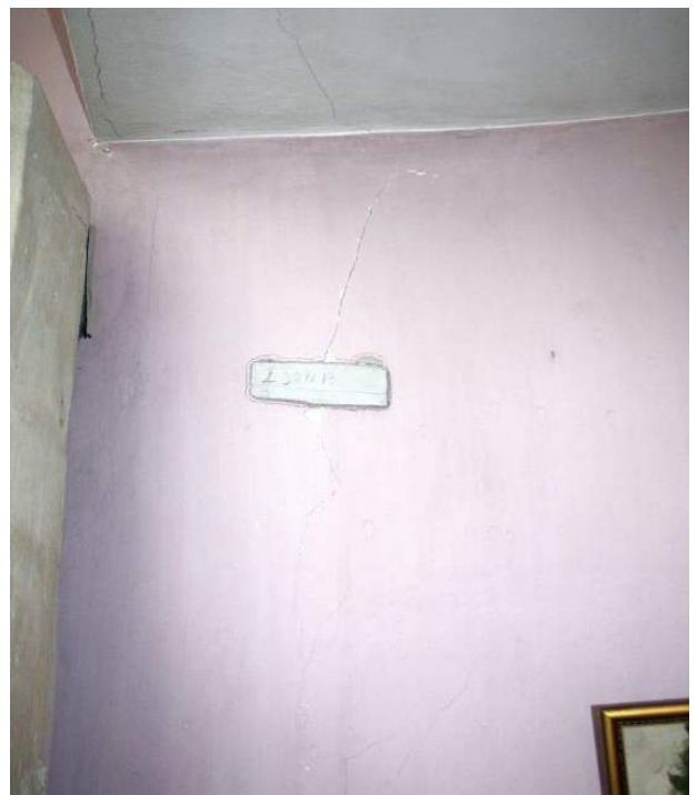
Living room on the first floor. The crack at the junction of the wooden joist and the brick wall. Cracks in the ceiling under the projection of the large cylinder
