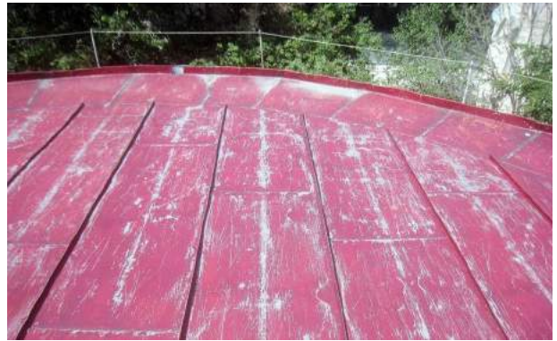
Roof of the large cylinder. Traces of water stagnation near the downspout. Paint damage
