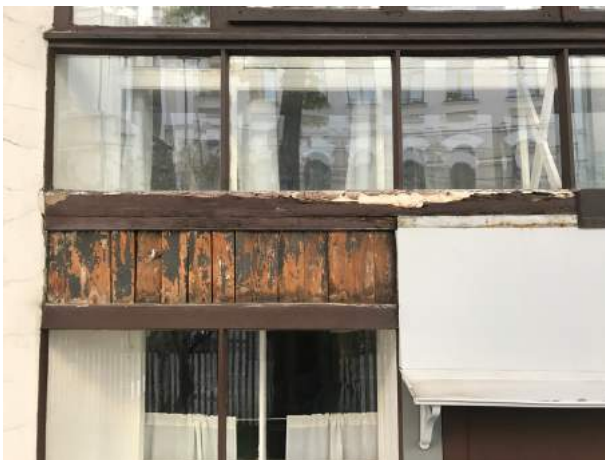
Opening of the metal sheathing. Visible old paint and wooden planks, filling the frame.
