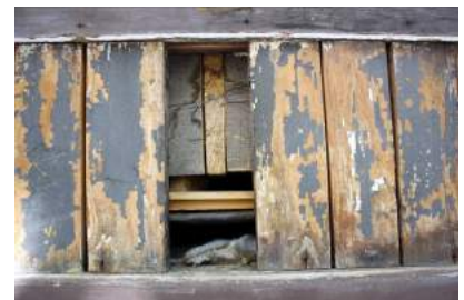
Opening of the frame filling under the large window. A visible end of a joist of the ground floor grid. Traces of the front board wetting. Traces of moistening of the filling planks and their surface rot.
