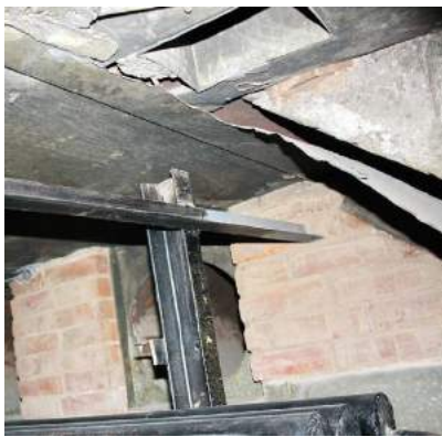
View inside the heater room. The reinforced concrete stairs are on the right side and the absence of thermal insulation of the stairs and ceiling (tinplate sheets) is clearly visible
