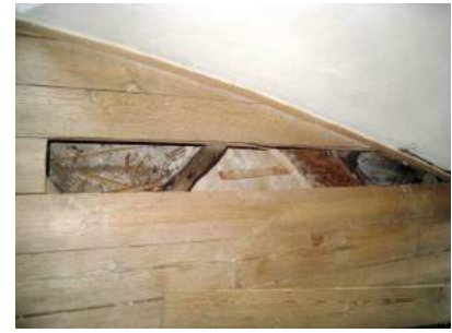
General view of the opening
