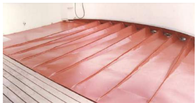
Sloped metal roof sheeting. Small cylinder
