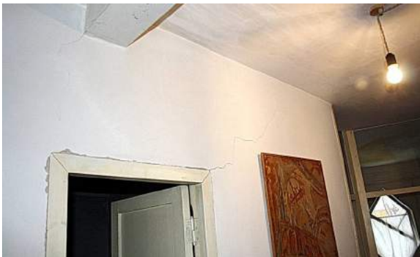
Settlement cracks in the partitions of the corridor of the large cylinder
