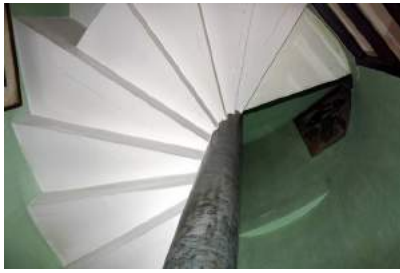
Main staircase between the first and second floors. Cracks in the plaster layers of the stairs and its cylindrical partition.
