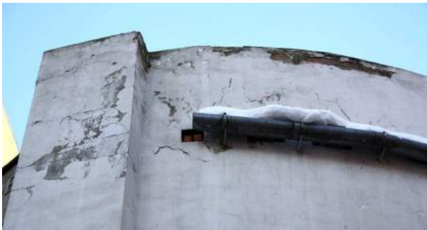
Damage to the masonry of the terrace walls owing to defrosting, loss of the plaster layer
