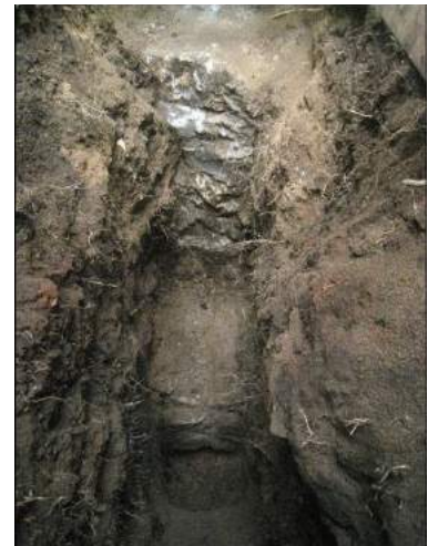
Pit 1. Lower footing. A chisel points out depth of the washed out mortar
