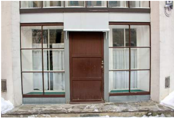
Cracks in the porch. Chinks and paint damage, warp of the entrance door boards
