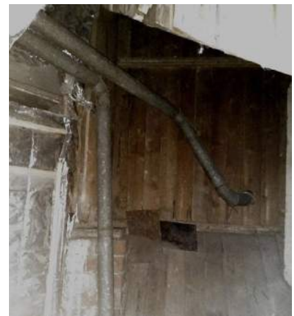
Pipes of the 'air phone'. Closet under the staircase. Ground floor
