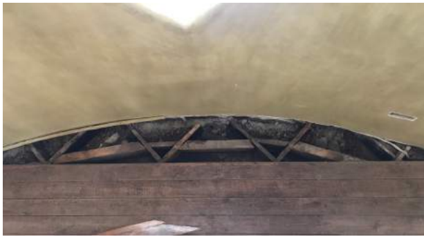
Inter-floor structures damaged by rot. Bedroom, 1st floor
