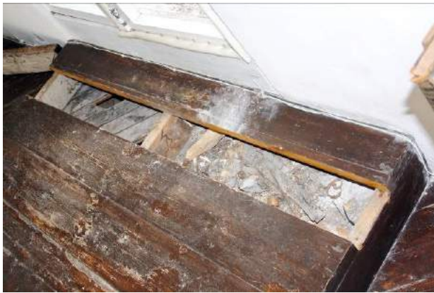
General view. Construction debris in the filling under the floor
