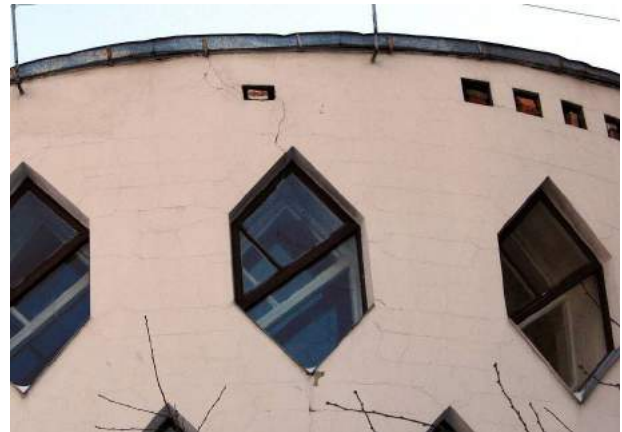
Through-wall diagonal crack 0.3 mm wide. Northwest façade.
