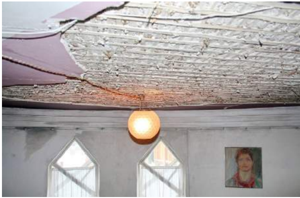
Dressing room on the ground level. Cracks in the ceiling, falling of the plaster layer. Parts of the remained plaster hang loose on the lath, bast fiber fabric and burlap, which cover the lower sheathing of the intermediate floor, and gradually crumble.
