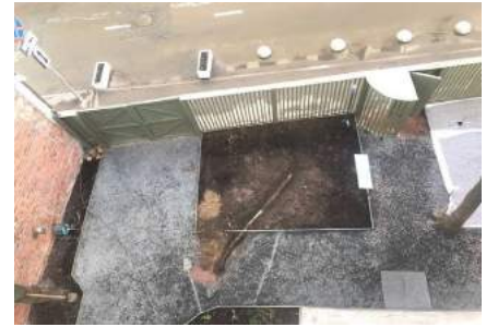
Excavated underground part of the 'air phone' going from the fence to the house
