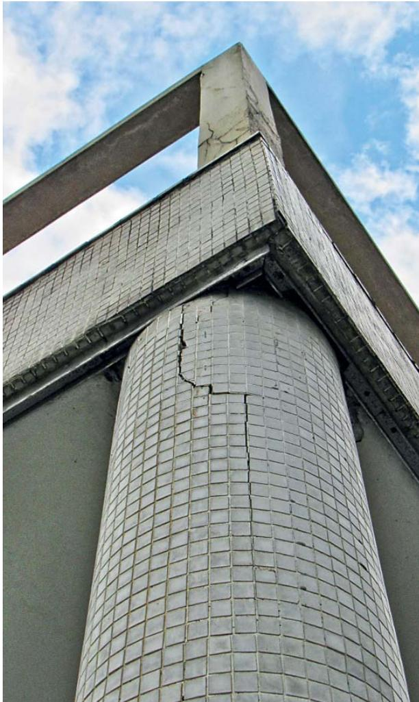
29 – Exemplo de fissura na coluna – An example of a crack in the pillar
