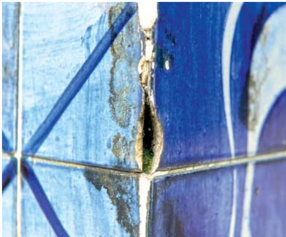
39 – Fissura na parte central do painel – Crack in the central part of the mural
