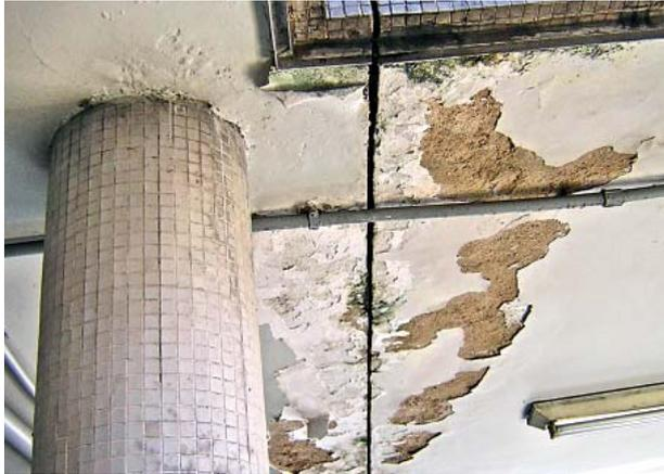
27 – Infiltração das lajes – Leaking roof
