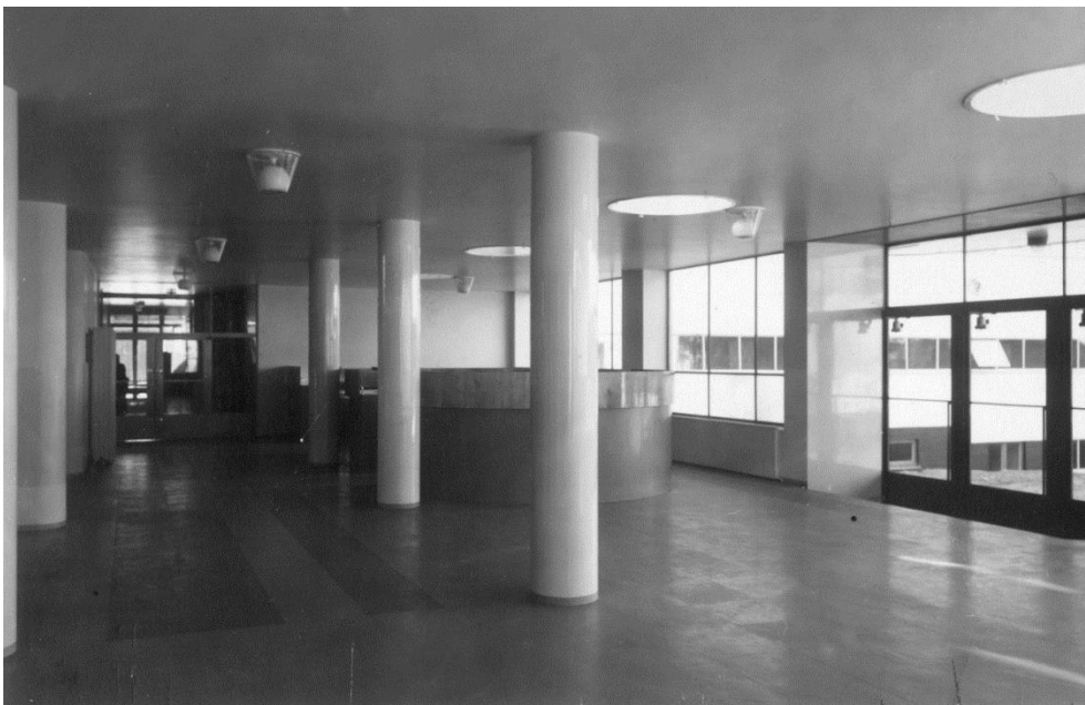
Main hall with the original flooring and front desk. No draught lobby was built at this stage. Below is the current status of the Main lobby. Notice how the light does not pass through the Ground floor ward through the ward doors due to some change, leaving the back part of the lobby dark. AAM Sign. 50-005-308.
