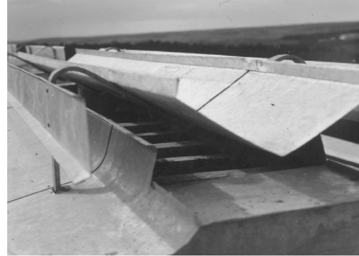
The covers of the A-wing ducts differed from the original design (AAM 50-003-142).
