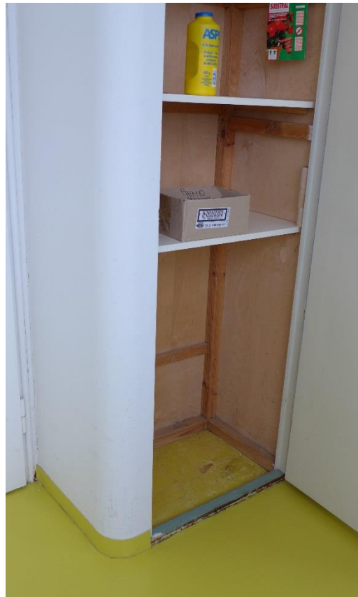
The original fragment of yellow flooring in comparison to the renewed flooring surrounding the cupboard.
