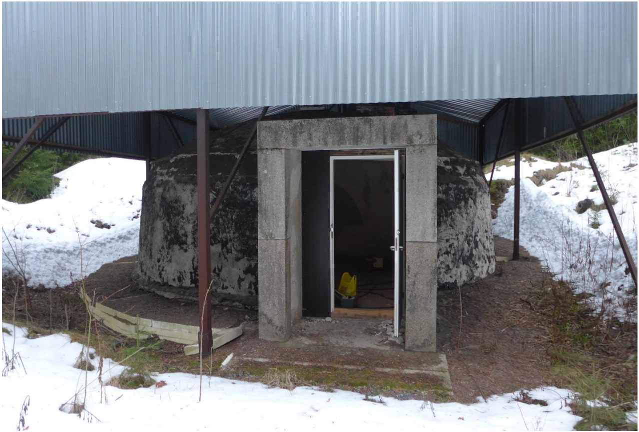
The state of Rose cellar today. The masses of soil covering the dome have been removed. The original moisture insulation, the black tar-like coating has been scraped down to ensure further drying of the structure. The cellar has been covered with a temporary shelter to protect it from rain and subzero temperatures during 2005. The original door has been removed, stored and replaced by a temporary door. An underground drain has been installed around the dome to gather most of the water from the ground.
