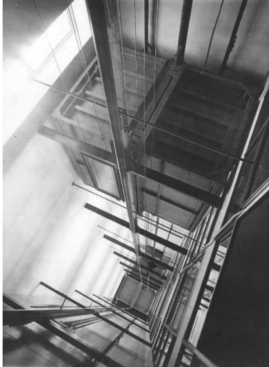
The main elevators were capable of transporting 15 persons at a time over 8 stories. (AAM 50-003-344; AAM 50-003-341 Gustaf Welin).
