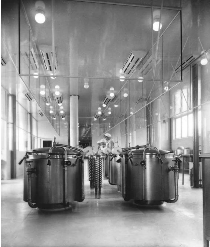
The original kitchen with air outlets and glazed steam collectors (AAM 50-003-402 Gustaf Welin 1933).
