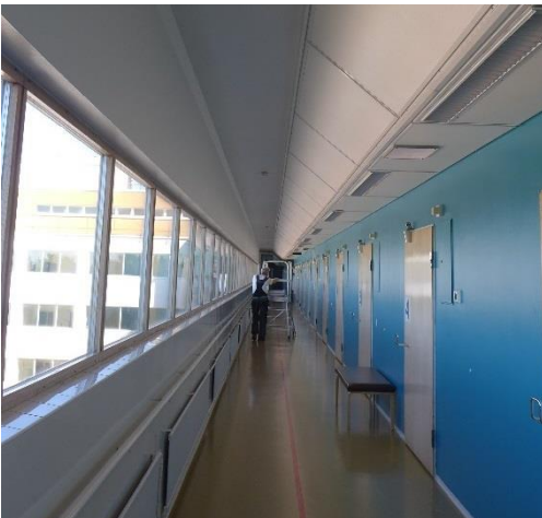
One of the wards (probably sixth according to the view from window). The wall with doors was painted in rich a tone and the outer wall in neutral color of off white. Below is a view today from the sixth floor ward to the opposite direction. Notice the built in structure in the ceiling for the purpose of hiding ventilation systems and electricity cords, dating to the 1970's. AAM. Sign. 50-003-328
