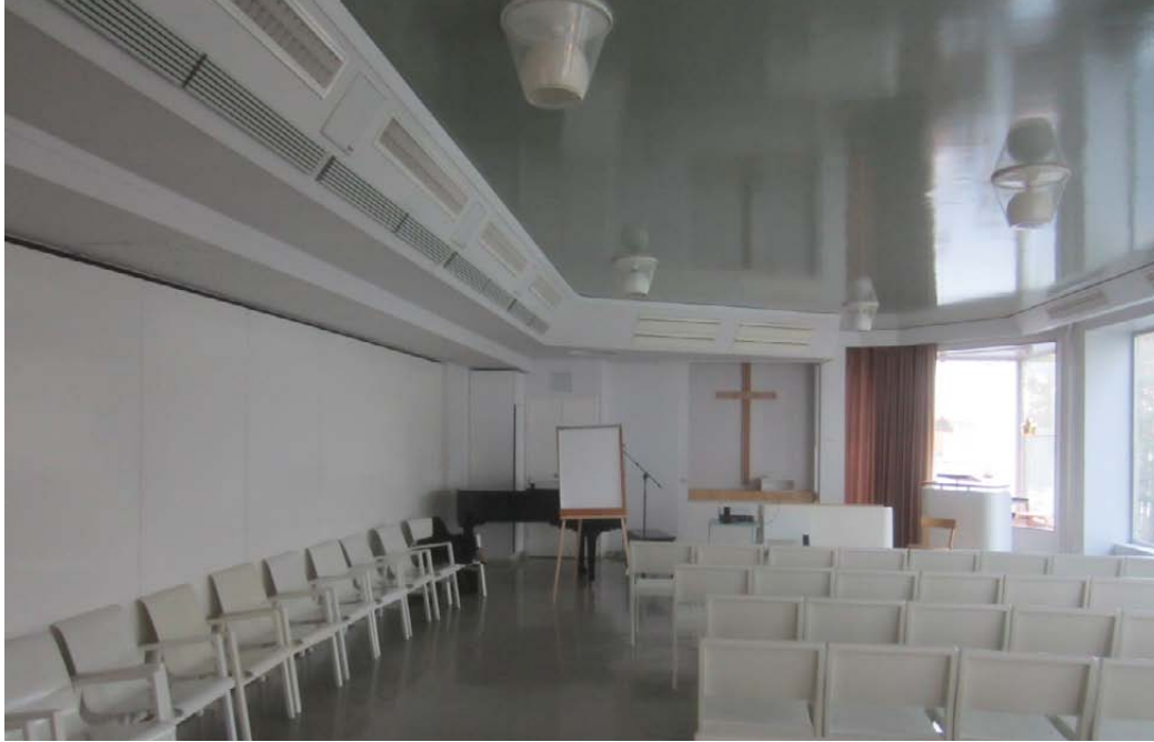
The partially suspended ceilings were installed in the day room in the 1980s (AAM Malmberg).
