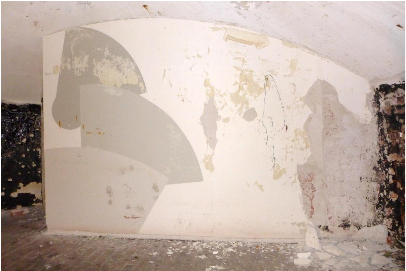
The current state of the Rose Cellar mural. August 2015. The presumed original redbrick floor is now revealed after the peeling of concrete flooring. Black tar-like watertight coating has also been stripped partly to enhance the drying process of the water damaged wall structures.
