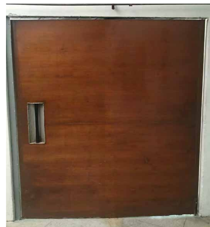
INSIDE FACE OF DOOR
