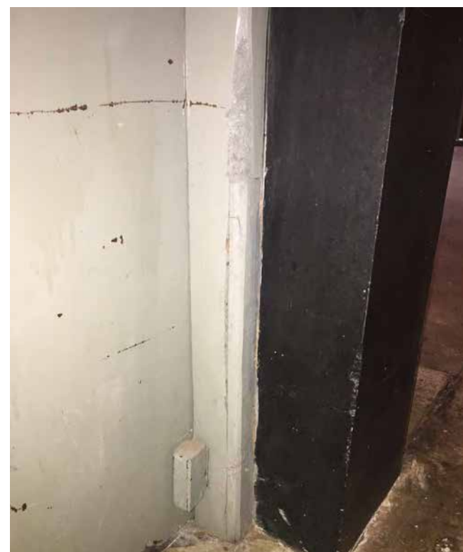
WOOD PIECE ADDED TO REPAIR
