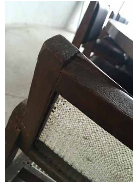
BUCKLING CAUSED DUE TO BREAKAGE
