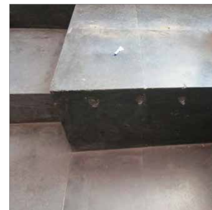
PREVIOUS INTERVENTION IN AUDITORIUM STEPS
