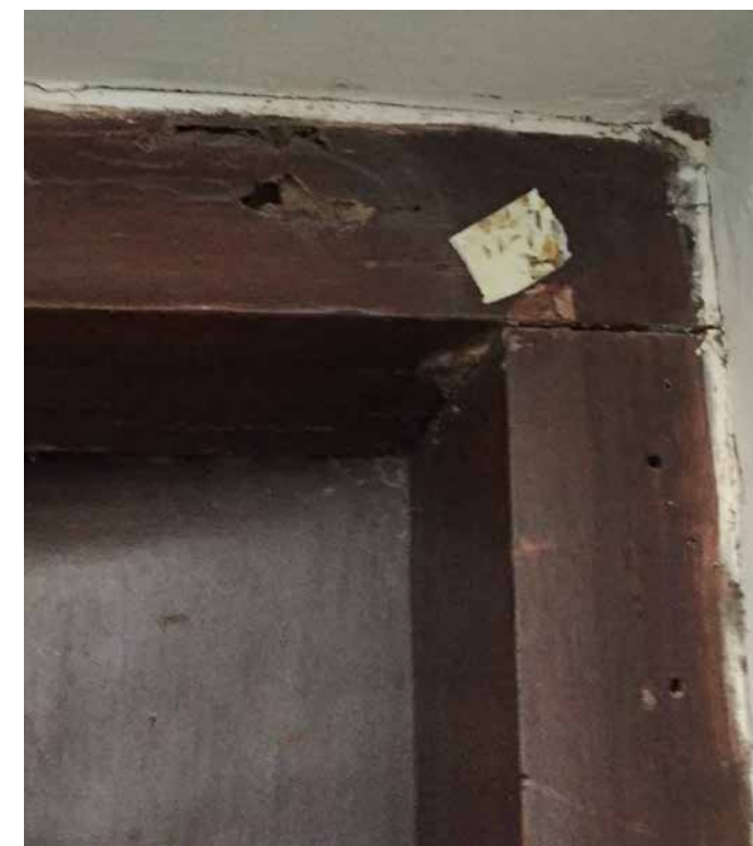
DAMAGED PORTION DUE TO TERMITE
