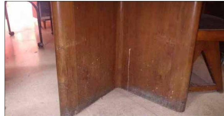
VENEER DISINTEGRATING FROM BOTTOM EDGE
