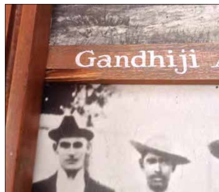
LOSS OF WOOD IN DISPLAY PANEL-1
