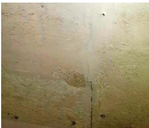
Joints flushed with Epoxy resin
