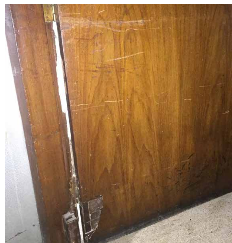
MATERIAL LOSS AND SURFACE ABRASION
