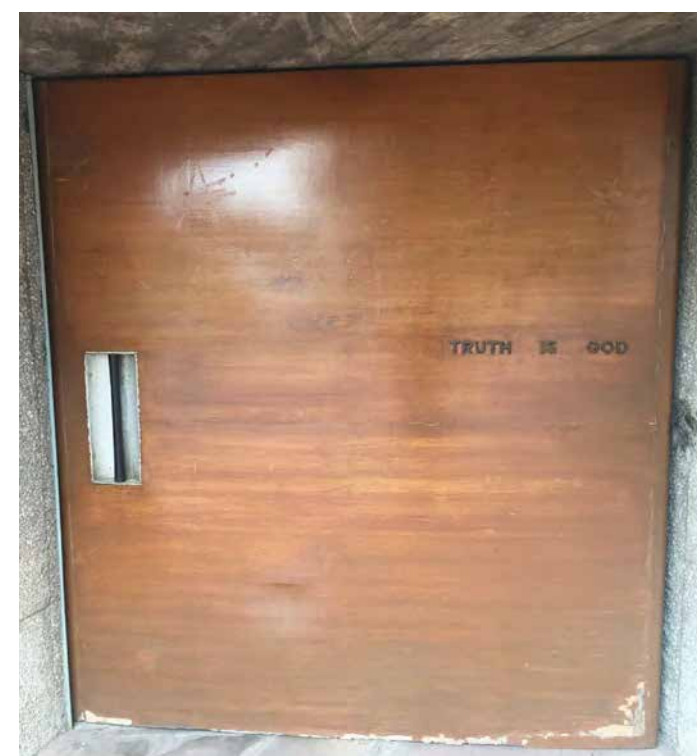
OUTSIDE FACE OF DOOR
