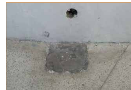
INTERVENTION IN OFF WHITE TERRAZZO FLOOR COMMITTEE ROOM (GF5)
