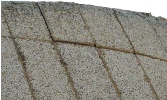
Figure 1.3 Dislodged Panel
