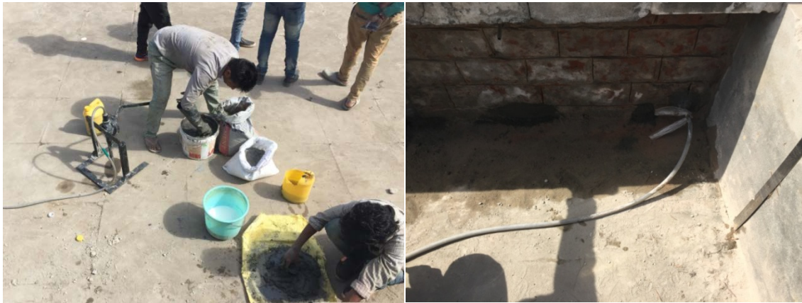
Figure 86 Mixing of compounds with cement and Pipe fixed onto the nipple for pressure grouting
