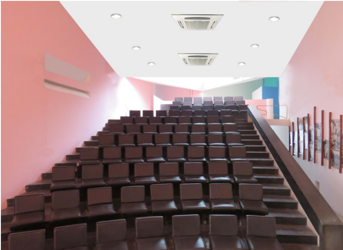
Figure 122 View of Option 1 : false ceiling A.C. units in the Auditorium
