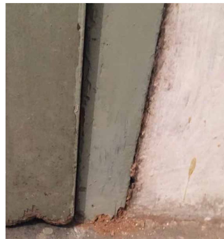
TERMITE INSIDE THE DOOR FRAME
