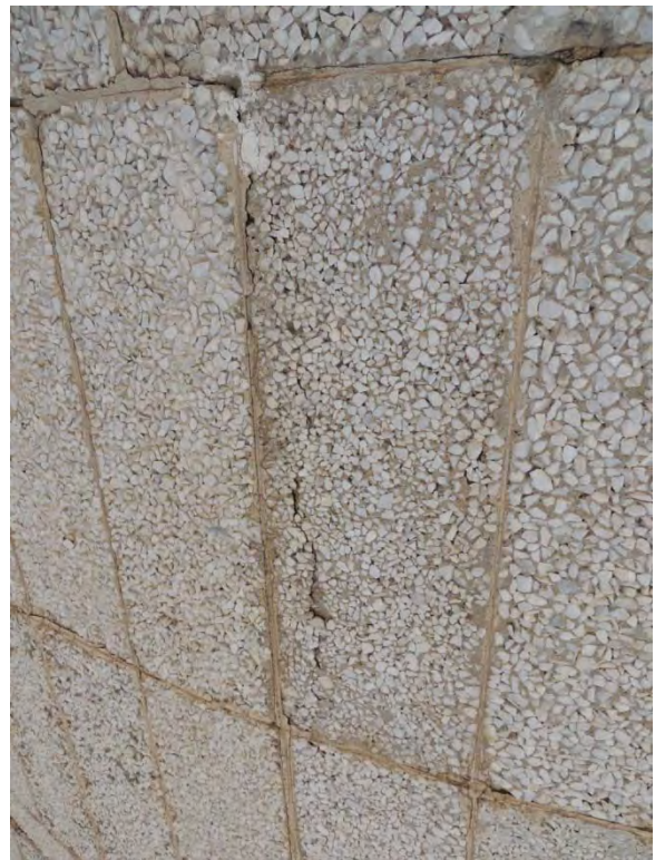
Figure 1.6 Cracked Panel
