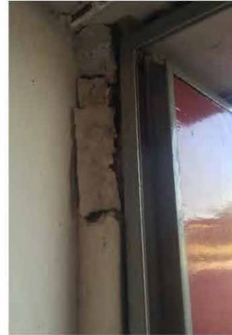
LOSS OF CONCRETE
