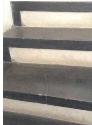
CRACKS IN LIBRARY STAIRCASE
