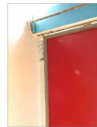
MATERIAL LOSS NEAR THE DOOR
