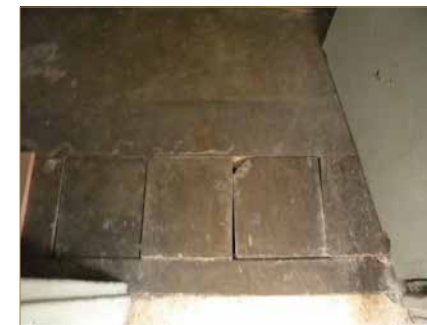
BROKEN FLOOR IN STORE ROOM (GF8)
