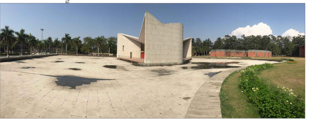
WATER STAGNATION IN THE POOL
