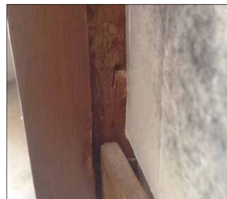
LOSS OF WOOD IN DISPLAY PANEL-1
