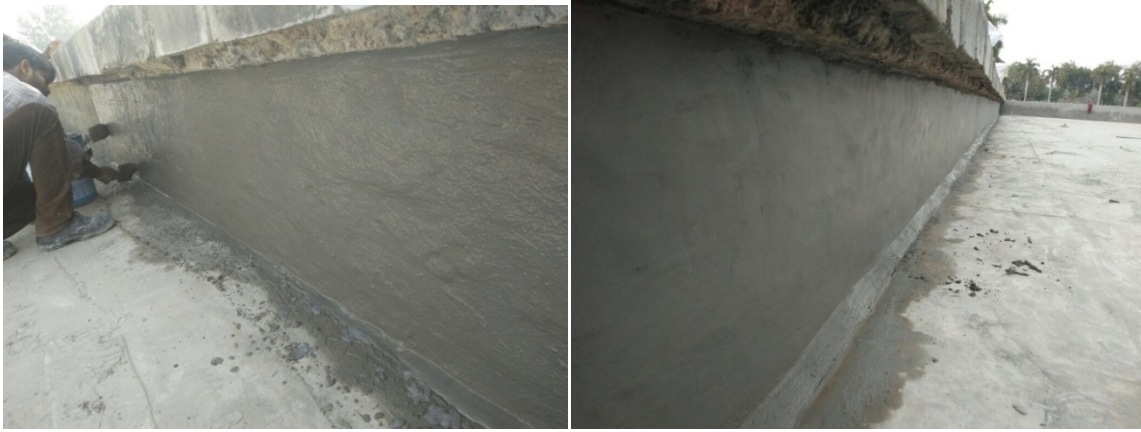
Figure 89 Coat of High Bond 40 mix with cement & water and Final plastering with Bond FRS
