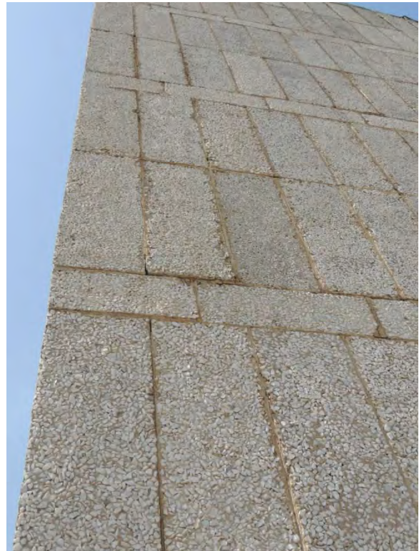
Figure 1.2 Dislodged Panel
