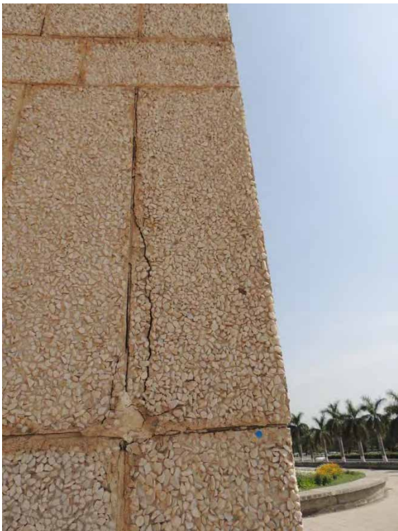
Figure 1.5 Cracked Panel
