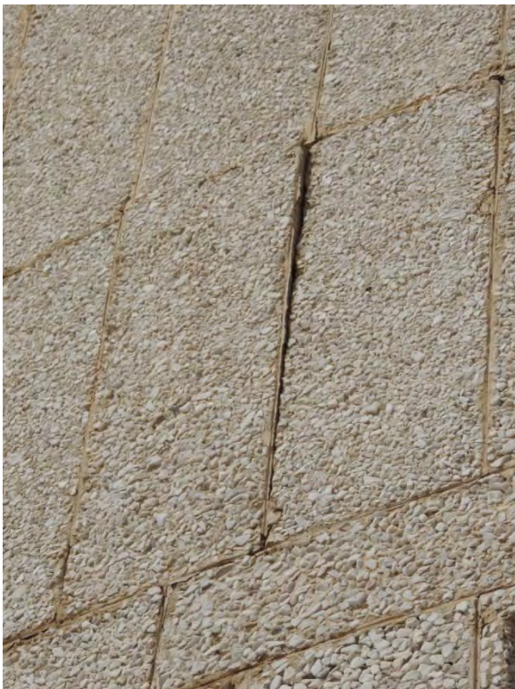
Figure 1.1 Dislodged Panel
