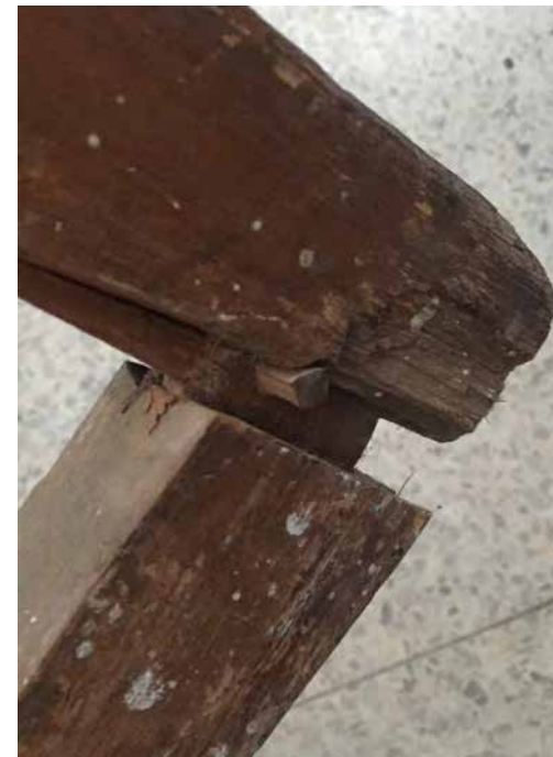
JOINT OPENING & MATERIAL LOSS ON RIGHT LEG
