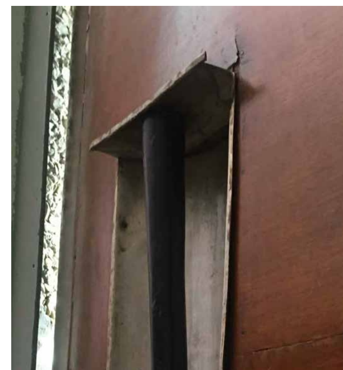
LOOSE HANDLE ON THE INNER FACE
