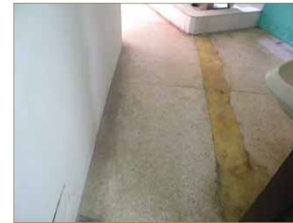
PREVIOUS INTERVENTIONS IN THE WHITE TERRAZZO FLOORS NEAR TOILETS (GF 9a)
