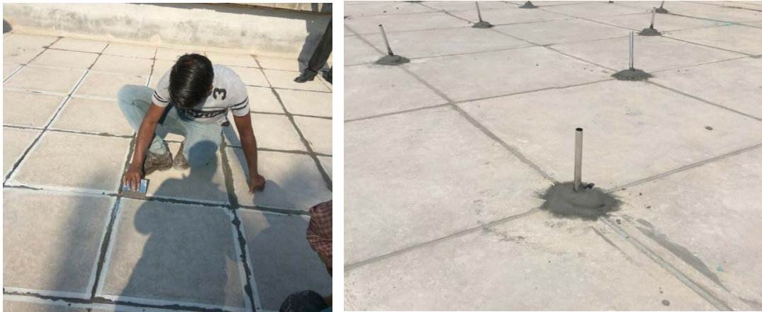
Figure 93 Sealing of joints with High Bond 40 mix and Inserting & fixing nipples 2" deep into the holes.
