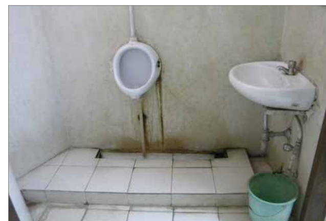
PREVIOUS INTERVENTION ON TOILET FIXTURES
