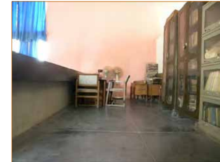
STAINS ON BLACK TERRAZZO FLOOR IN MEZZ. LIBRARY (MF2)
