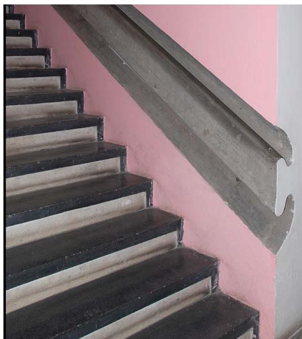
Figure 74 Detail of original cove lighting incorporated with staircase railing
