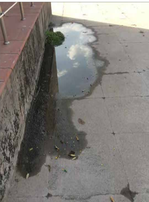
WATER STAGNATION IN THE POOL & ALGAE GROWTH ON THE BASE OF THE BUILDING
