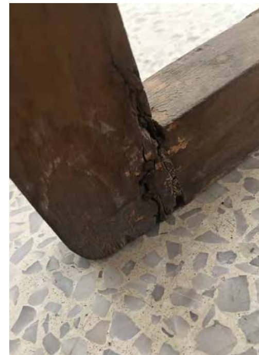
MAJOR CRACKS IN REAR LEFT LEG
