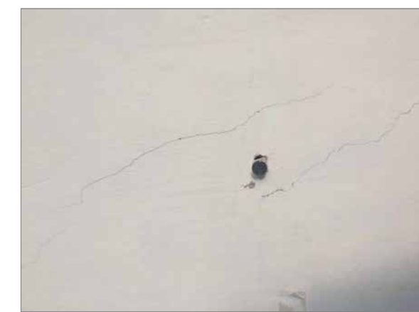
CRACKS IN PLASTERED WALL
