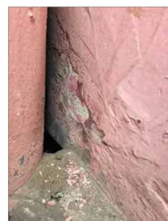
PLASTER LOSS ON WALL
