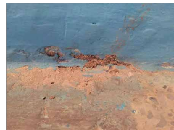
TERMITE ON THE WALL
