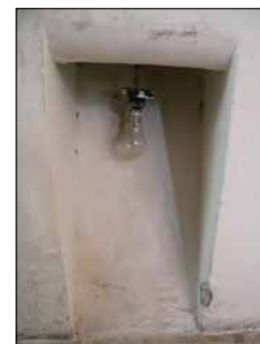
LOSS OF EDGES AND DEPOSIT
