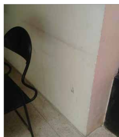
STAINS ON WALL
