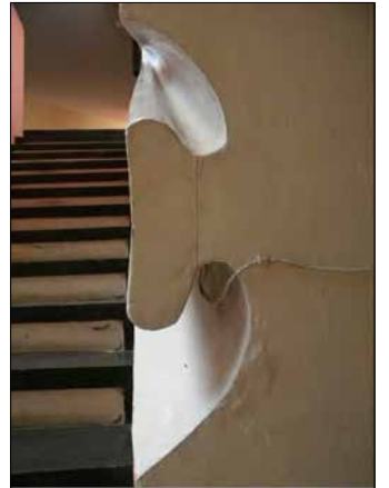
SATINS AND DEPOSIT IN THE RAILING
