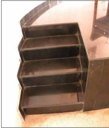
PREVIOUS REPAIR ON STAGE
