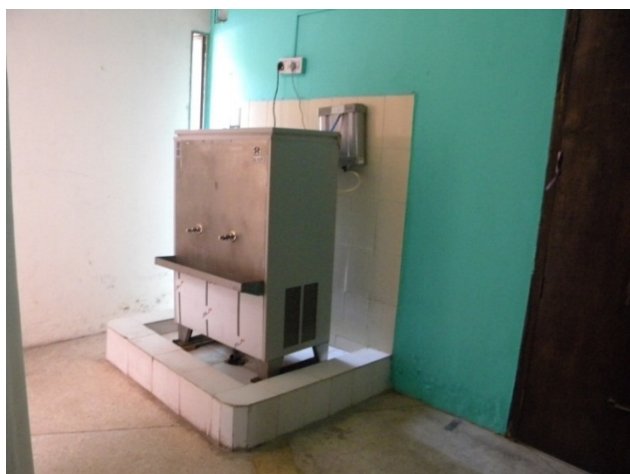
Figure 75 Water cooler at Gandhi Bhawan, which is an eyesore, needs to be replaced
