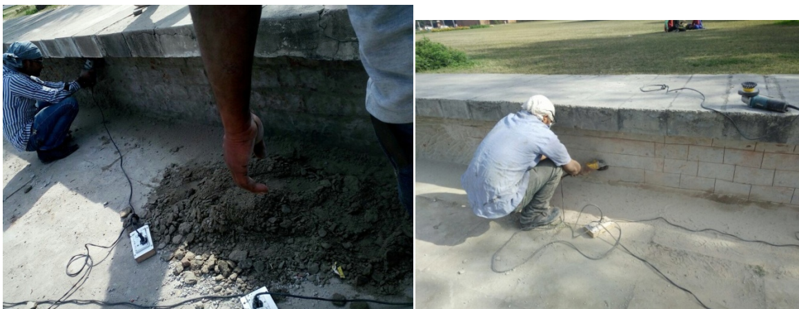
Figure 83 Removing plaster with mechanical means and Cutting construction joints with cutter
