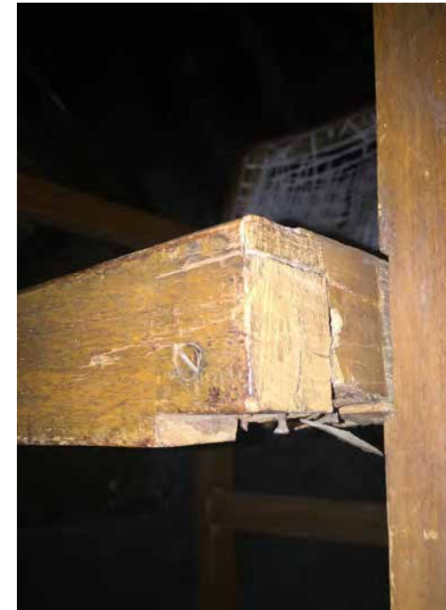
INAPPROPRIATE REPAIR WORK
