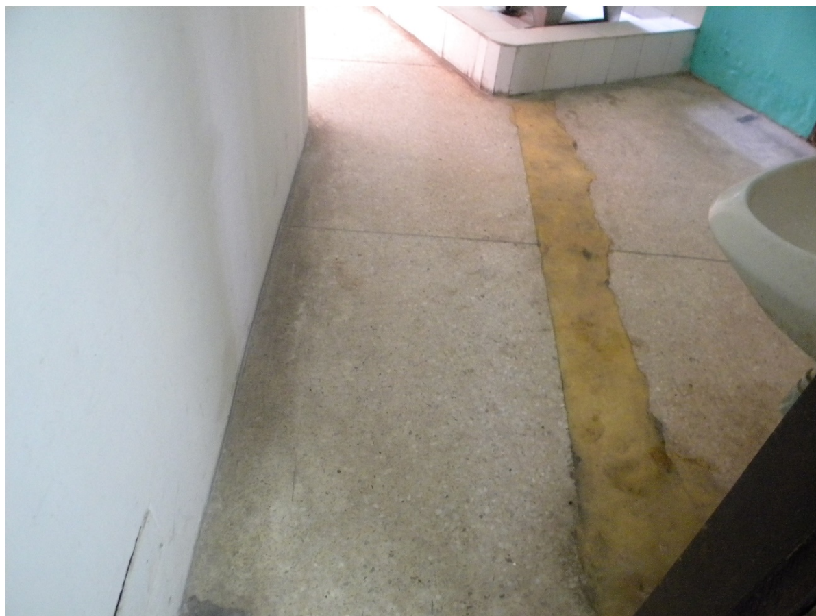
Figure 69 Patch repairs in floor outside the toilets
