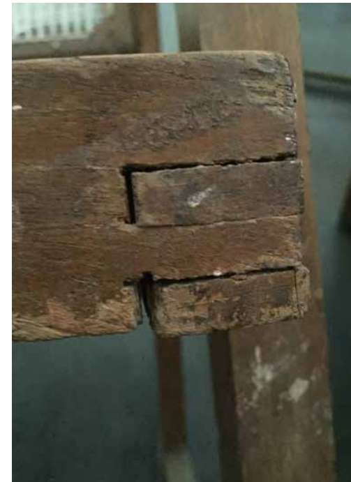
LOOSE JOINT ON FRONT SIDE
