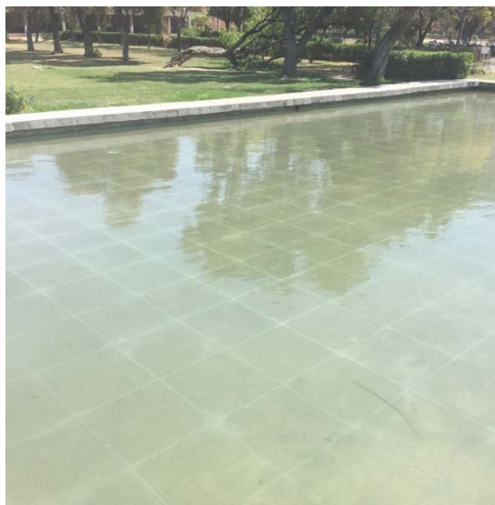
Figure 95 Cleaning of surface and Filling of water upto 20" after 2 days of treatment
