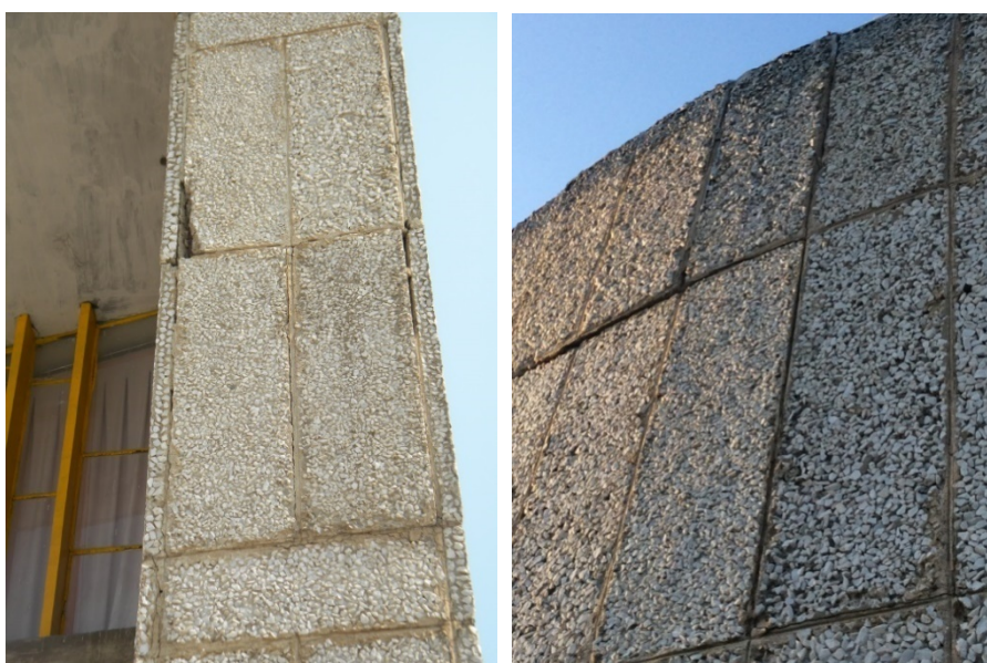
Figure 76 External panels that are showing signs of structural distress as identified by the various assessment techniques used for the Gandhi Bhawan pose a significant threat to both life and to the integrity of the panels themselves and need urgent attention
