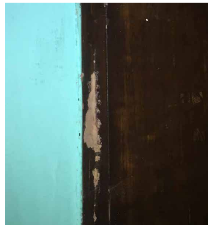
MATERIAL LOSS DUE TO TERMITE
