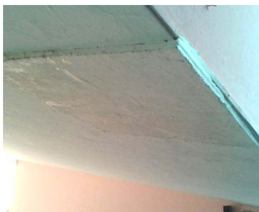
Rough edges and joints finished
