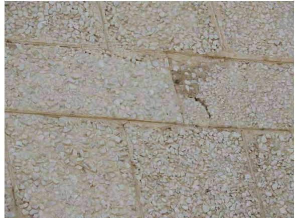
Figure 1.4 Cracked Panel
