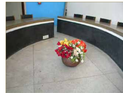
STAINS ON TERRAZZO FLOOR IN SEMINAR ROOM (GF5)
