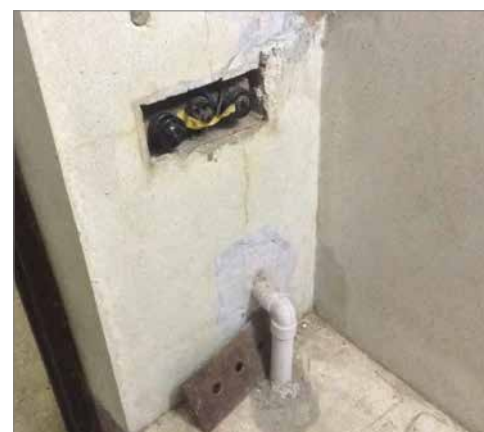
DAMAGED ELECTRICAL FIXTURES
