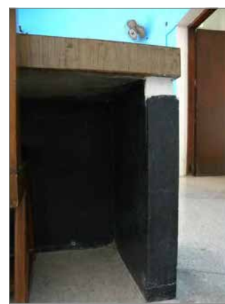
CRACK IN FIXED TABLE IN COMMITTEE ROOM
