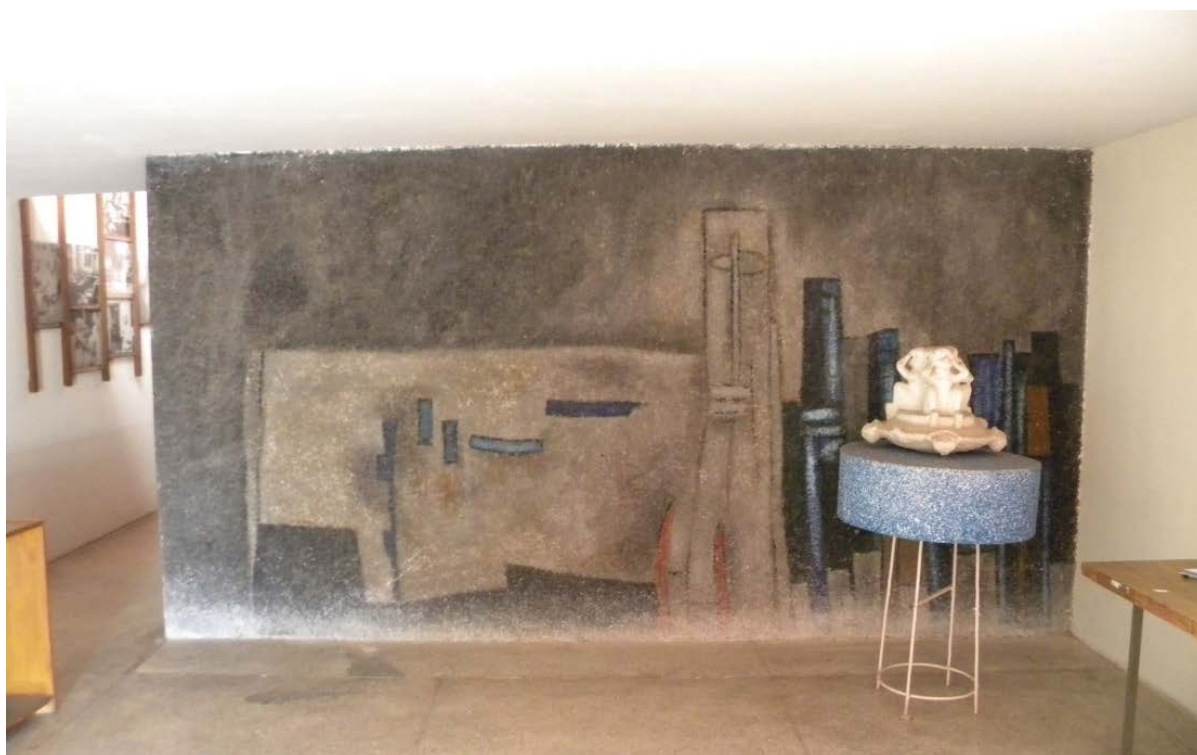
Figure 70 Mural as seen from the entrance in 2016 shows deterioration and splash of paintwork at bottom
