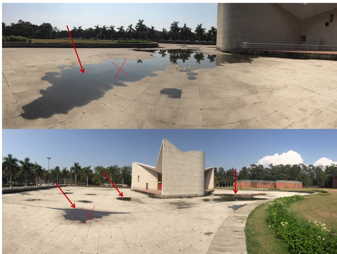
Figure 62 Standing water in empty pool
