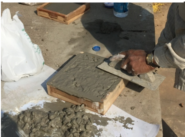
Figure 103 mixing of aggregate with mortar and filling it in mould
