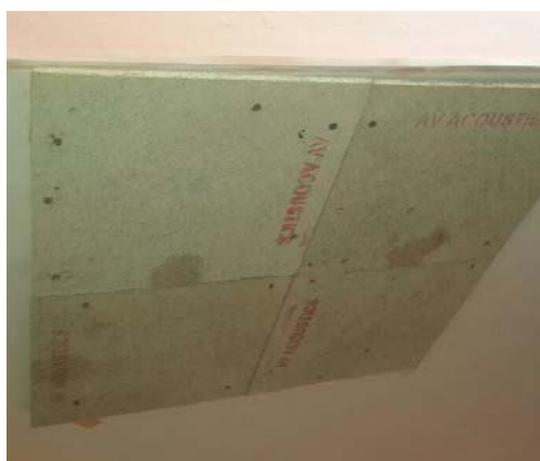
Wood composite Board fixed on top of base layer
