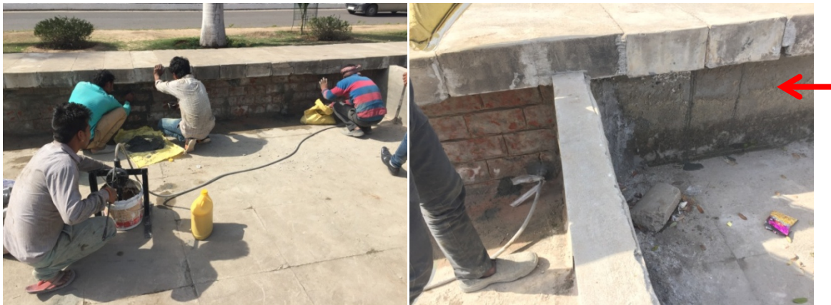
Figure 87 Pressure grouting being done with a manual pump and Grout coming out of sieves and spaces in the wall
