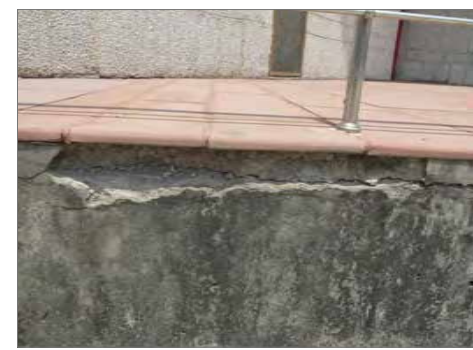
LOSS OF MATERIAL AT THE EDGE OF SIDE WALLS OF THE POOL
