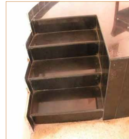
PREVIOUS INTERVENTIONS ON THE STAGE (GF 3)
