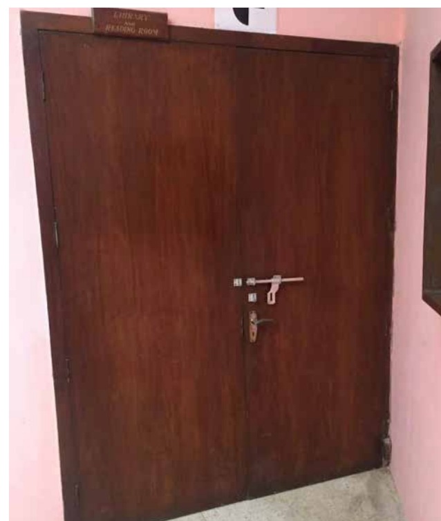
OUTSIDE FACE OF DOOR
