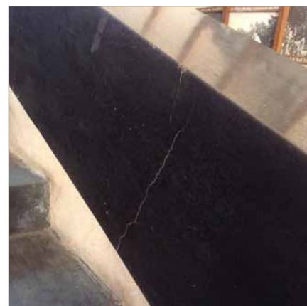
CRACK IN BLACK TERRAZZO WALL
