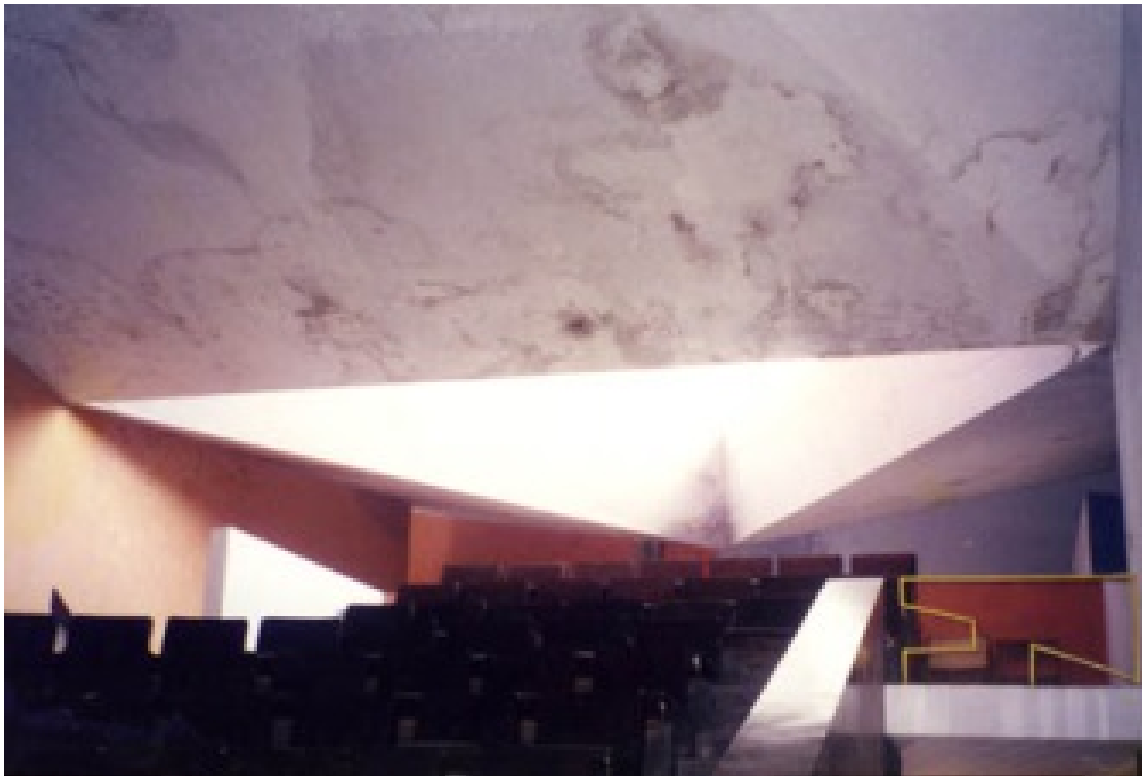
Figure 58 In 1995, extensive seepage could be seen in the ceiling (Source: Byunguh Yu, http://cnu.daejeon.kr/awa/Asia-India/ENGLISH-WFB%20Asia-India-Chandigarh-Open%20Hand%20&%20Rock%20Garden.htm )
