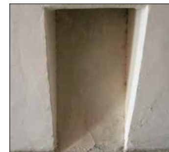
WALL COVE LIGHT
