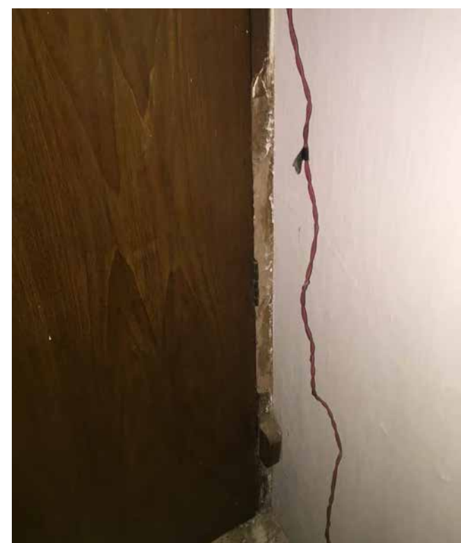
DISINTEGRATED DOOR FRAME DUE TO TERMITE
