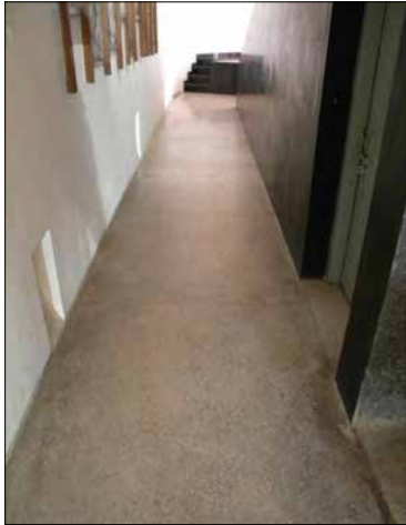
STAINS ON WHITE TERRAZZO FLOOR IN CORRIDOR
