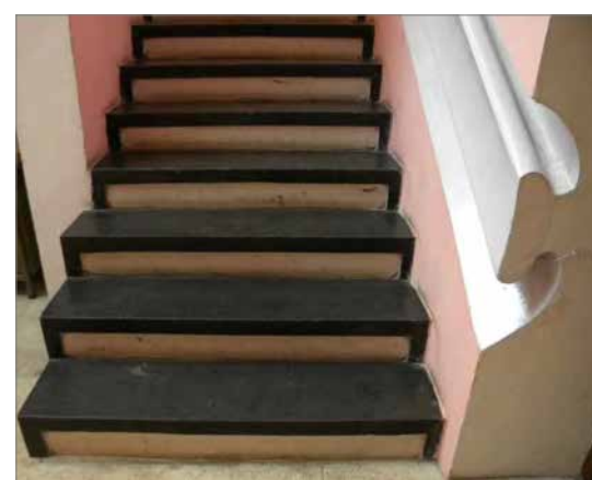
CRACK IN BLACK TERRAZZO FINISH STEPS IN LOBBY
