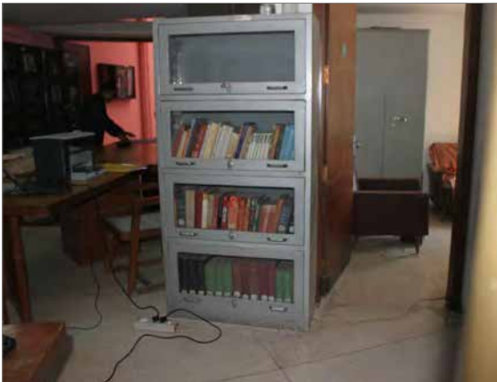
PREVIOUS INTERVENTION OF LIBRARY STACKS AND ELECTRICAL WIRING
