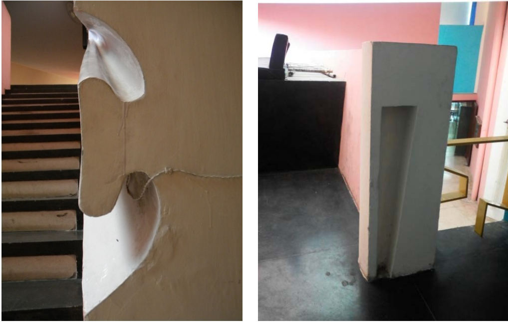
Figure 52 Details of Cove lighting in wall and Railing
