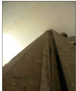
DIRT DEPOSIT WALL COVE LIGHTING IN MEZZ. LIBRARY
