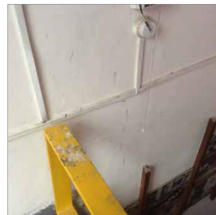
DEPOSIT ON MILD STEEL RAILING
