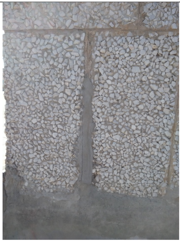
Inappropriate repairs
