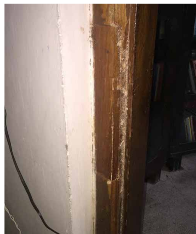
WOOD PIECE ADDED TO REPAIR
