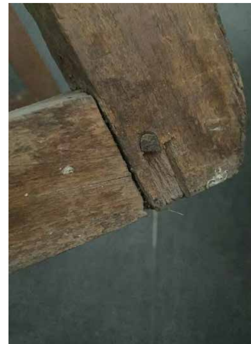
MATERIAL LOSS ON RIGHT LEG
