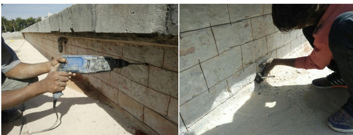
Figure 84 Drilling 12" deep holes into the wall and Inserting nipples into the holes up-to 2"
