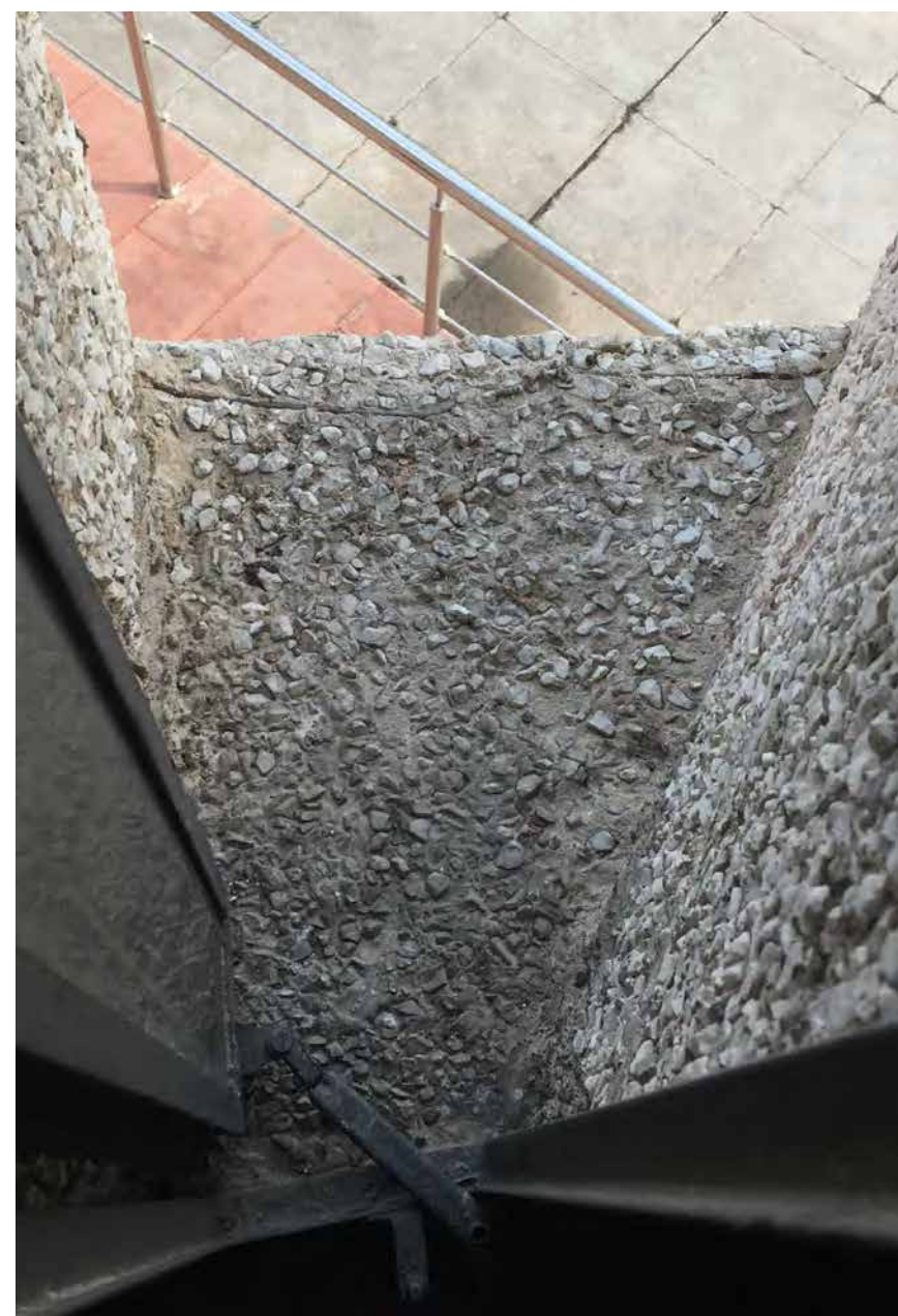
EXPOSED RE-BARS IN PANEL
