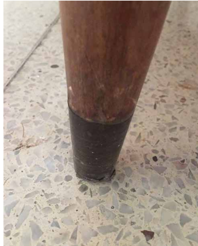
METAL CAPPING ON LEFT FRONT LEG
