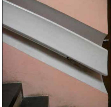
SATINS AND DEPOSIT IN THE RAILING
