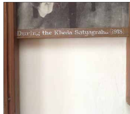
CRACKS IN DISPLAY PANEL-2
