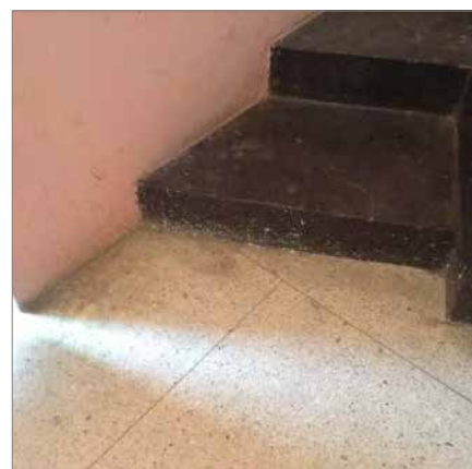
CRACK IN BLACK TERRAZZO FLOOR STEPS
