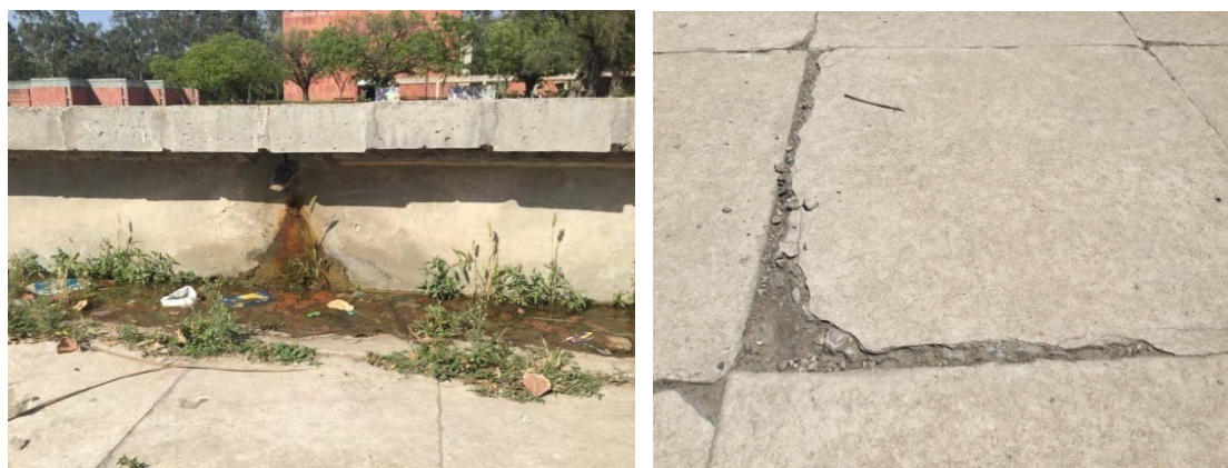
Figure 64 Vegetation growth & Deterioration in Pool base and sides
