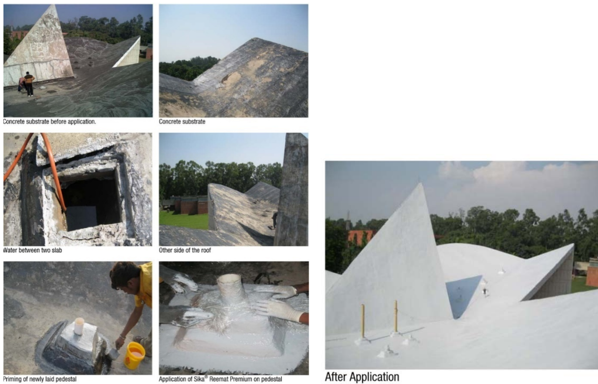
Figure 59 In 2010-2011 Sikalastic MTC Roofing were commissioned to make the roof form of the building water tight (Source: Siklastic)
