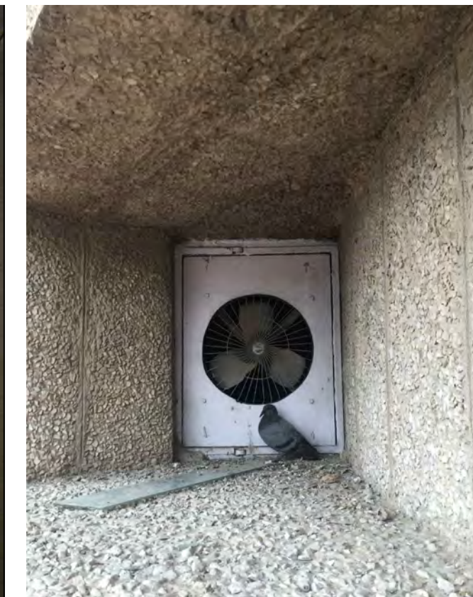
LINTEL SURFACE REPAIRED
