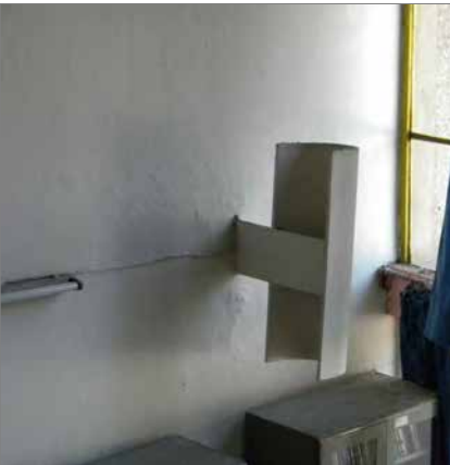
PLASTER DEFECTS ON WALL IN LIBRARY
