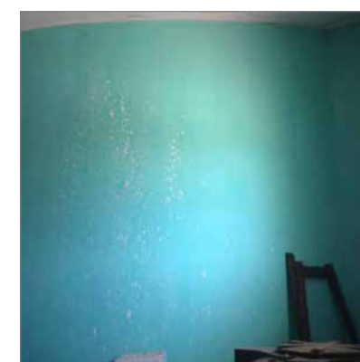
DEPOSIT ON THE WALL
