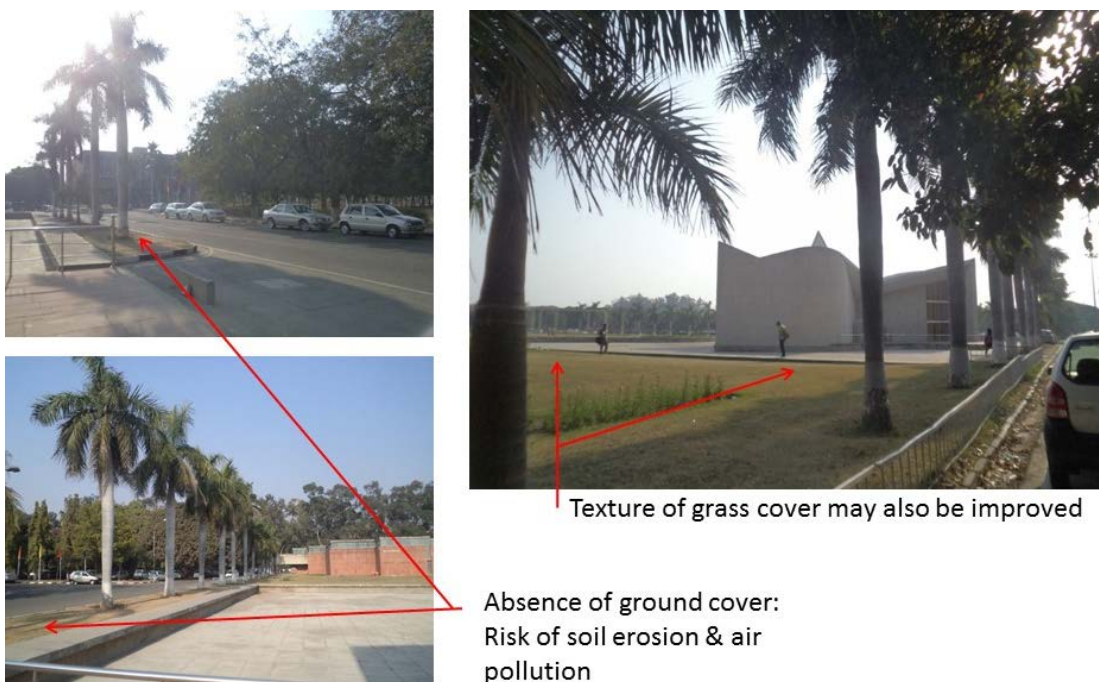
Figure 63 Surrounding vegetation assessment
