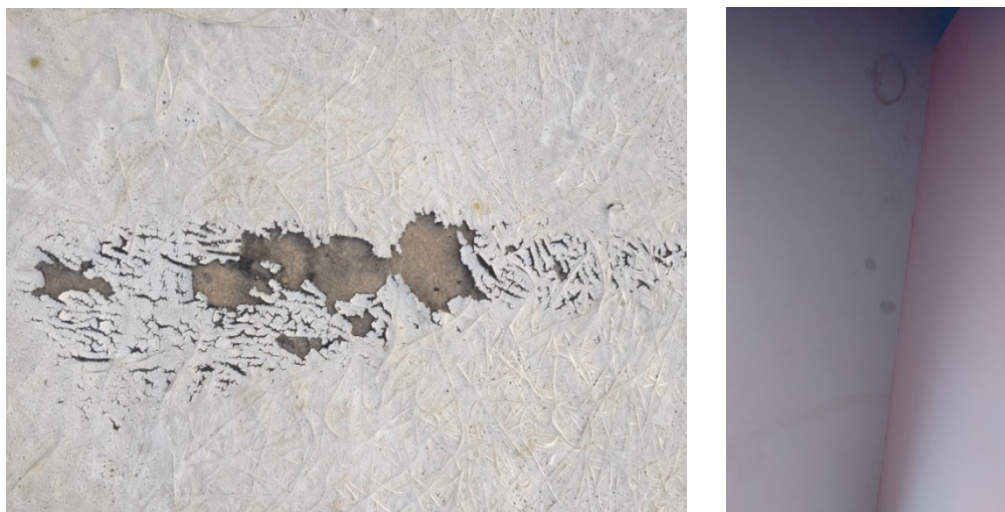
Figure 65 Failing water proofing on the terrace and water stains in interiors
