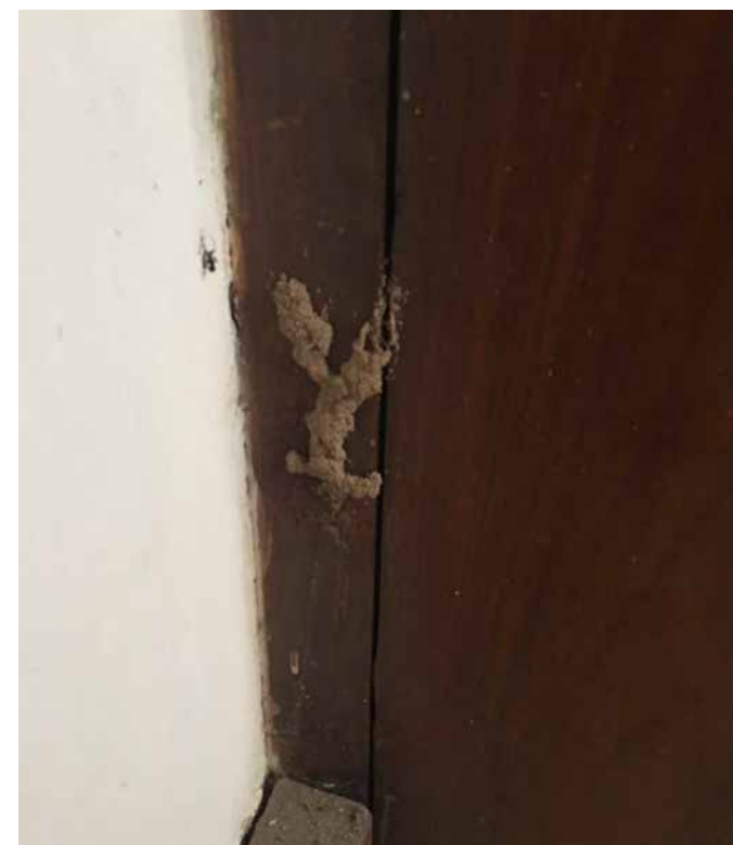
DISINTEGRATED DOOR FRAME DUE TO TERMITE
