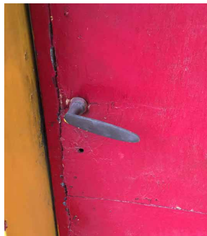
CRACKED PLY DUE TO RUSTY DOOR LOCK
