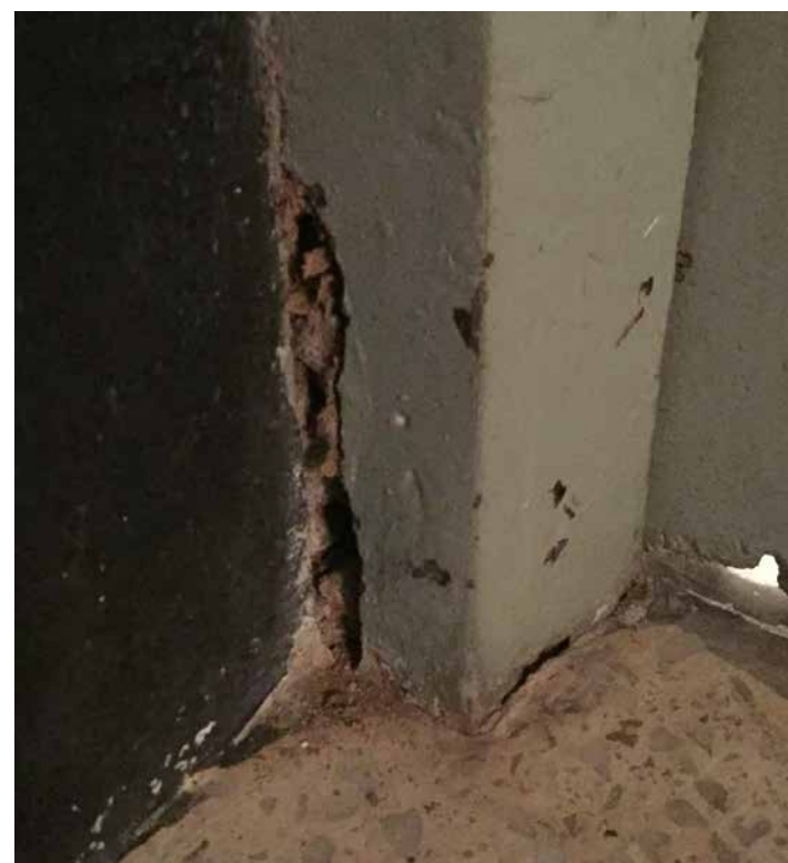
TERMITE INSIDE THE DOOR FRAME
