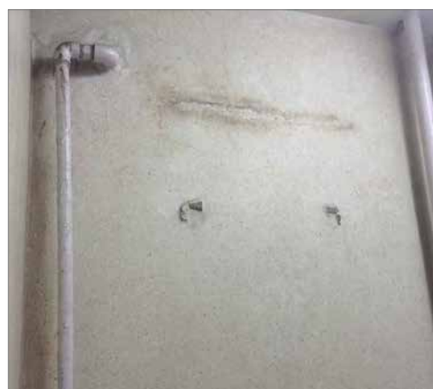
STAINS ON THE WALL SURFACE
