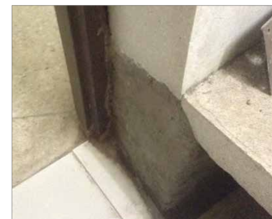
PREVIOUS INTERVENTION WITH CEMENT ON WALL
