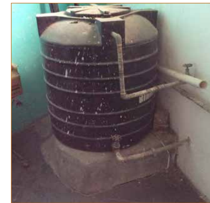
CEMENT FLOOR ADDED ON BLACK TERRAZZO FLOOR IN MEZZ. STORE (MF4)
