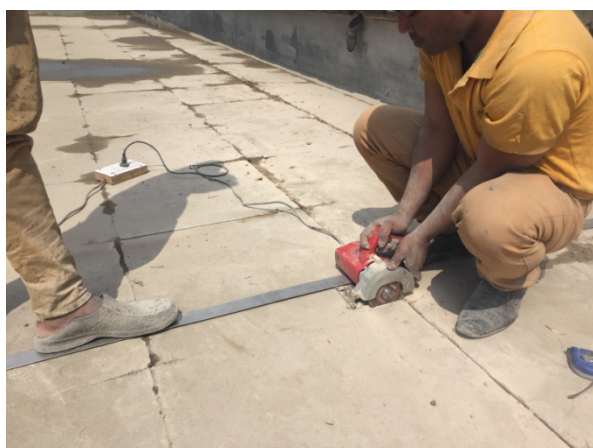
Figure 91 Cutting of floor joints and drilling holes at corners
