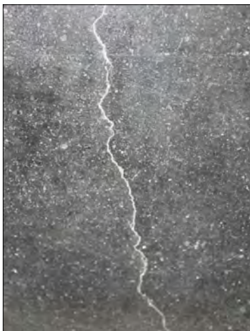
CRACKS IN BLACK TERRAZZO FLOOR IN AUDITORIUM
