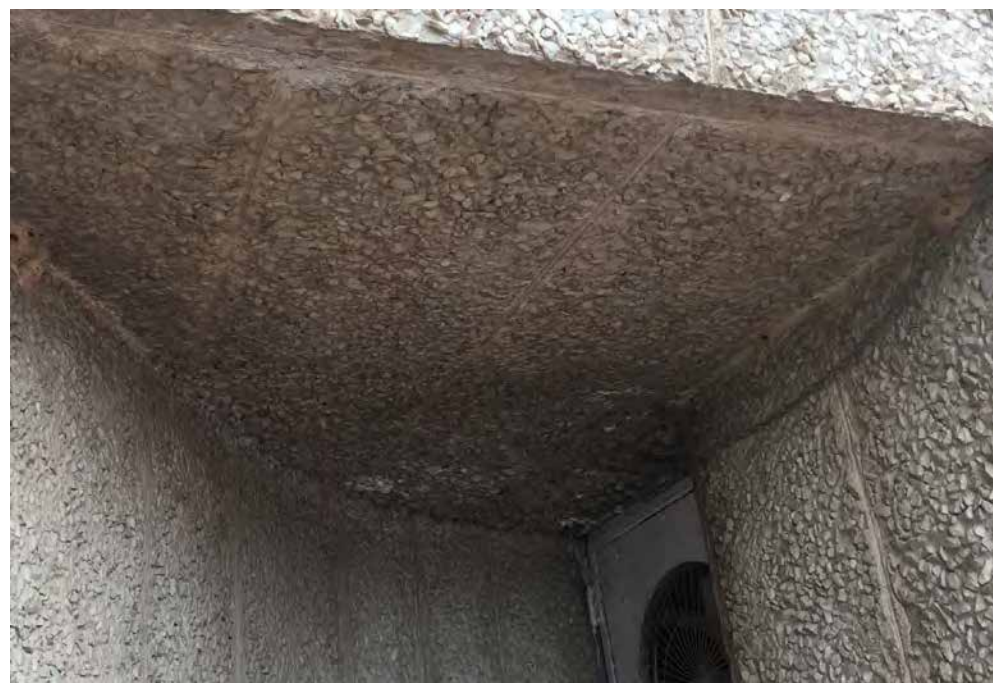
STAINS & ACCUMULATION ON SURFACE
