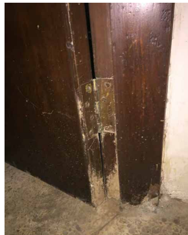
TERMITE ENTERING THE DOOR
