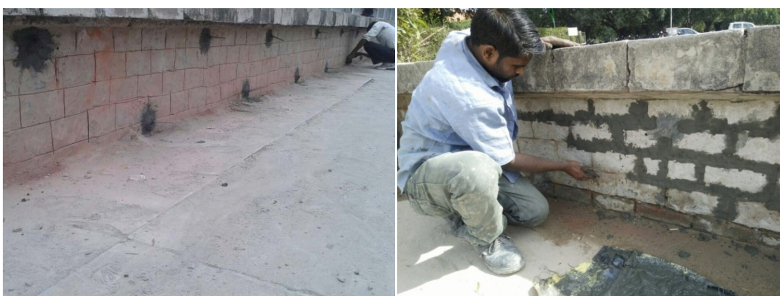
Figure 85 3ft spacing of the nipples covering 5sqft area each and Sealing the joints with High Bond 40 & cement
