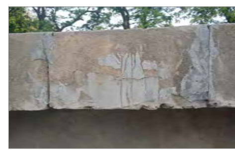
DETACHED POOL PANELS AND PREVIOUS REPAIRS
