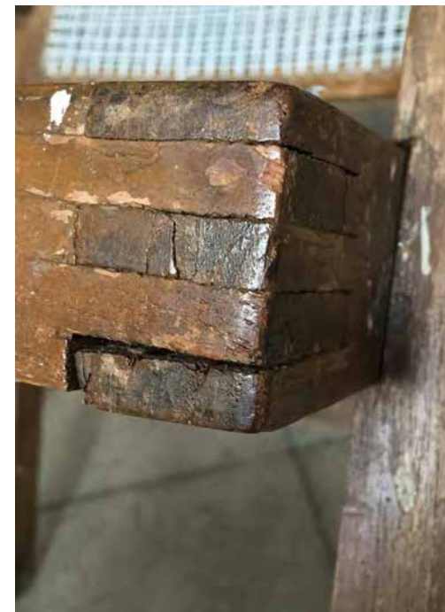
LOOSE JOINT ON FRONT SIDE
