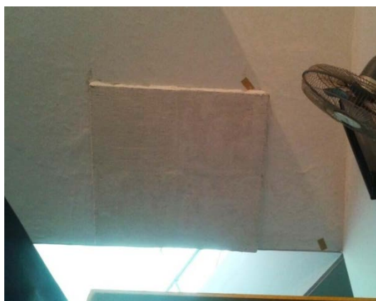
White cement putty base for top layer of paint
