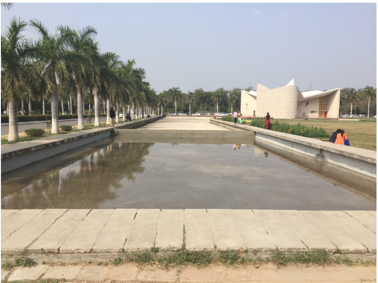
Figure 90 Filling water after waterproofing treatment up-to 20 inches and monitoring for seepage
