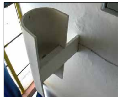
PREVIOUS INTERVENTION OF PAINT ON THE ORIGINAL LIGHTING FIXTURE
