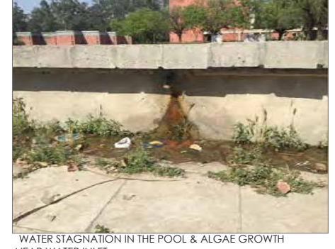
WATER STAGNATION IN THE POOL & ALGAE GROWTH NEAR WATER INLET
