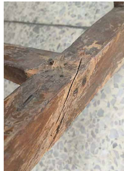
MAJOR CRACK RIGHT SIDE BOTTOM MEMBER
