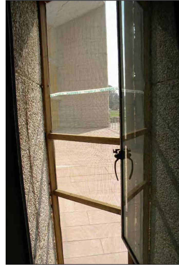
WIRE MESH FRAME INSTALLED ON THE OUTER SIDE
