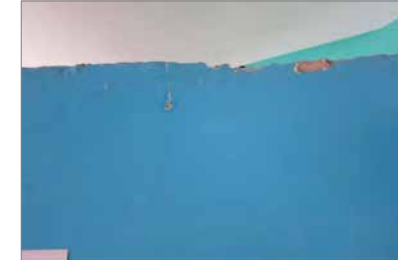
MATERIAL LOSS ON THE WALL EDGE
