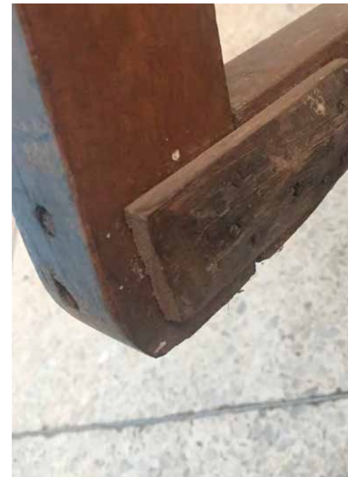
NEW ADDITION / INAPPROPRIATE REPAIR
