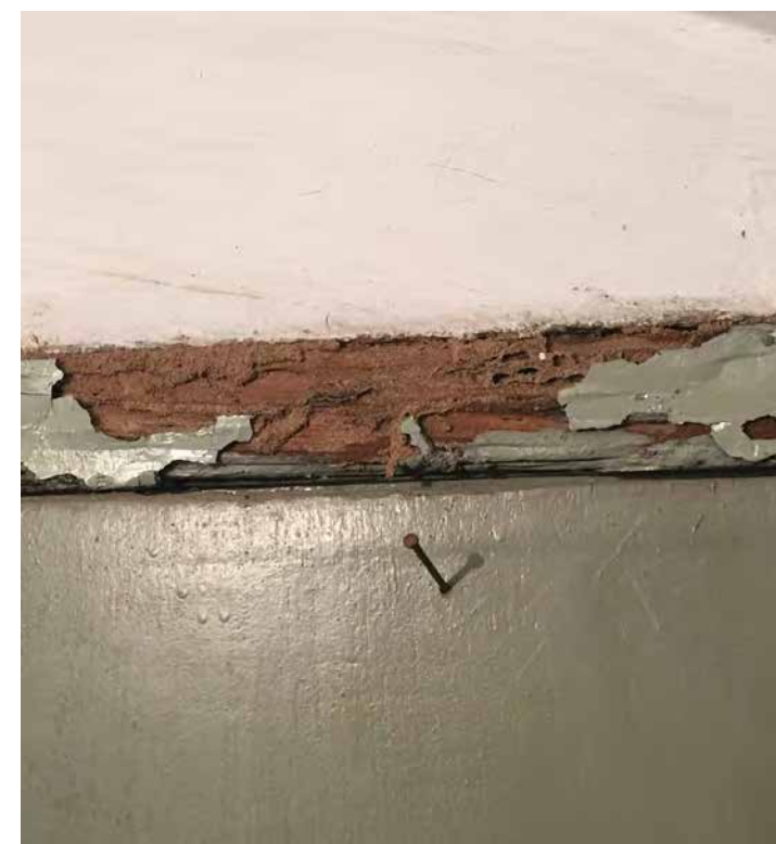
MATERIAL LOSS DUE TO TERMITE
