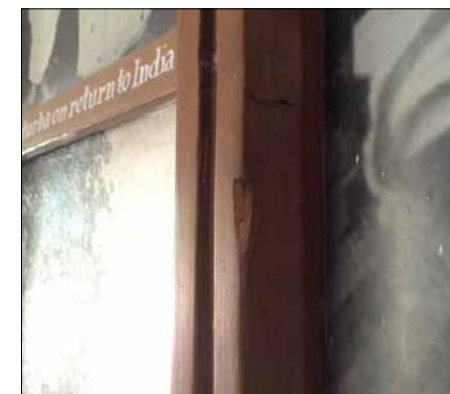
LOSS OF WOOD IN DISPLAY PANEL-1
