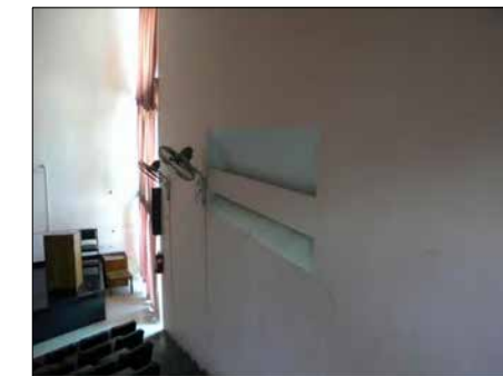
DIRT DEPOSIT ON LIGHTING FIXTURES
