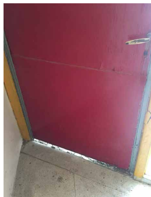
REPAIRED BOTTOM SECTION OF THE DOOR
