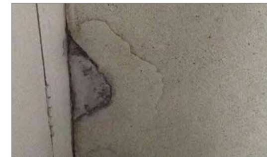
CRACKS IN WHITE TERRAZZO FINISH WALL
