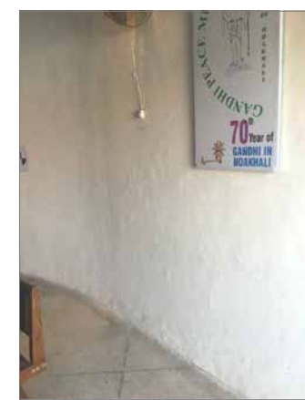
PLASTER DEFECTS ON THE WALL
