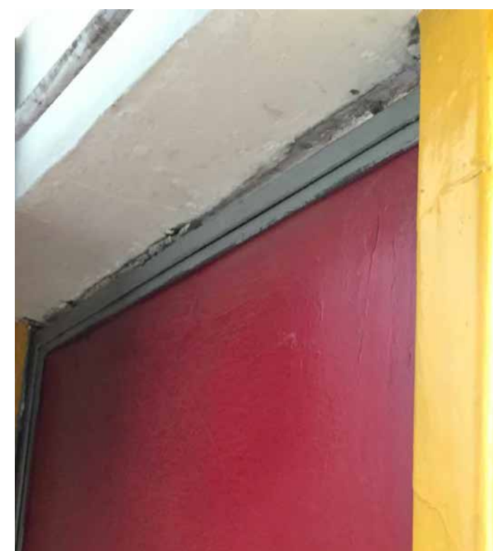
DOOR FRAME DETACHED FROM LINTEL
