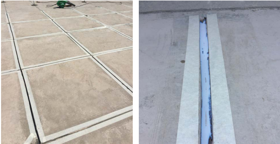
Figure 92 Masking of joint edges with tape and QS- 530 poured into the cut joints
