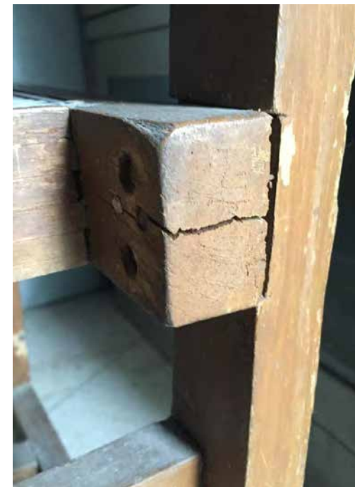
MAJOR CRACKS ON REAR SIDE
