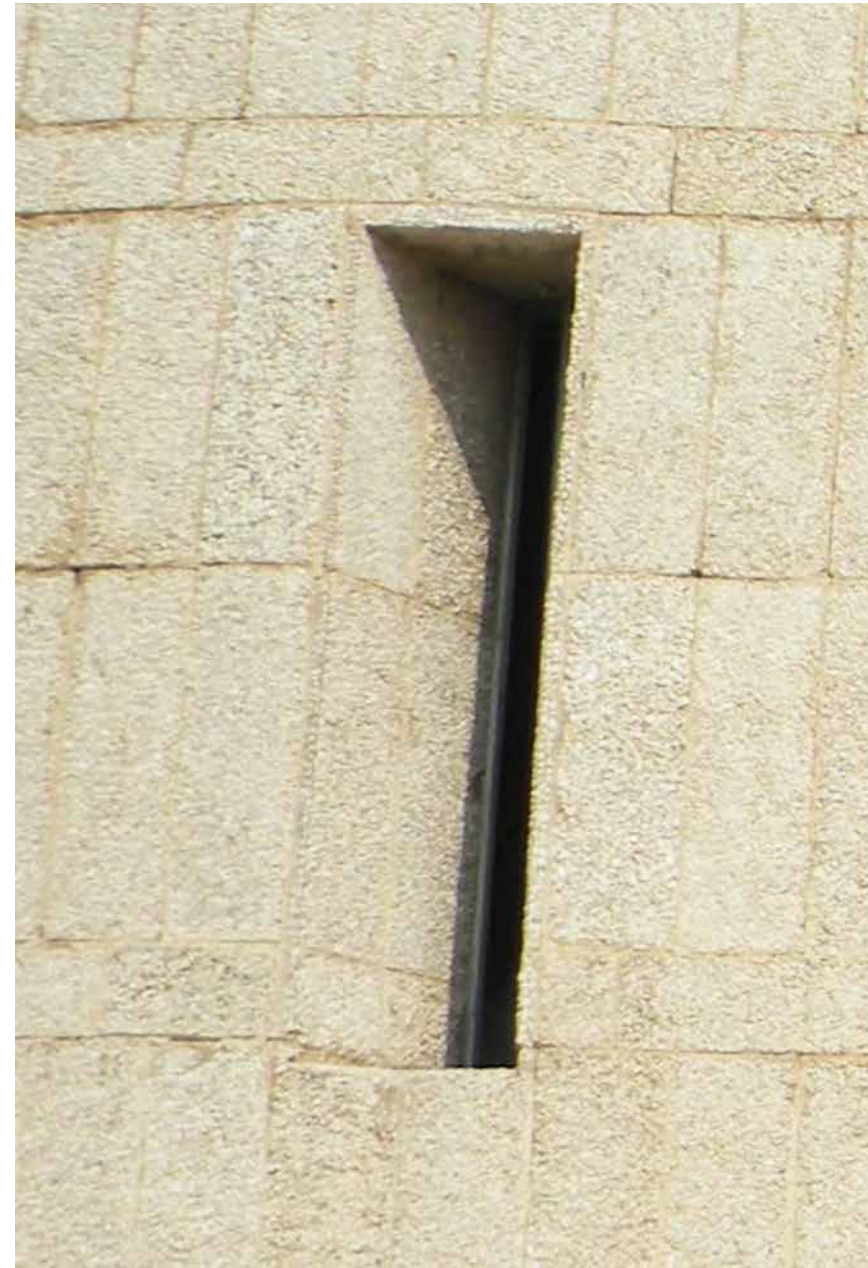
OUTER FACE OF S1
