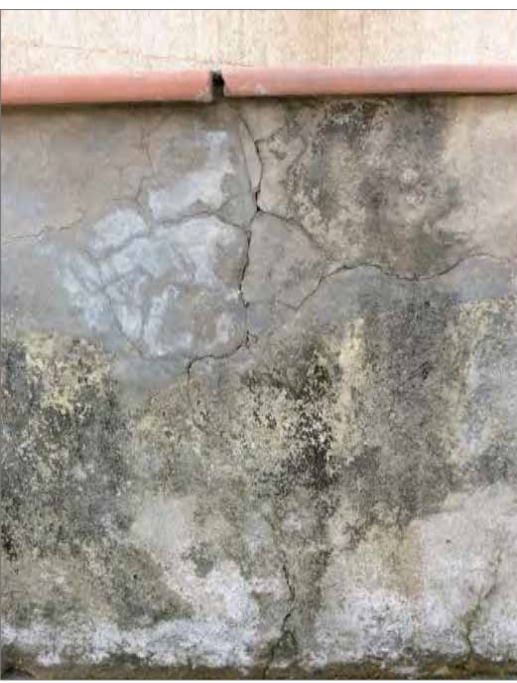
CRACKS & ALGAE GROWTH ON THE BASE OF THE BUILDING
