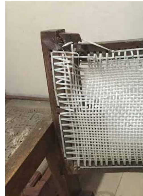
INAPPROPRIATE REPAIR WORK
