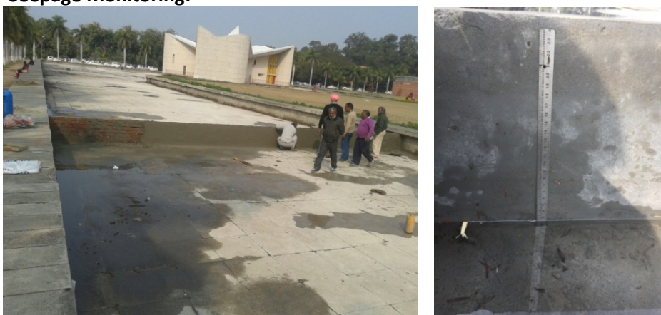
Figure 81 Construction of new wall to enclose 500sq metre area & Setting up graduated staff gauge to measure water level
