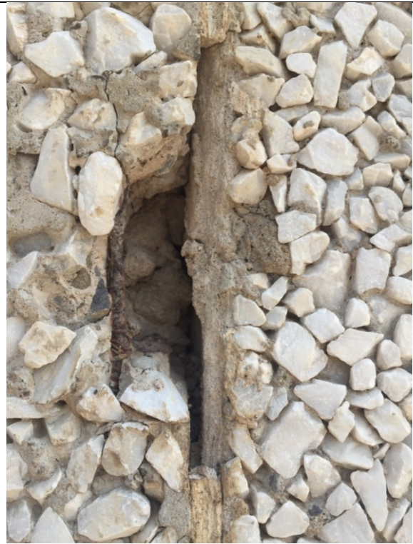
Loss of material and exposed rebars
