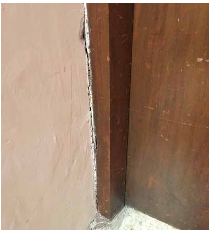
DOOR FRAME DETACHED FROM WALL
