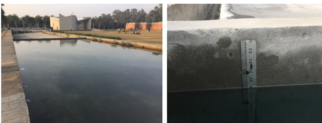
Figure 82 Filling water up to 20 inches and Monitoring for drop in water level
