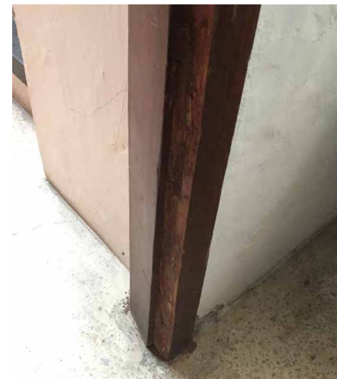
DAMAGED PORTION DUE TO TERMITE
