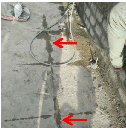
Figure 88 Grout coming out of joints in the floor while pressure grouting
