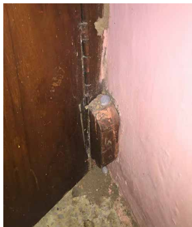
REPAIR WORK ON TOP LEFT CORNER
