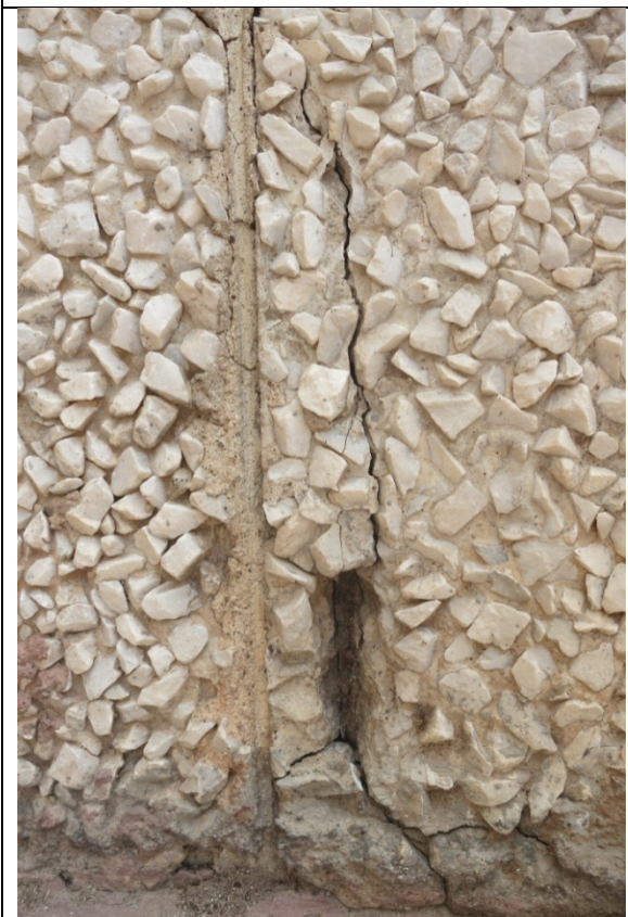
Cracks in the finish layer
