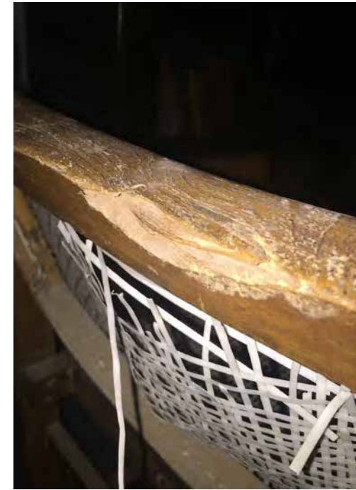
MATERIAL LOSS DUE TO TERMITE ON BACK REST
