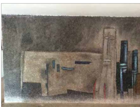
SALT DEPOSIT ON THE MURAL WALL
