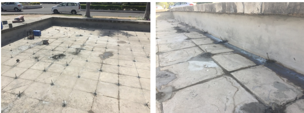
Figure 94 Pressure grouting with manual pressure pump and Grout coming out from the floor joints.
