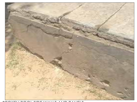
BROKEN POOL SIDE WALLS AND PANELS
