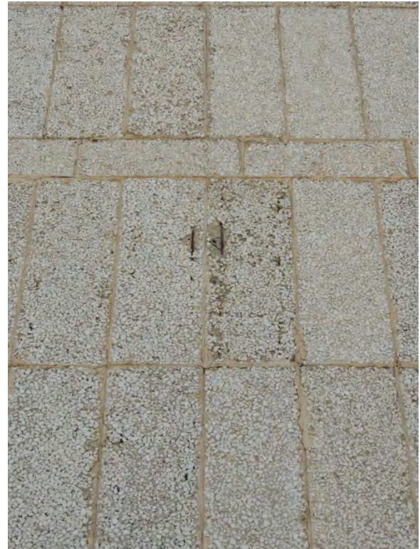
Figure 1.8 Loss of aggregates from Panels
