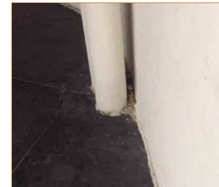
CRACKS IN BLACK TERRAZZO FLOOR (MF3)
