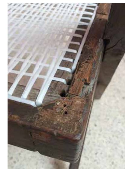
LOSS OF MATERIAL
