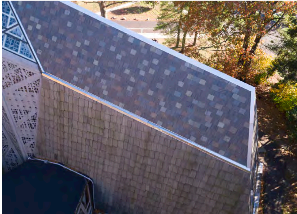
Figure A15. View of roofing and wall slate at the west end of the north elevation. The roofing slate in this area was previously replaced and varies in color from the slate over the Narthex; this work is assumed to be part of the 2003-2007 waterproofing campaign. In accordance with the original design, the roofing slate is laid in uniform horizontal lines while the slate wall shingles exhibit more variation.
