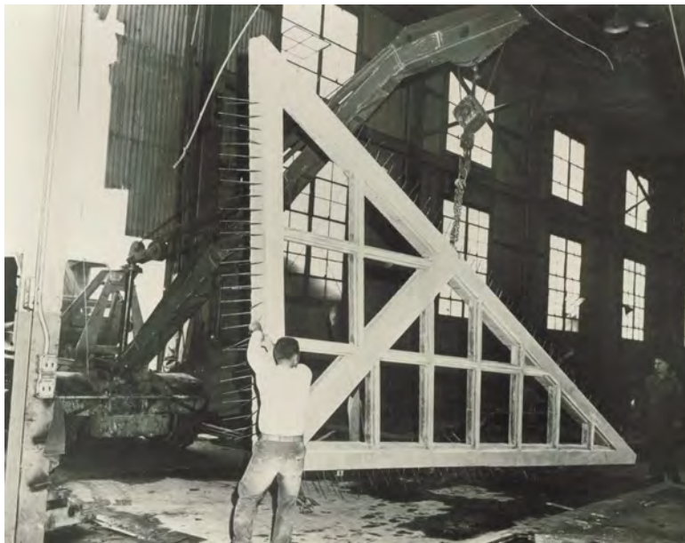
Figure A4. Pre-cast concrete panel in the shop of the Long Island by Precast Building Sections, Inc. The two rows of rebar protruding from the edge of the panel were wrapped around the rebar installed between the panels when set in place on site. Courtesy of the First Presbyterian Church of Stamford archives.
