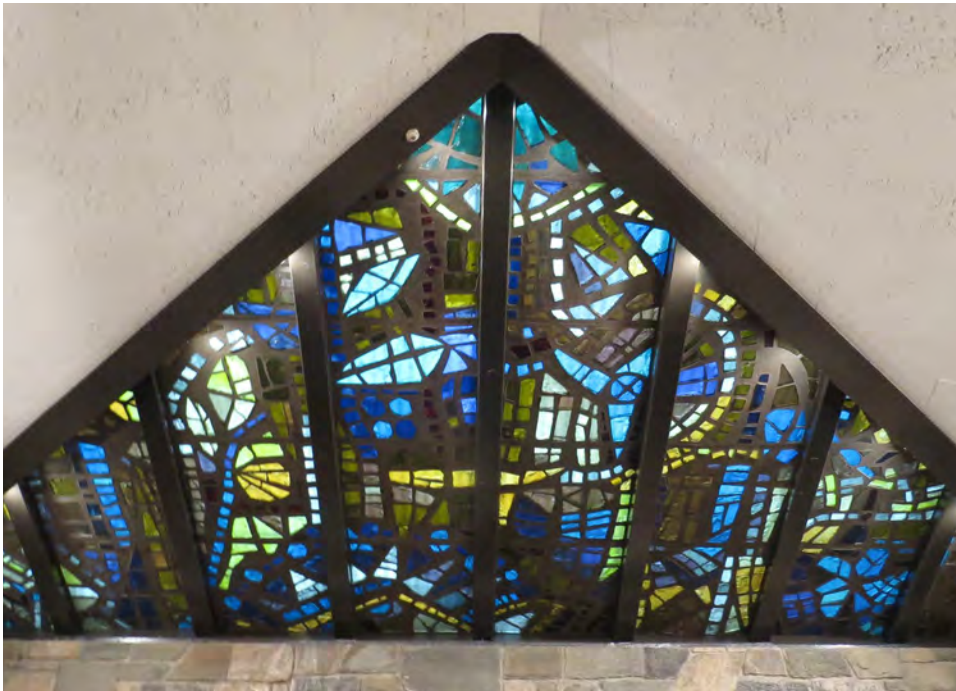
Figure A18 Existing dalle de verre in the Chapel with painted framework.
