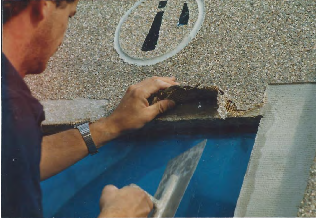
Figure 35 (above): Removing STO coating. Source: Rohlf Archive.
