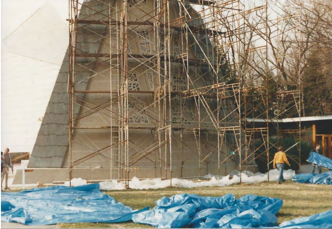
Figure 32 (above): Scaffolding installed during the 1980s Sanctuary restoration. Source: Rohlf Archive.
