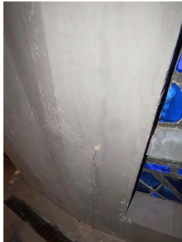
Typical vertical crack at the interior, where pre-cast panels abut cast-in-place concrete framework.
