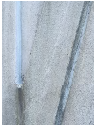
Typical failing sealant between the pre-cast and cast-in-place concrete on the north elevation.
