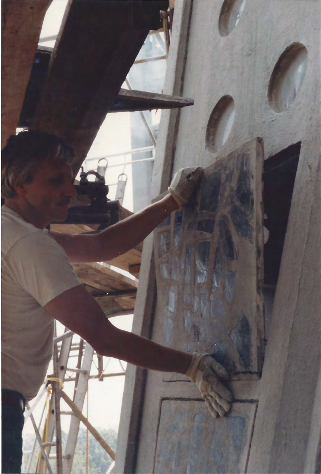
Figure 34: Removing dalle de verre panels. Source: Rohlf Archive.
