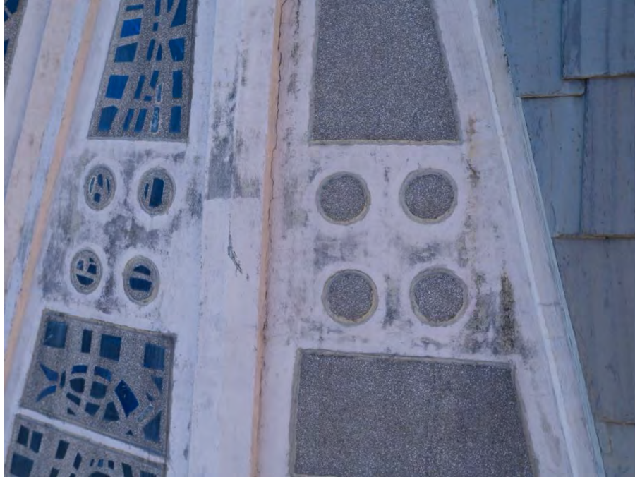
Above: Aerial image of the east elevation (narthex), panel E1, showing replacement dalle de verre in epoxy matrix.
