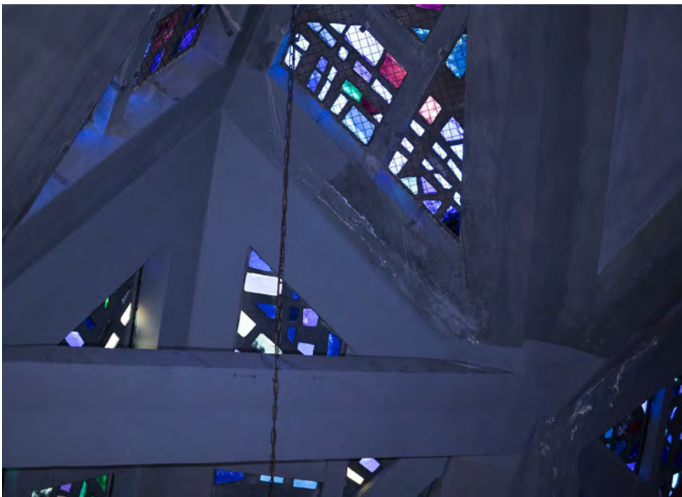
Figure A22. Interior work was not performed above the roofline in 1986. The interior painting stops at this level, as shown here.
