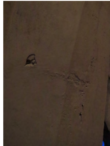
Typical pitting on interior concrete framework surface.
