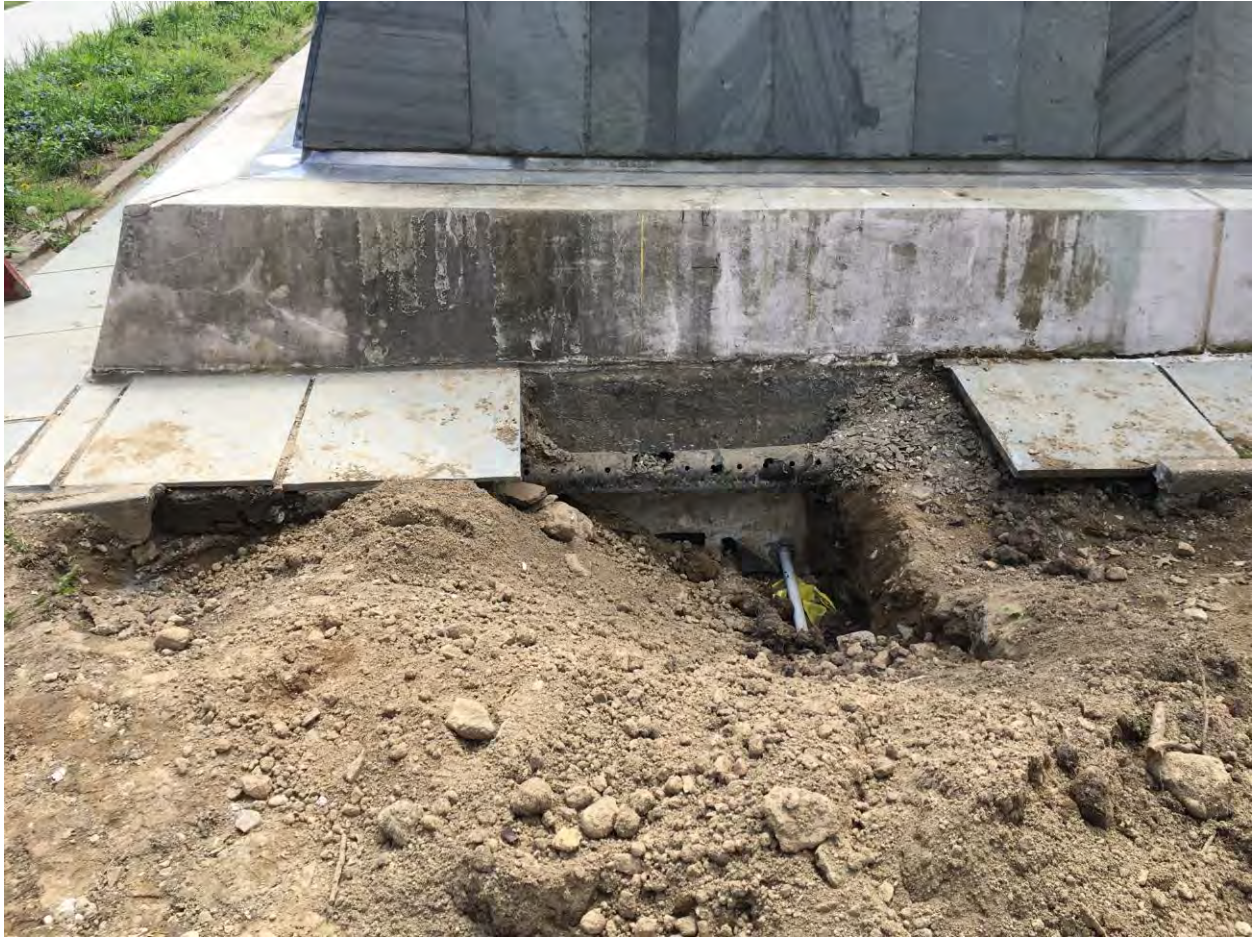
Figure 43: Exposed defunct foundation drain (northeast). Photo by Prudon and Partners. 5/02/2017
