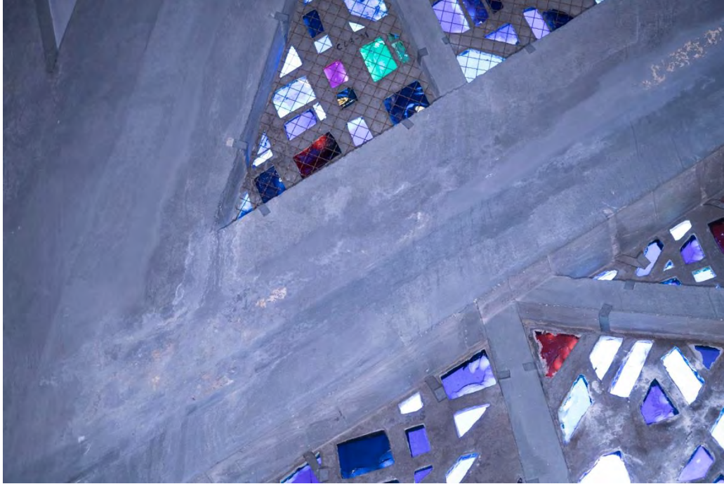
Figure 16 (above): Roof line damage. Photo by Propellerheads.
