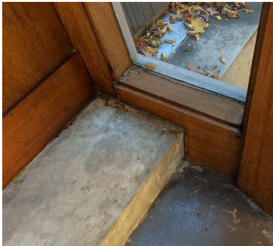
Figure 23 (below): Conditions at connecting link and north facade. Photo by Prudon & Partners.
