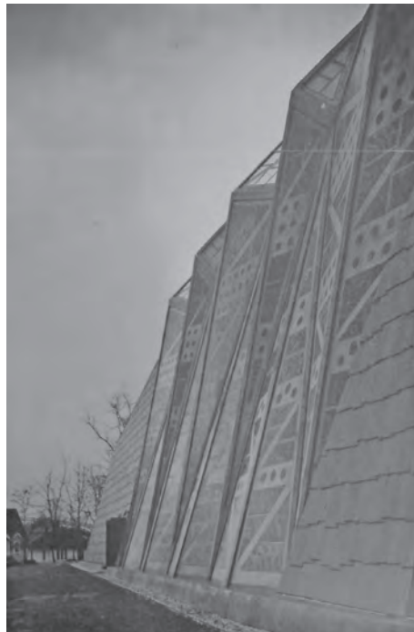
Figure A12. Archival image of completed Sanctuary showing protective glazing panels at skyward facing dalle de verre. "A Brilliant Canopy for Worship," Architectural Forum, April 1958, 107.
