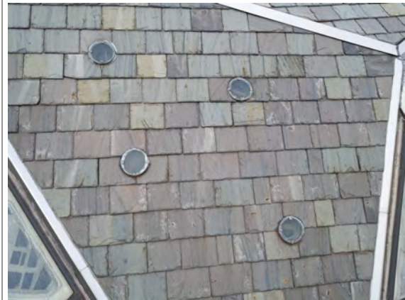
Typical efflorescence visible on isolated slate.
