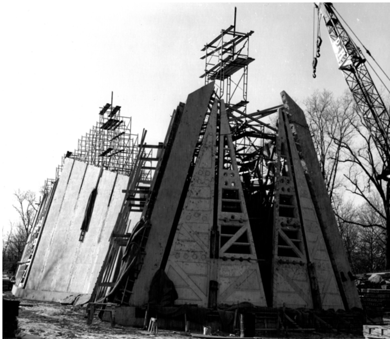
Figure A8. Construction of Sanctuary. The small solid panels installed at the openings in the east elevation match the larger pre-cast concrete panels and were installed before the dalle de verre. Courtesy of the DeLuca Construction Company archives.
