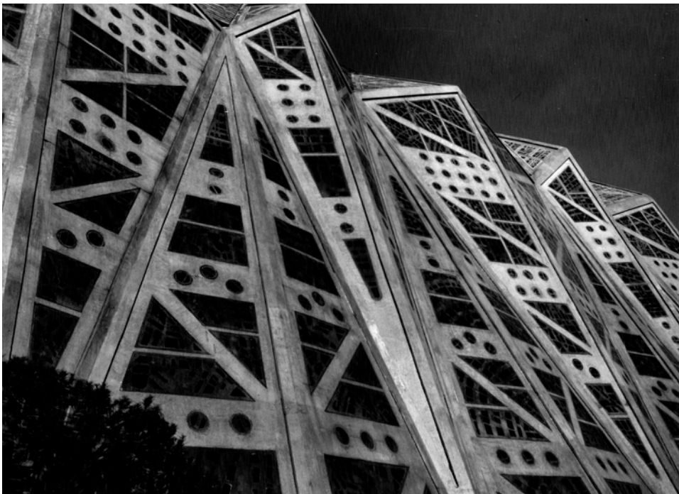
Figure A14. Completed Sanctuary façade coated with the original clear waterproofing coating and protective glazing at the skyward facing panels above the roofline. The dalle de verre appears darker than the adjacent pre-cast and cast-in-place concrete. Courtesy of the DeLuca Construction Company archives.
