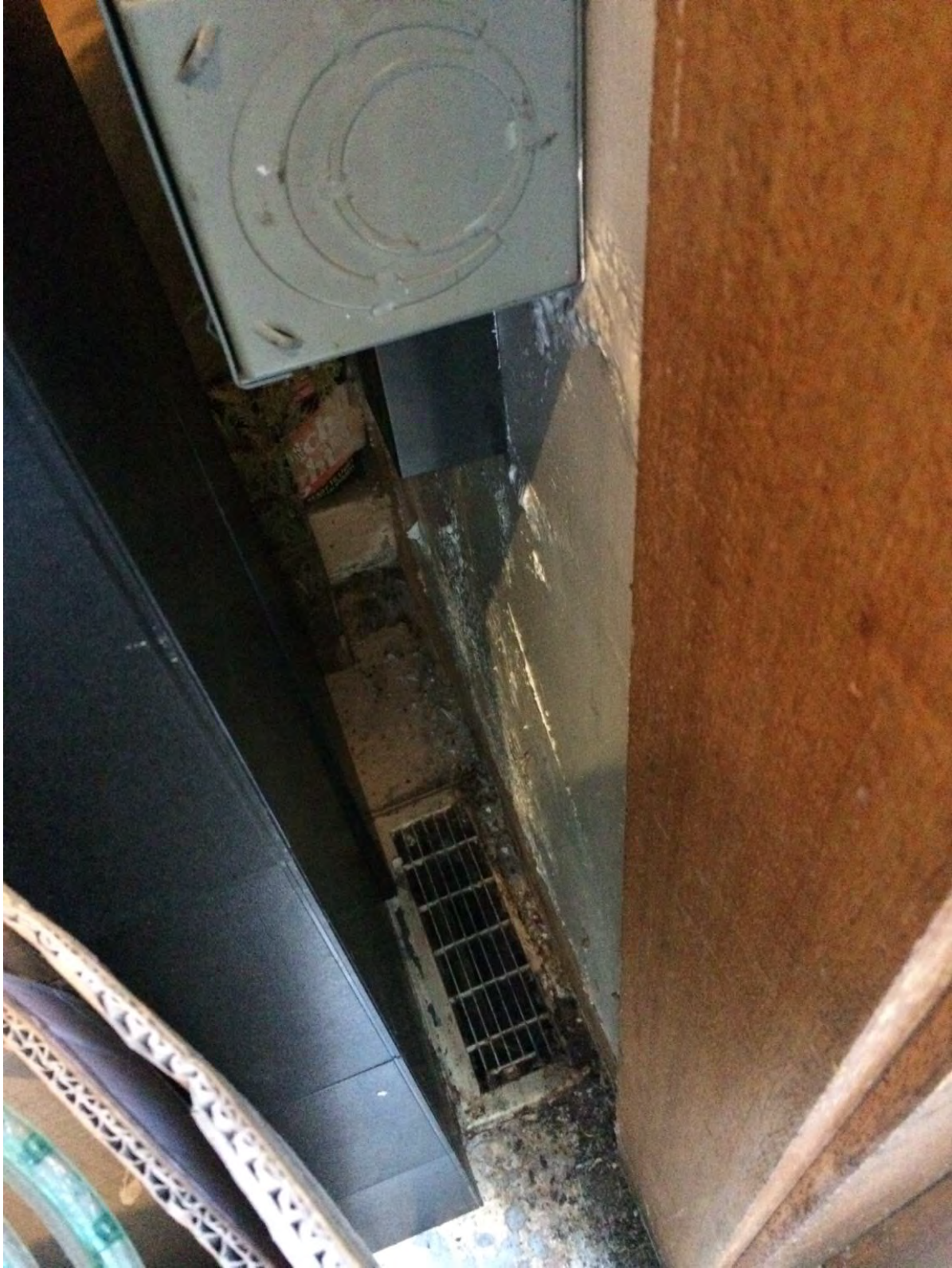
Figure 15: Condition at Choir wall interior. Photo by Prudon & Partners.
