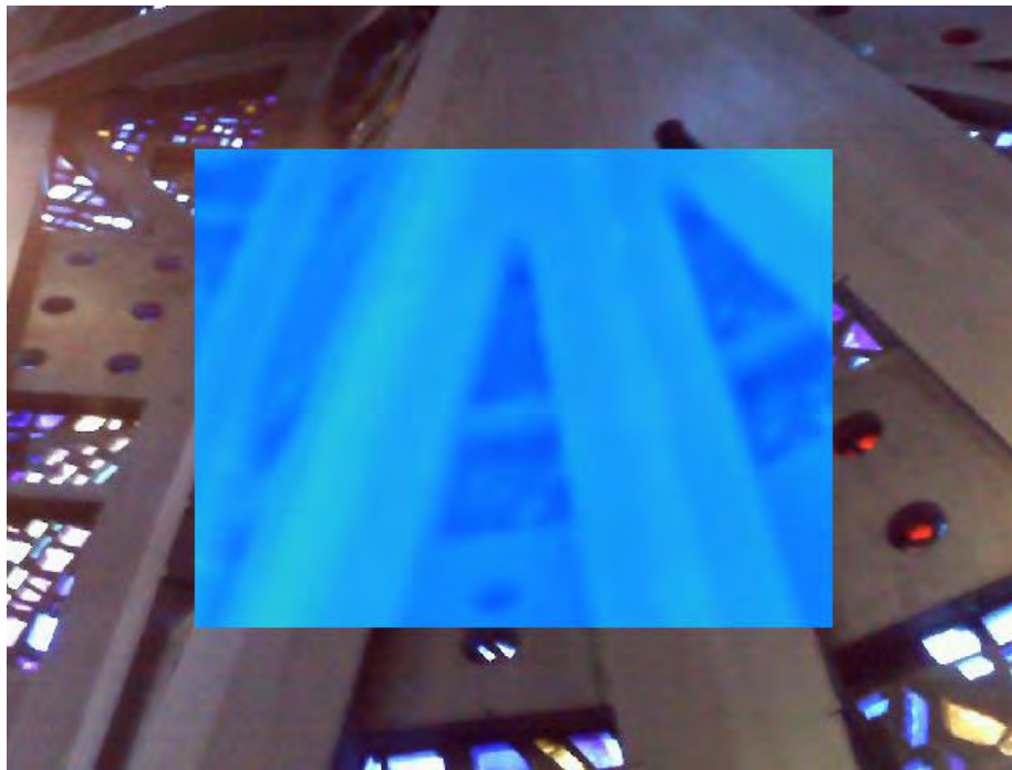
Figure A26. Thermogram of interior north elevation in January 2017. Thermogram processed to show range of temperatures 55 (Blue) -100 (Red). The temperatures of the materials on this elevation were substantially cooler than those on the interior of the south (Figure A27).
