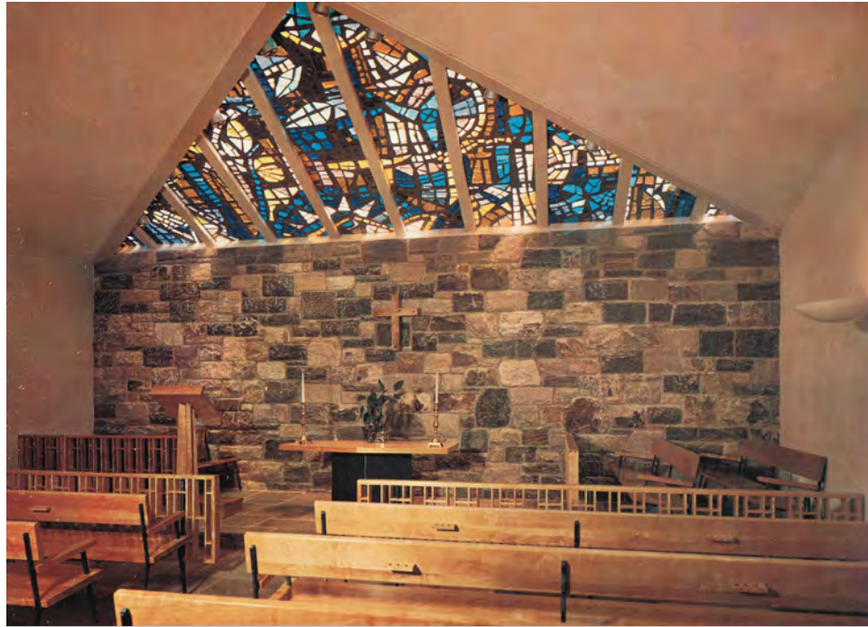
Figure A19. Archival image of dalle de verre in Chapel. The framework between the dalle de verre panels is identified as wood on archival drawings and is painted a light color to match the walls, in contrast to the current dark finish (See Figure A18). Courtesy of the First Presbyterian Church of Stamford archives.
