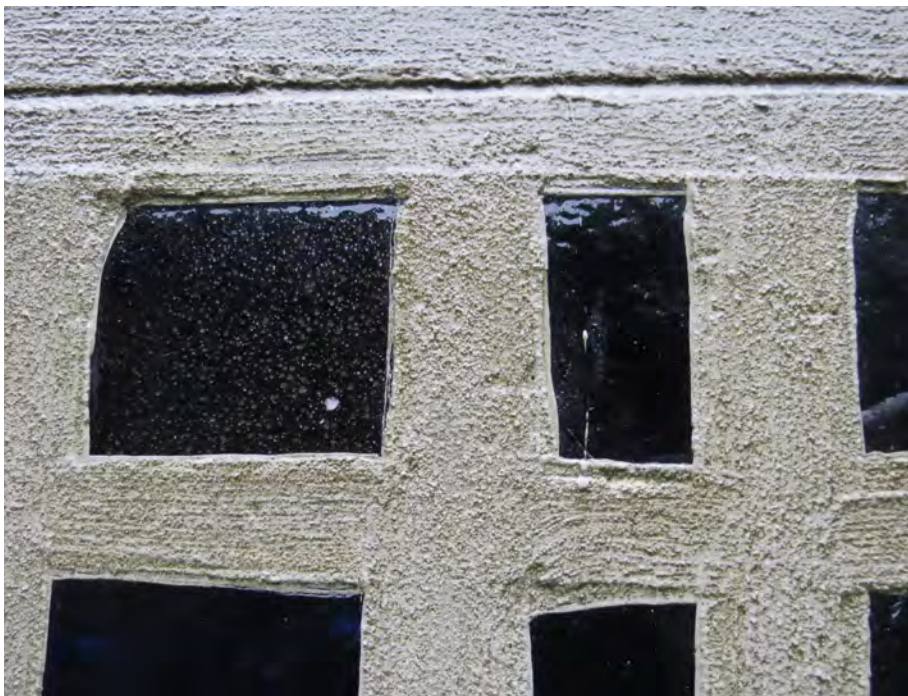
Figure A28. Typical application of the exterior concrete coating on the north elevation. The 2003 report by Hoffman Architects, Inc. suggests this coating was applied in 1994. Note the coating overlaps the edges of the glass.
