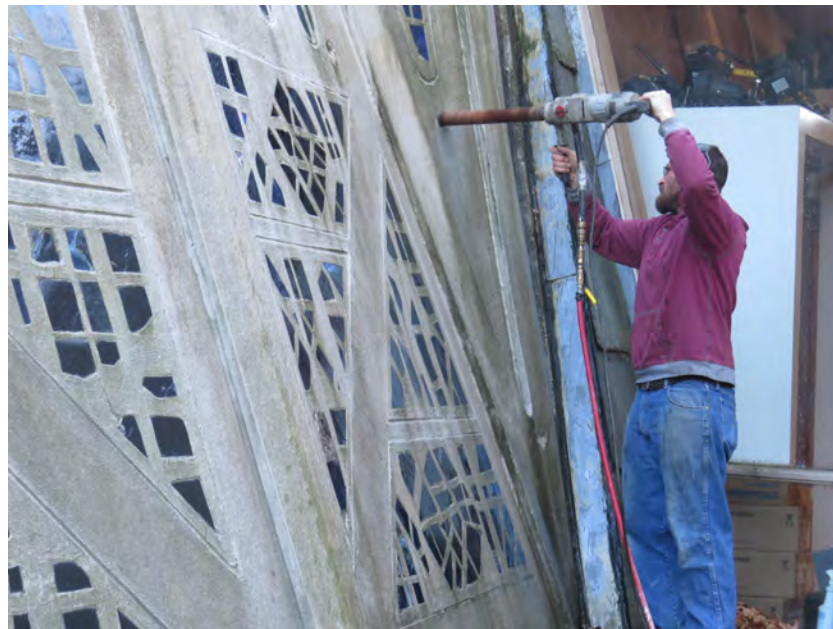
I Removal of core at sample location #2.
