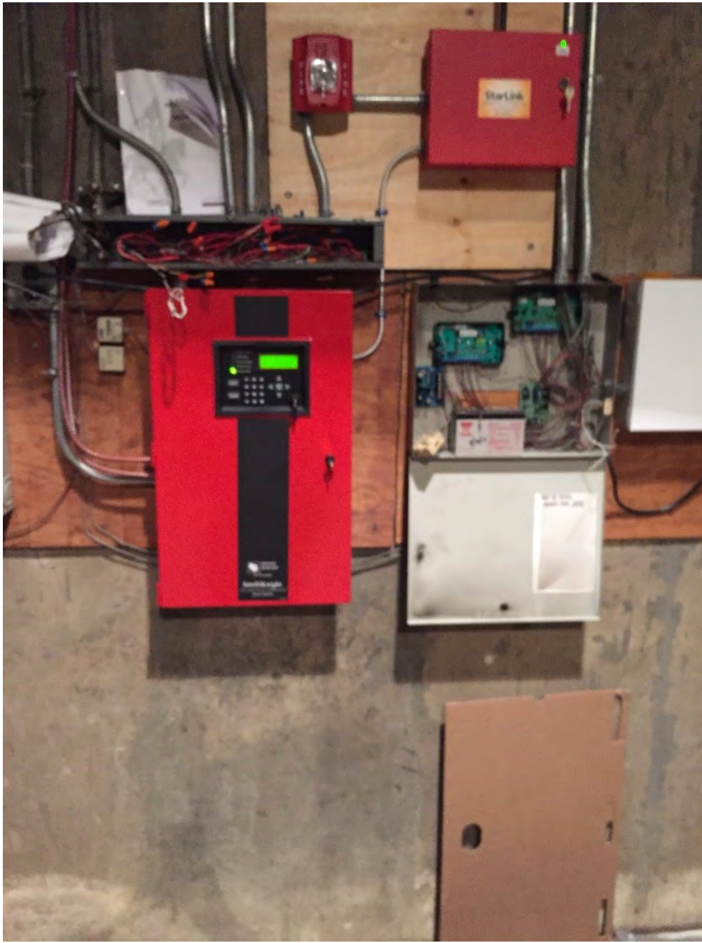
Picture#9-Fire Alarm System
