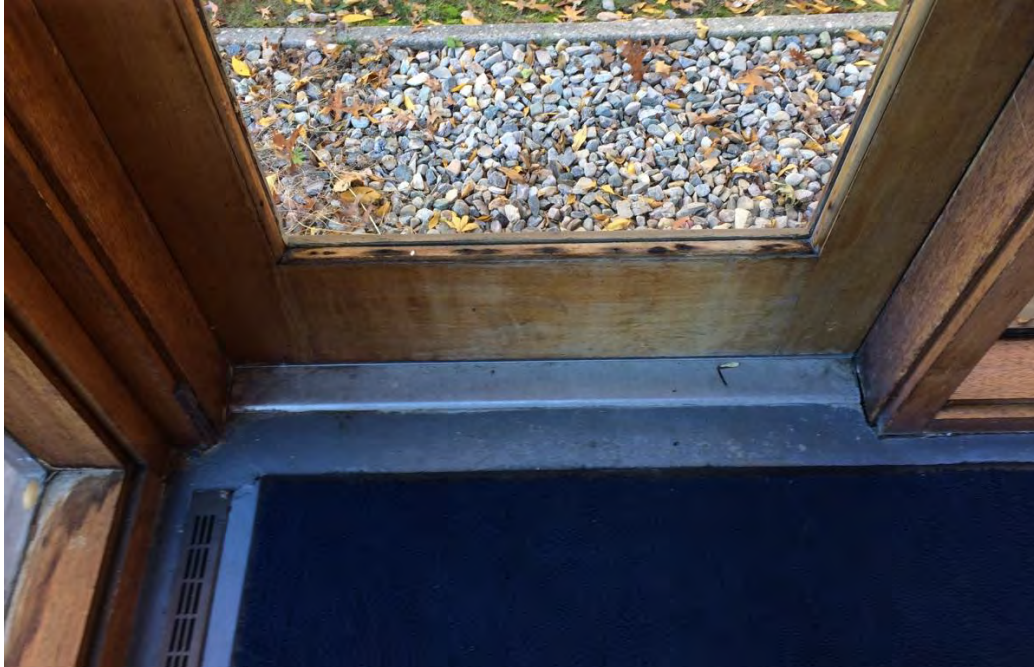
Figure 24: Conditions at connecting link. Exit to memorial garden (wood damage). Photo by Prudon & Partners.
