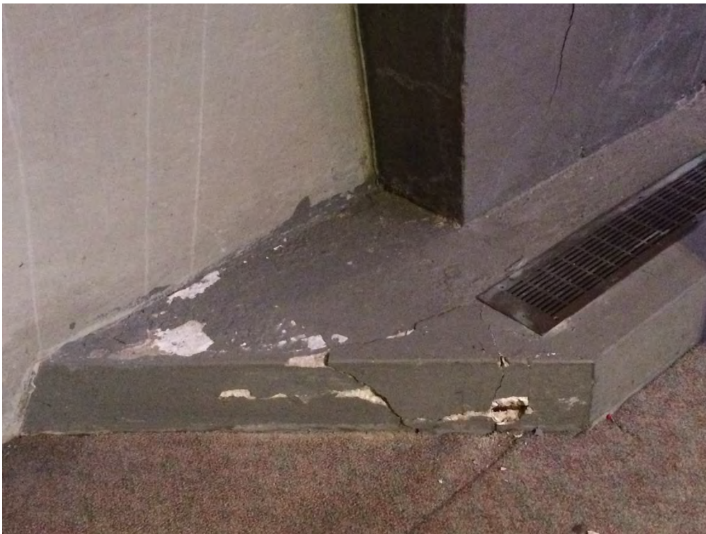
Figure 17 (below): Base damage. Photo by Prudon & Partners.
