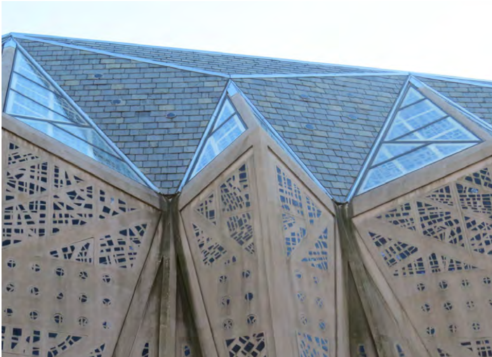
Figure A13. Existing aluminum framed protective glazing on the north elevation showing that the frames do not fully coincide with the pre-cast concrete and dalle de verre patterns. The pre-cast concrete below the glass exhibits a previously applied waterproofing coating.
