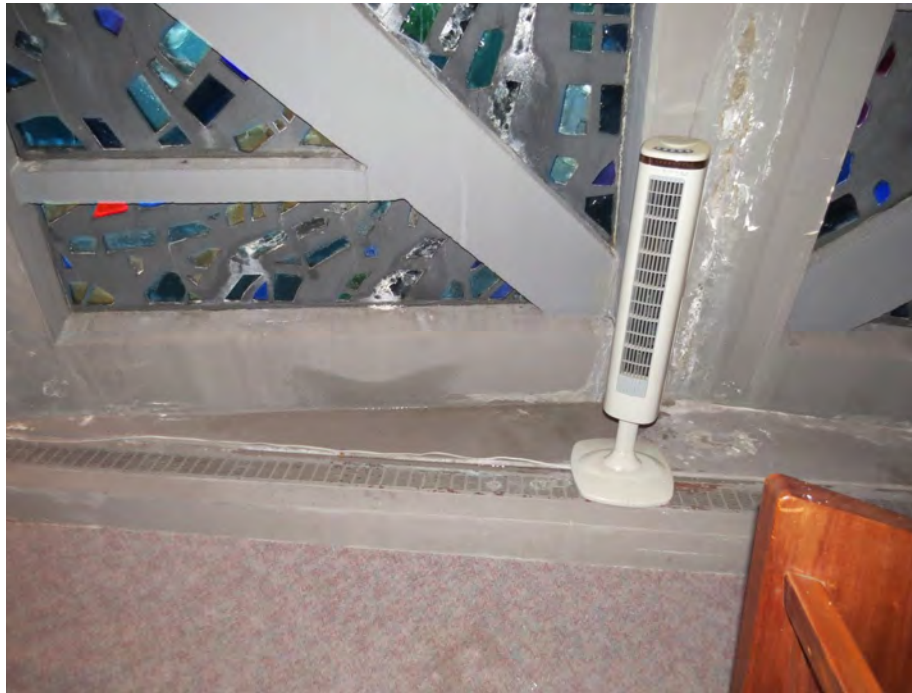
Figure A30. Water pooling at the base of the south elevation during a heavy rain in October 2016.
