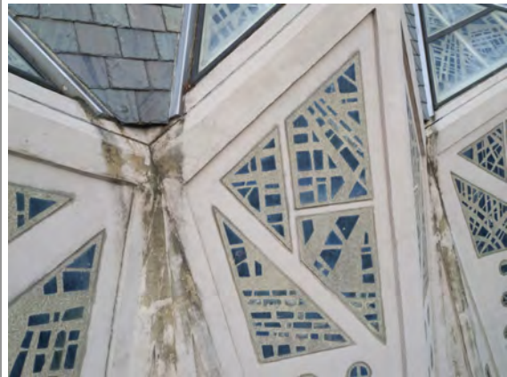
Reglet installed at roof line during 1980s restoration campaign. The sealant and concrete coatings are typically deteriorated at the valley where the roof and wall panels connect. See Condition 8A for typical interior damage in these areas.
