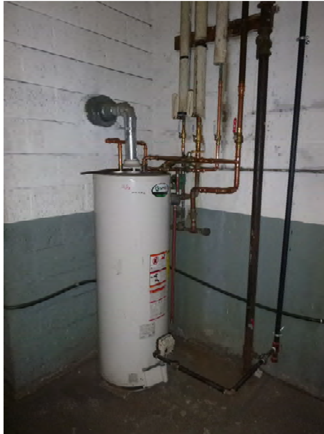
Picture#5-AO Smith Hot Water Heater
