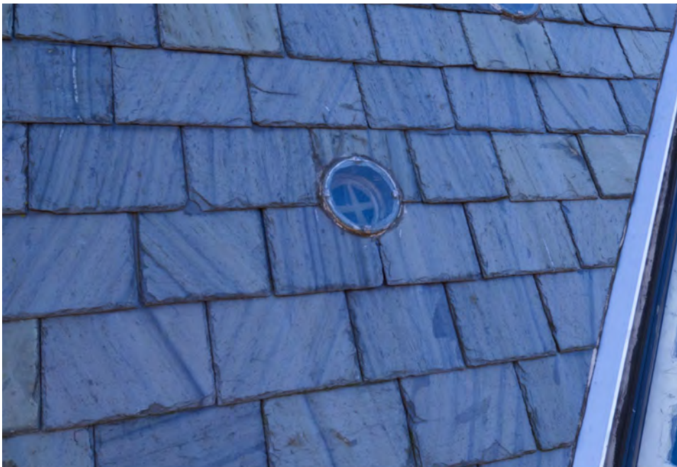
Figure A10. Typical existing portal window with protective glazing, installed in area of roofing slate. Sealant at the perimeter of the protective glazing typically appears to be deteriorated.
