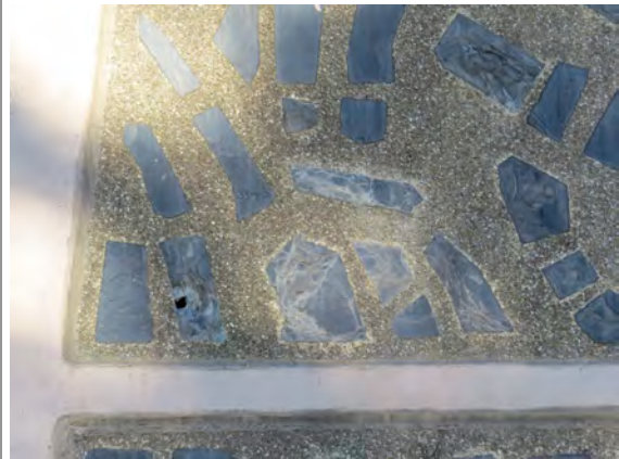
Hole in glass dalle in epoxy dalle de verre panel.
