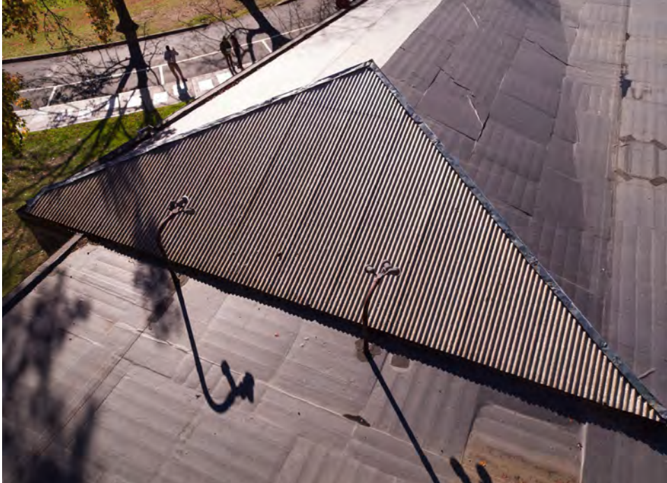
Figure A17. Existing roof protection over dalle de verre in Chapel and two existing light fixtures.
