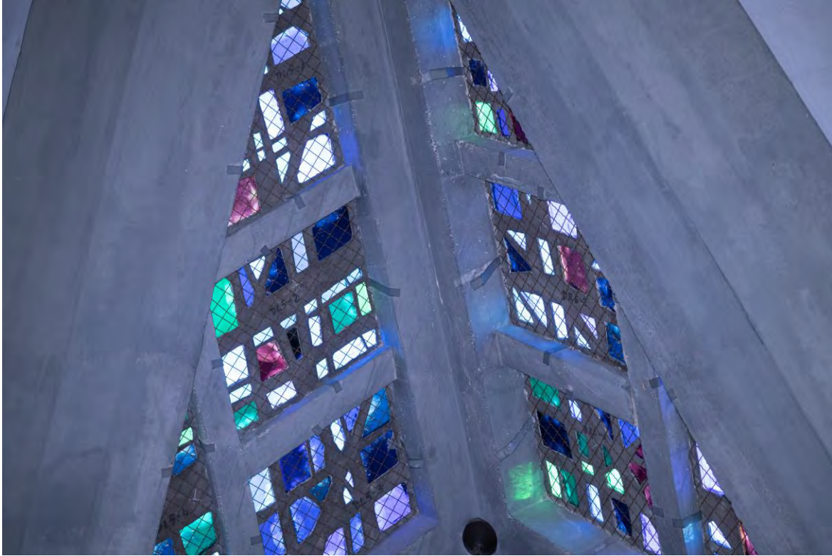
Figure 14: Conditions at interior south roof panels S21 and S22. Photo by Propellerheads.
