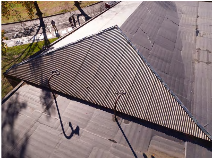
Below: Image of the exterior of the chapel, showing condition of the original corrulux protective material and lighting. Photo by Propellerheads, November 2016.
