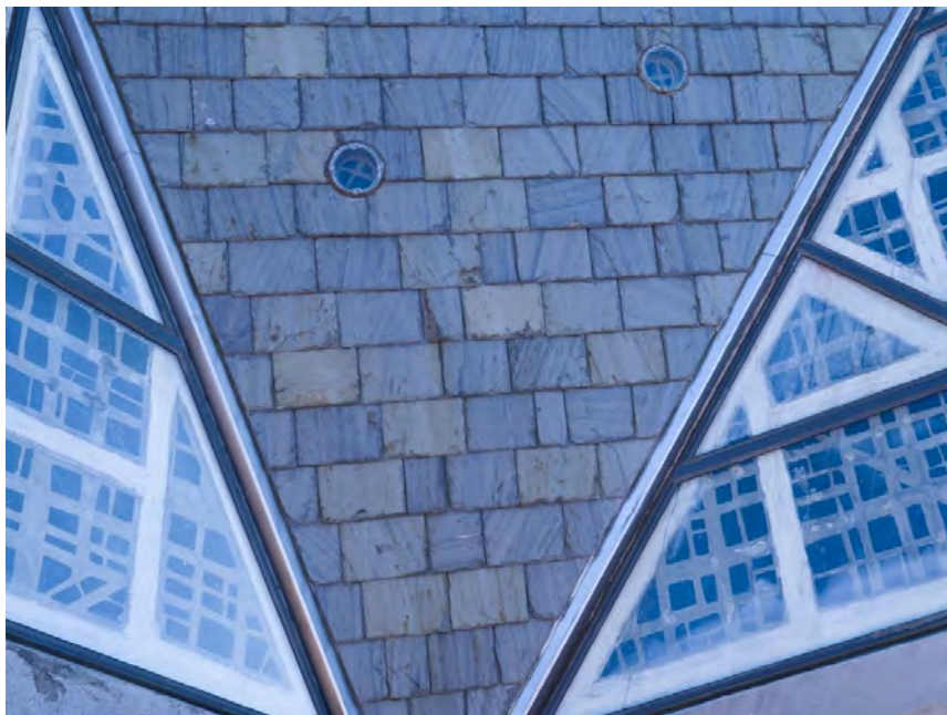
Below: Aerial image of the north elevation (nave), between panels N21 and N20, showing condition of roof slate, original dalle de verre in concrete matrix with secondary glazing, and dalle de verre portals.
