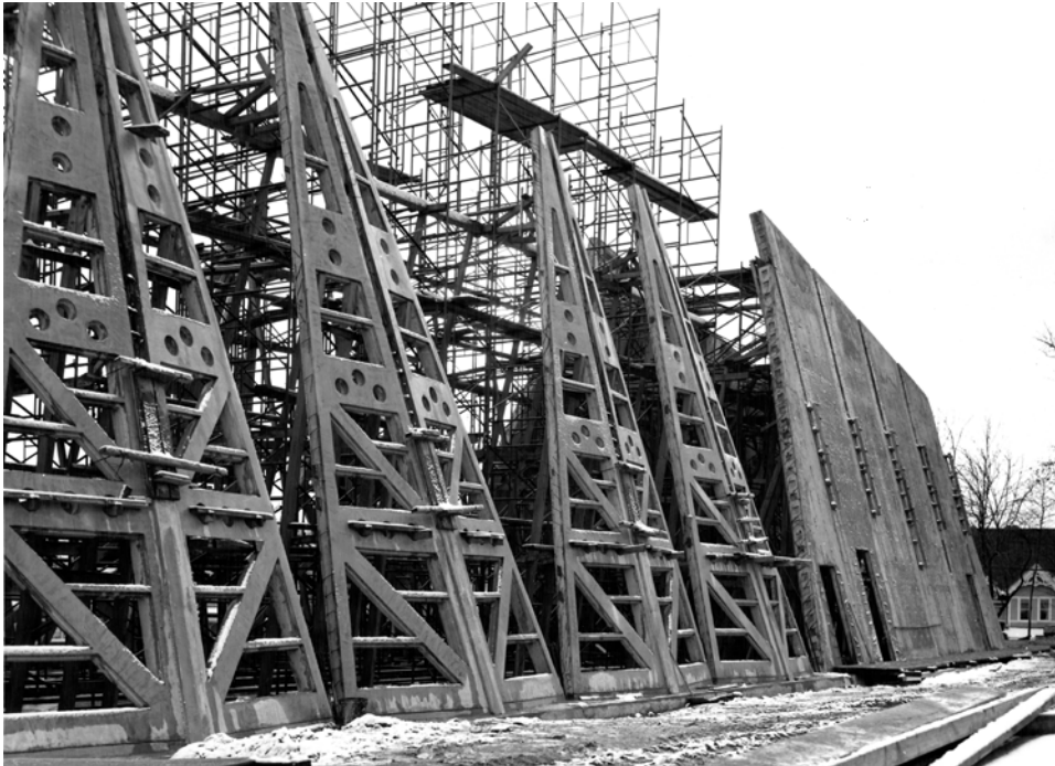
Figure A3. Triangular and quadrangular pre-cast panels installed on site. The cast-in-place concrete is the process of being built up between the triangular panels, which are anchored to the concrete foundation. The concrete ribs were poured in lifts using a 6-foot long form. Courtesy of the DeLuca Construction Company archives.
