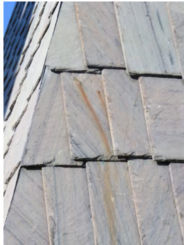
Typical ferrous stains from inclusions in the slate.
