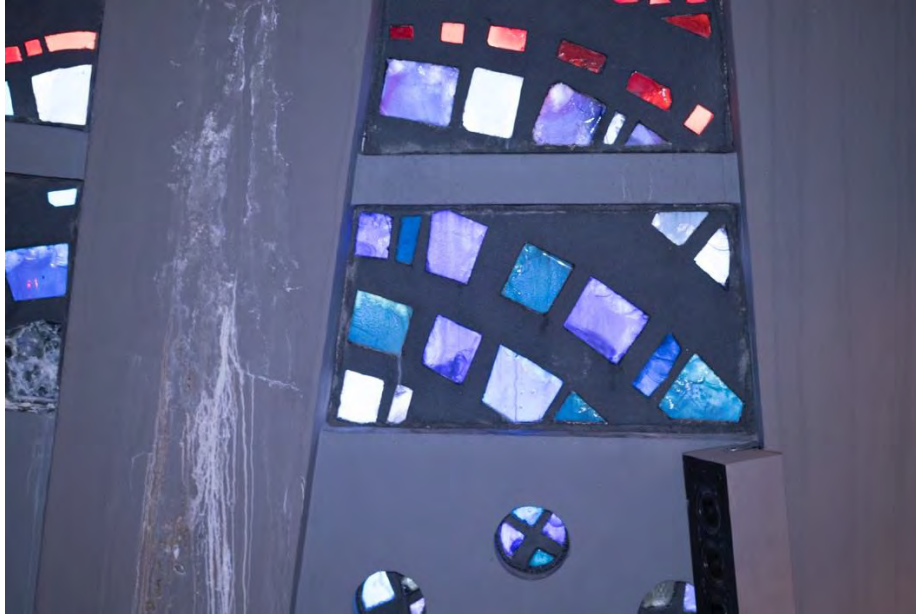
Above: Interior image of the south elevation (nave), panel S7C, showing efflorescence on the poured-in-place concrete, condition of replacement dalle de verre in epoxy matrix. Photo by Propellerheads, November 2016.
