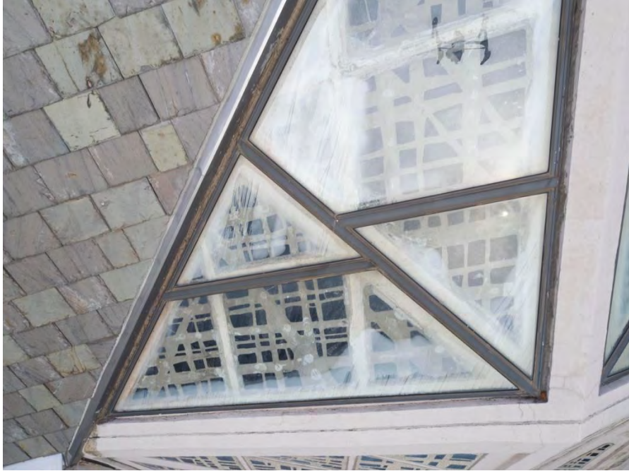
Figure 22 (above): Condensation at roof panel secondary glazing. Photo by Propellerheads.
