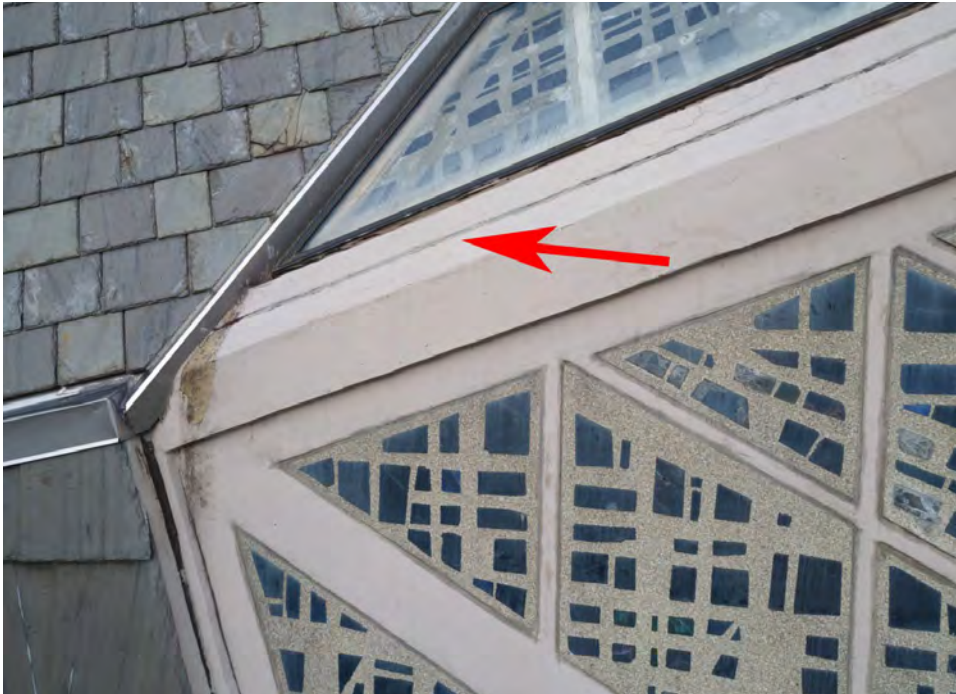
Figure A21. Red arrow indicates the reglet cut at the roofline on the south elevation in 1986. See the archival detail for this work in Figure C3. The reglet was also installed on the east elevation. The reglets are currently filled with sealant. The STO product installed in this area in 1986 was identified for replacement with a new coating during the 2003-2007 waterproofing campaign.
