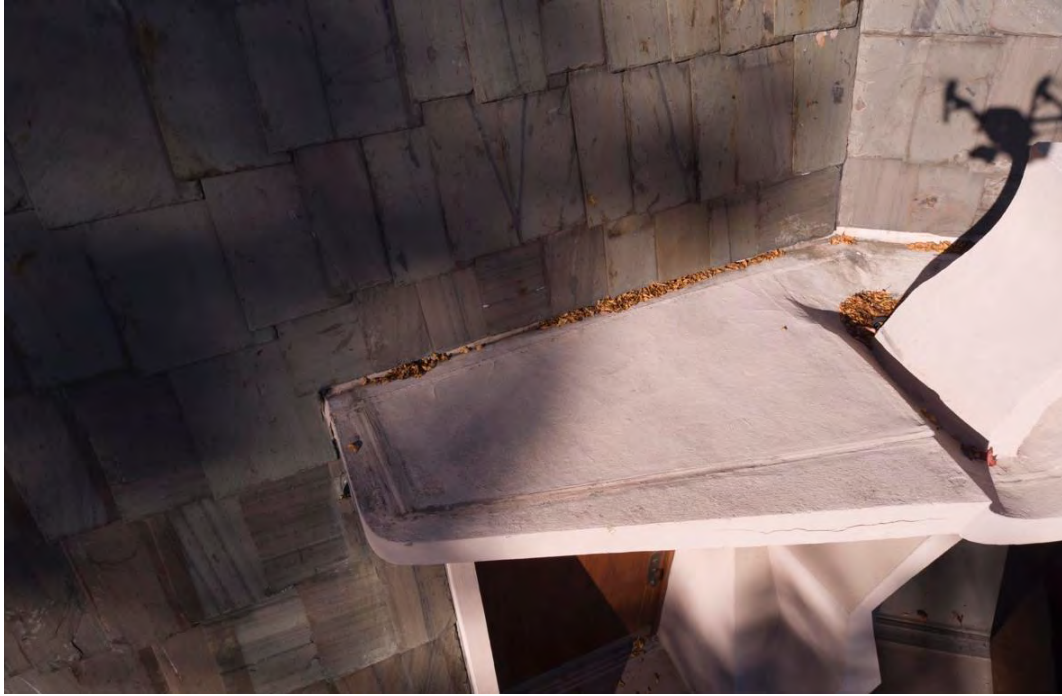
Figure 25 (above): Conditions at entry canopy (SE). Photo by Propellerheads.
