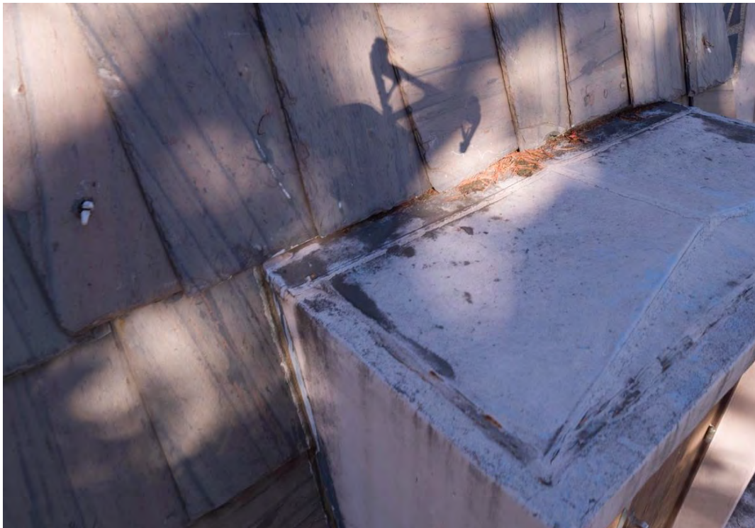
Figure 26 (below): Conditions at entry canopy (SW). Photo by Propellerheads.
