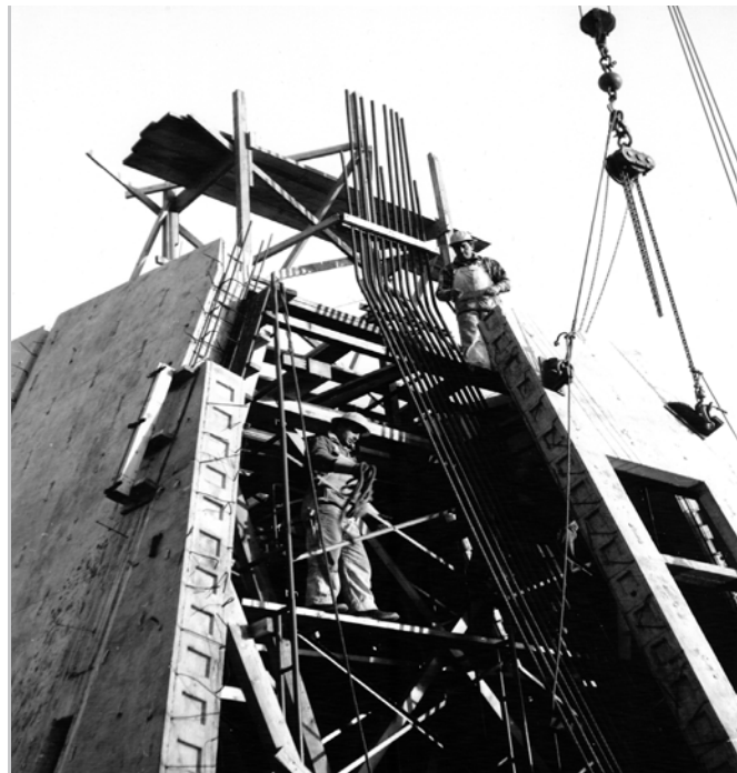
Figure A6. Installation of large pre-cast panels at the west elevation showing the shallow voids at the returns of the panels into which the cast-in-place concrete framework keyed. Courtesy of the DeLuca Construction Company archives.
