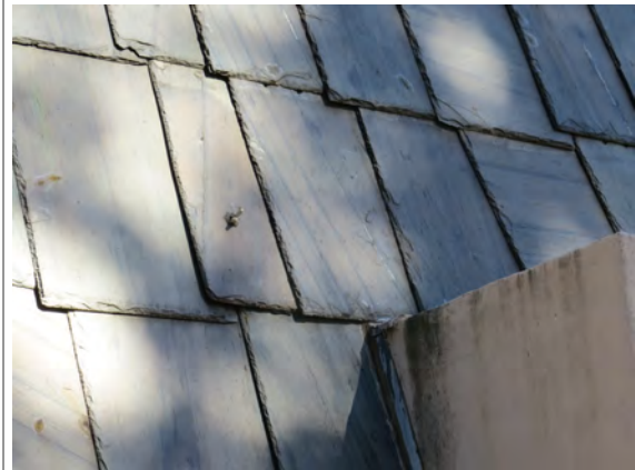
The 2005 water infiltration report noted that the fixtures in this location were water logged. They appear to have been subsequently removed.
