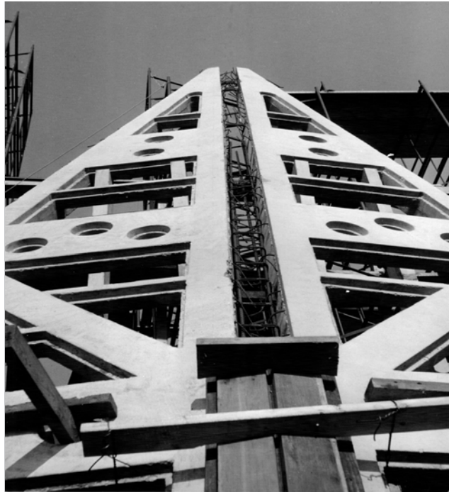
Figure A5. View of rebar installed between the pre-cast panels. Formwork used to construct the cast-in-place concrete rib between the pre-cast panels is visible at the bottom of the image. Courtesy of the DeLuca Construction Company archives.
