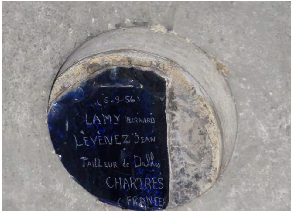
Figure A1. Dalle de verre panel installed in portal window near the base of pre-cast panel N7 (See Figure B2 for pre-cast panel location). Glass inscribed by a stained glass artist at Loire's studio in Chartres and dated 1956.
