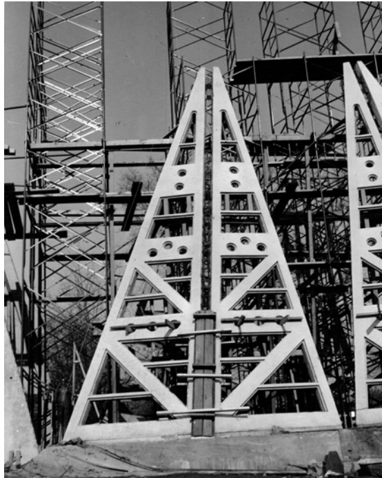
Figure A7. Formwork used to construct the cast-in-place concrete rib is visible between the pre-cast panels at the bottom of the triangular panels. The concrete ribs were poured in lifts using 6-8 foot long forms. Courtesy of the DeLuca Construction Company archives.
