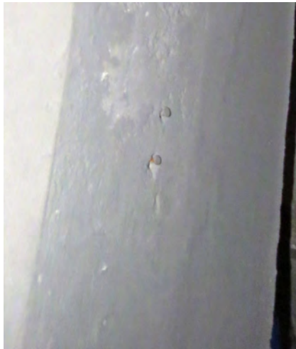
Isolated abandoned anchors in concrete.
