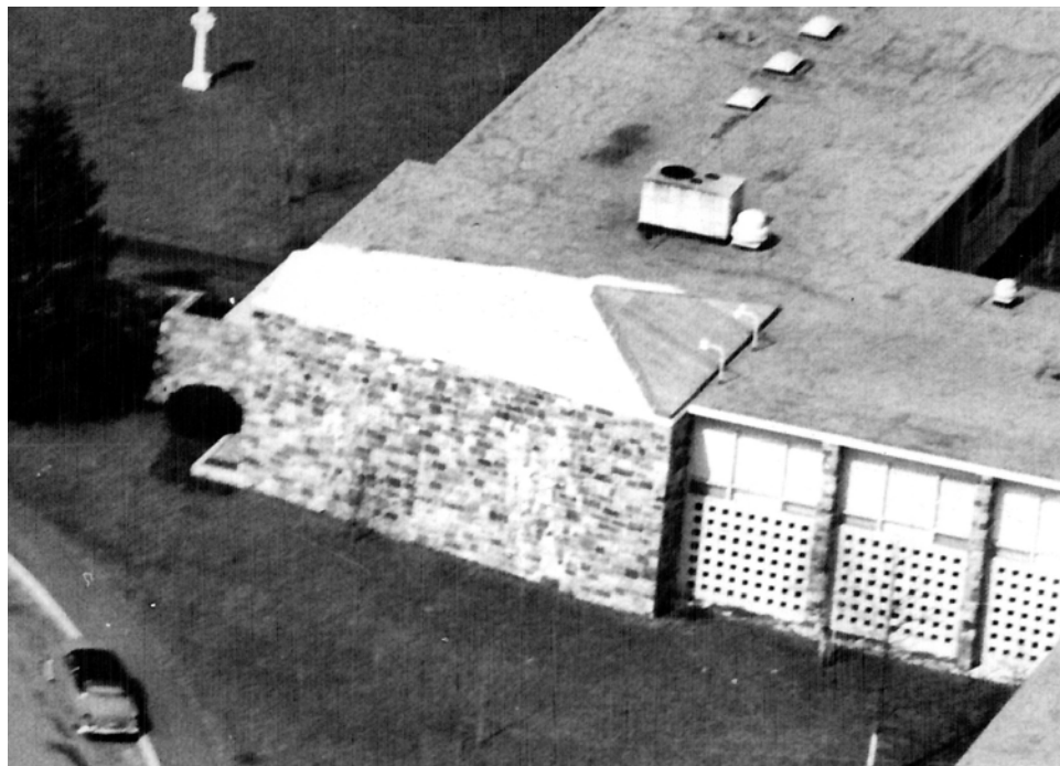
Figure A16. Detail of archival image showing the Chapel roof in 1966. The enclosure over the dalle de verre appears similar to the existing materials (See Figure A17). Note the two light fixtures to the right of the Chapel roof, which back light the skylight. Courtesy of the DeLuca Construction Company archives.
