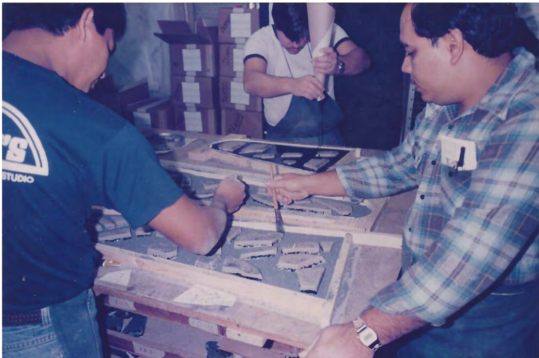
Figure 33 (below): Replicating dalle de verre panels at Rohlf's Studio. Source: Rohlf Archive.
