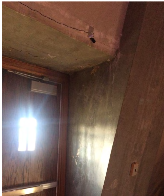
Figure 13 (below): Entrance at the south interior elevation. Photo by Prudon & Partners.
