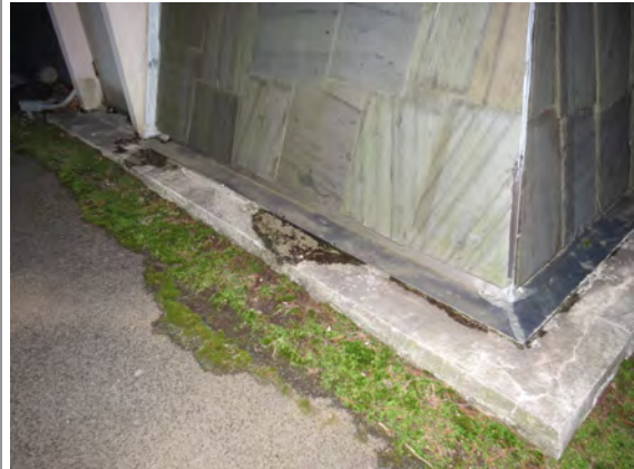
Grass adjacent to concrete base at the northwest corner of the Sanctuary.
