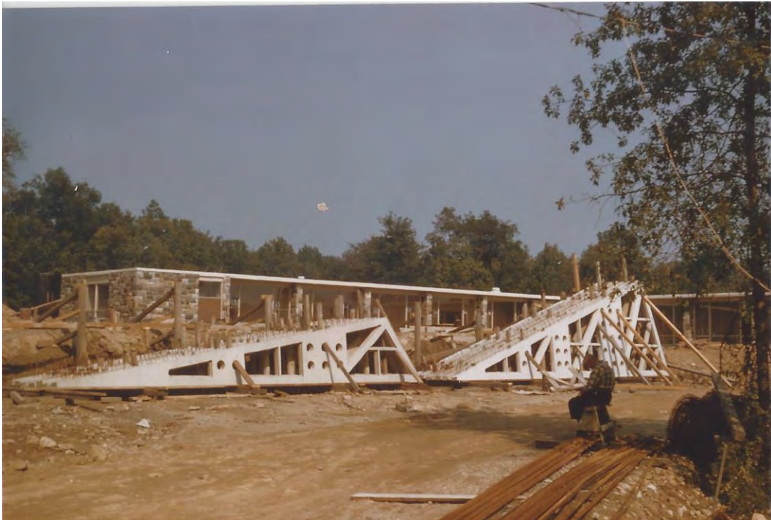
Figure 36 (below): Delivery of precast panels onsite, November 1956. Source: FPC Archive.
