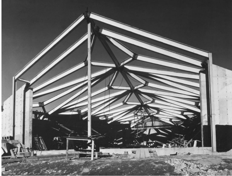
Figure 8 (above): The Parish Unit's Fellowship Hall construction framework. Source: FPC Archives.
