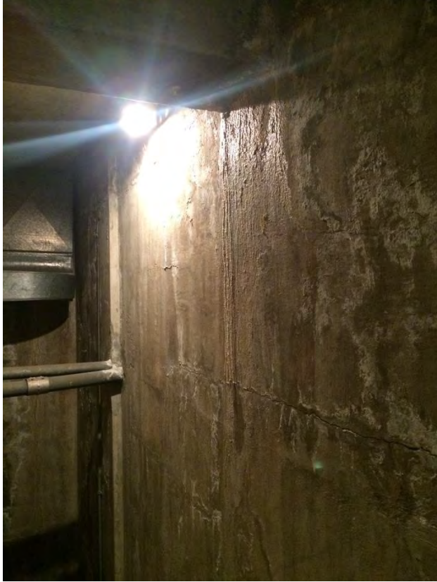
Figure 20 (above left): Conditions at foundation wall. Photo by Prudon & Partners.
