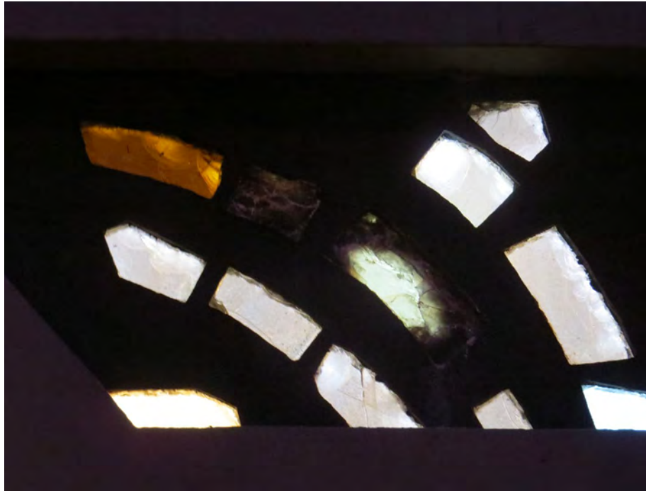
Figure A29. Typical darkened interior appearance of deteriorated glass on the south elevation due to biological growth and dirt deposition between layers of delaminating glass. Similar glass deterioration is visible on the north and east elevations.
