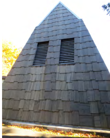
Typical soil and biological growth on slate.
