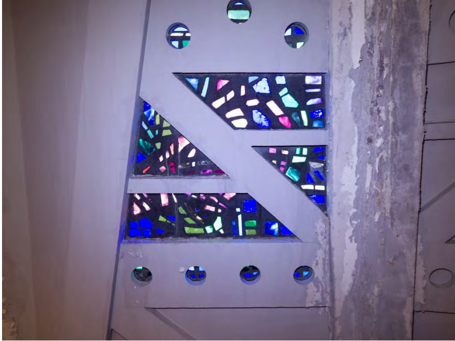
Above: Interior image of the east elevation (narthex), panels E5 and E6, showing condition of the replacement dalle de verre in epoxy matrix and condition of the poured-in-place concrete. Photo by Propellerheads, November 2016.
