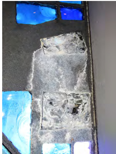
Heavy efflorescence on the glass and epoxy dalle de verre at the base of pre-cast panel S15.
