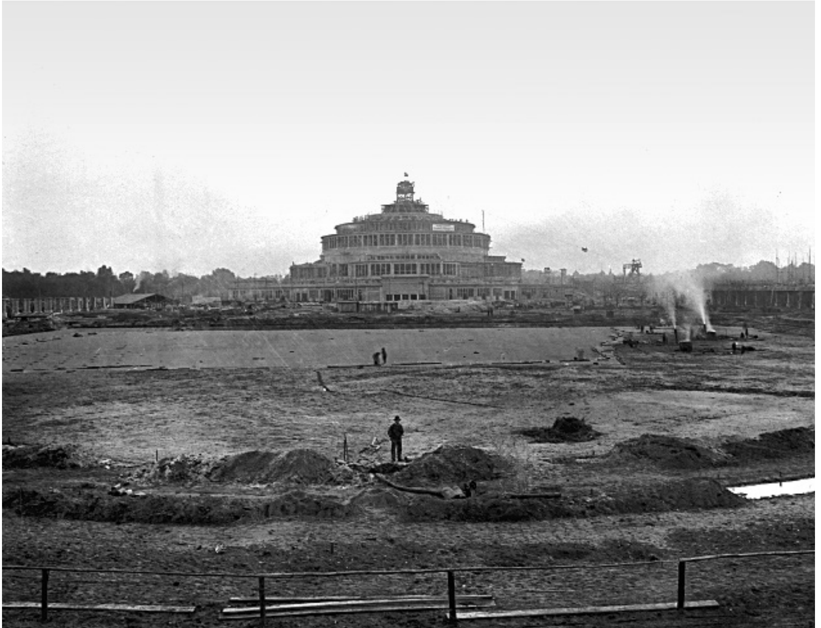
30 Centennial Hall, concrete shell, 1912/1913. Leibniz Institute for Research on Society and Space in Erkner near Berlin
