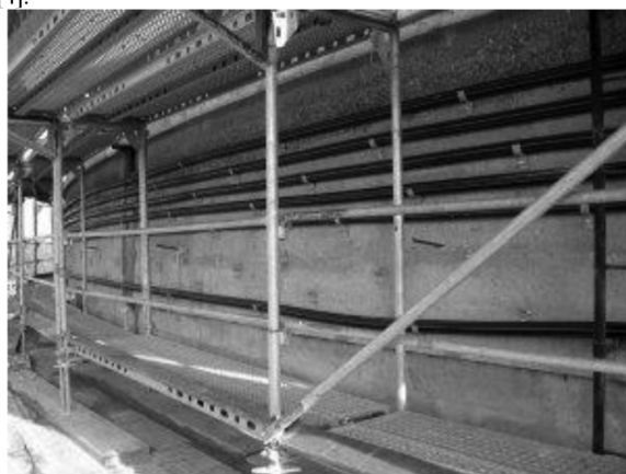
Fig. 2.14. Strengthening of the bottom tension ring –laying cables, [1].
