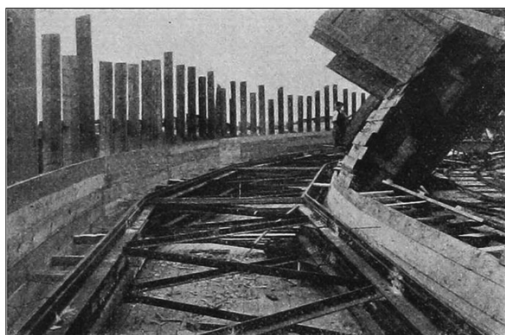
Fig. 3.75. Lattice structures which carry the tensile loads – archive photo
