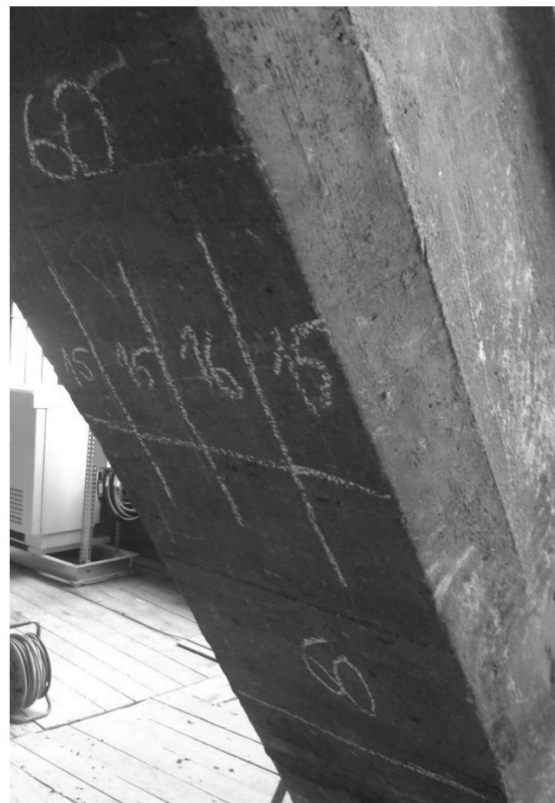
Fig.3.62. Spacing of the main reinforcing bars crosswise.
