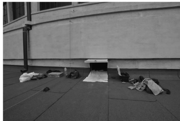
Fig. 3.78. One of the hatchways allowing access to the bearings.
