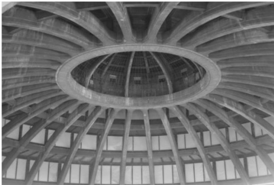
Fig. 2.2. The ribbed structure of the dome of the Centennial Hall.
