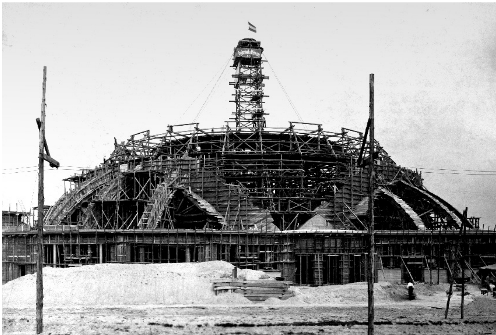
27 Centennial Hall, foyer construction, ca. September 1912. Museum of Architecture in Wrocław
