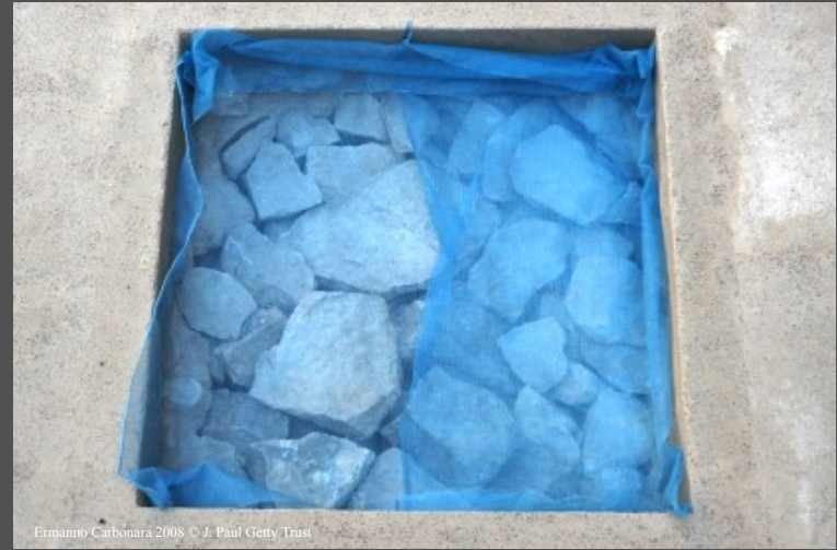
2 – separation membrane
