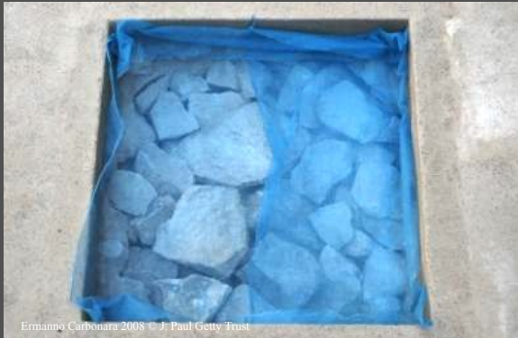
2 – separation membrane
