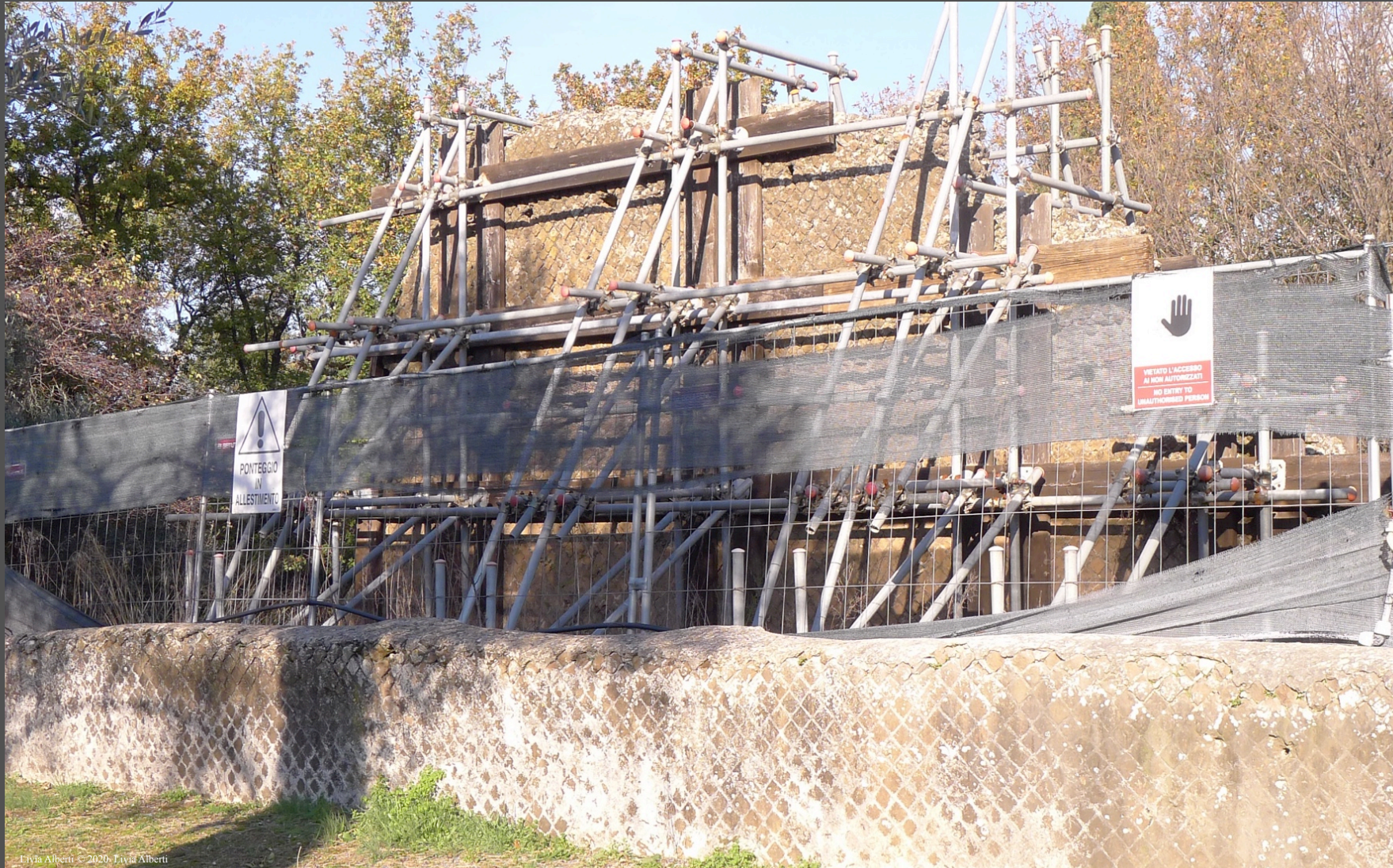
Temporary metal structure buttress
