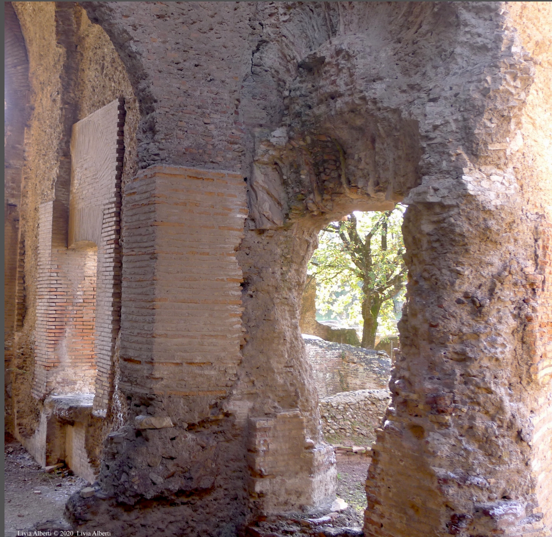
Reinforcement with masonry
