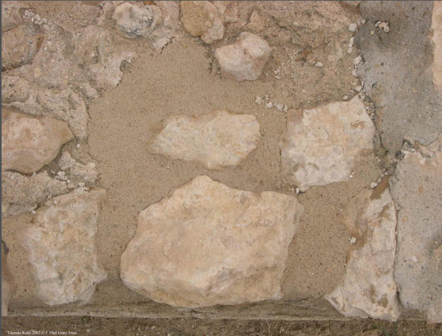
In-filling of lacunae with stones and mortar
