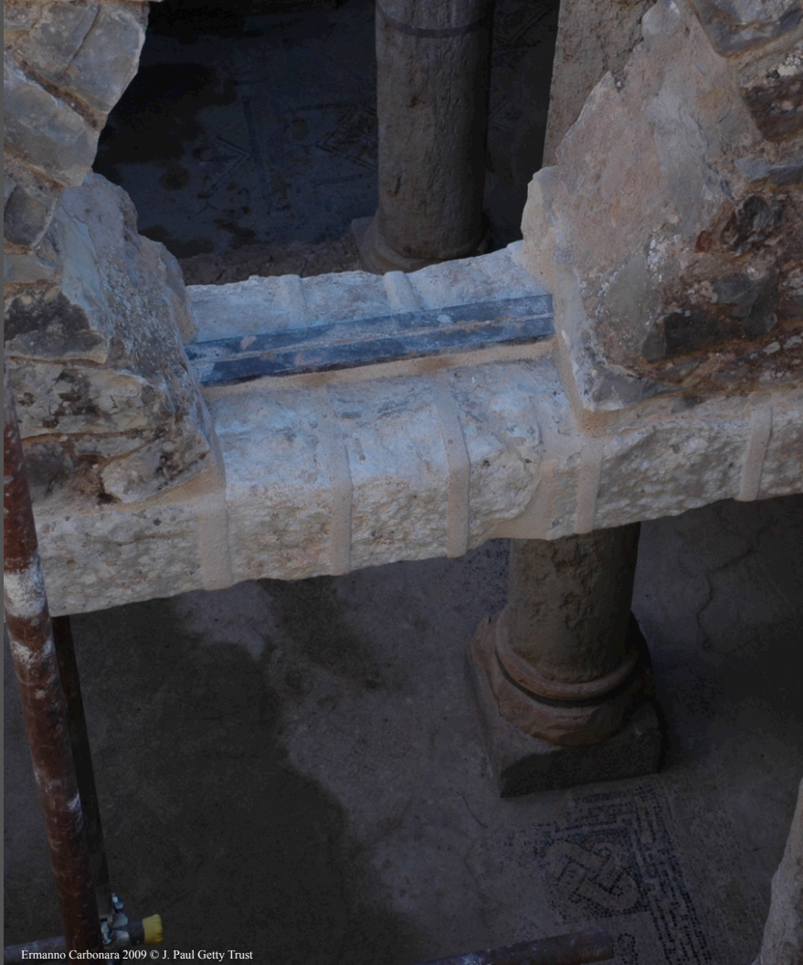
Reinforcement with metal elements
