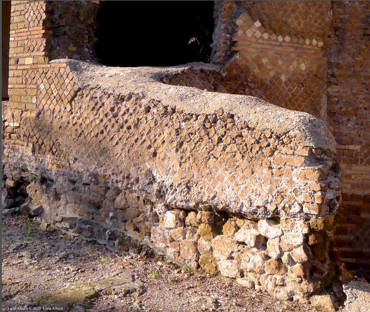
Wall capping using a layer of mortar
