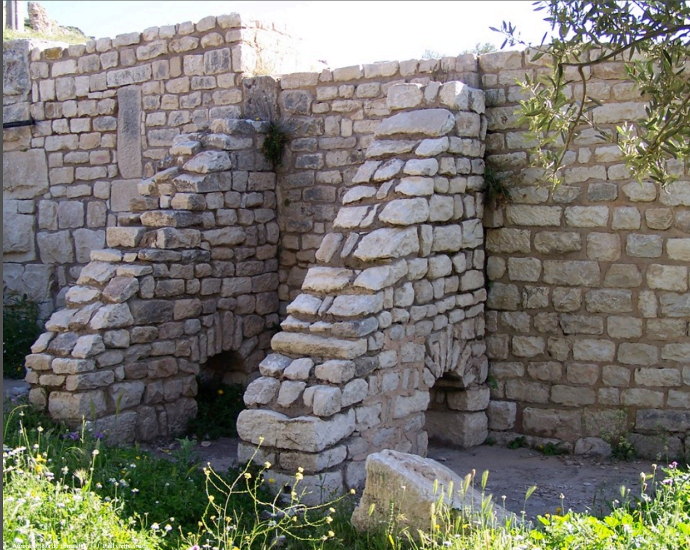
Masonry buttress
