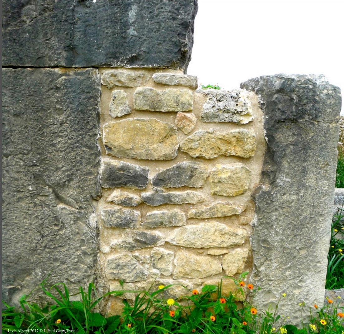
In-filling of masonry joints with mortar
