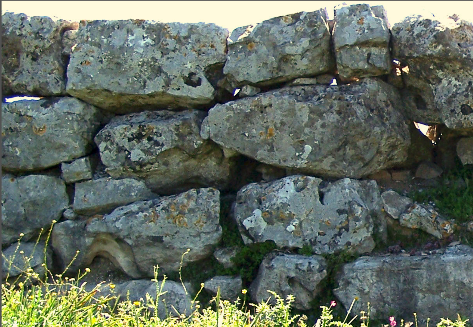
Dry wall construction No binder present.
