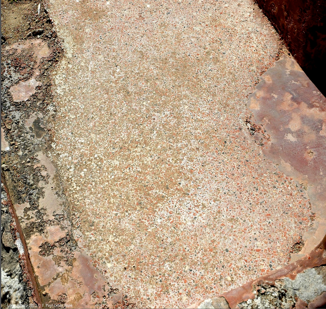
Cocciopesto - mortar with ceramic fragments
