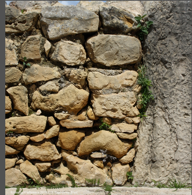
Loss of mortar of the construction
