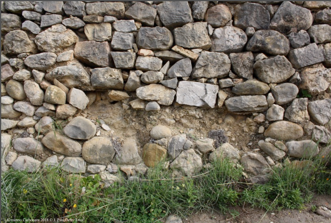
Loss of stones of the construction
