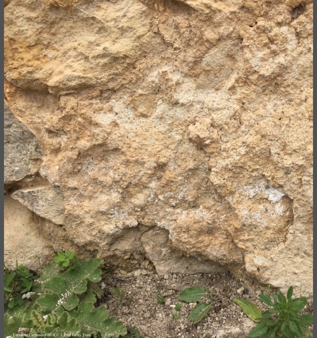
Deteriorated mortar of the construction and decorative surface
