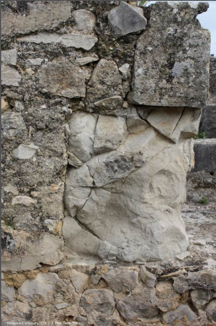
Deteriorated elements of the construction (stones and bricks)
