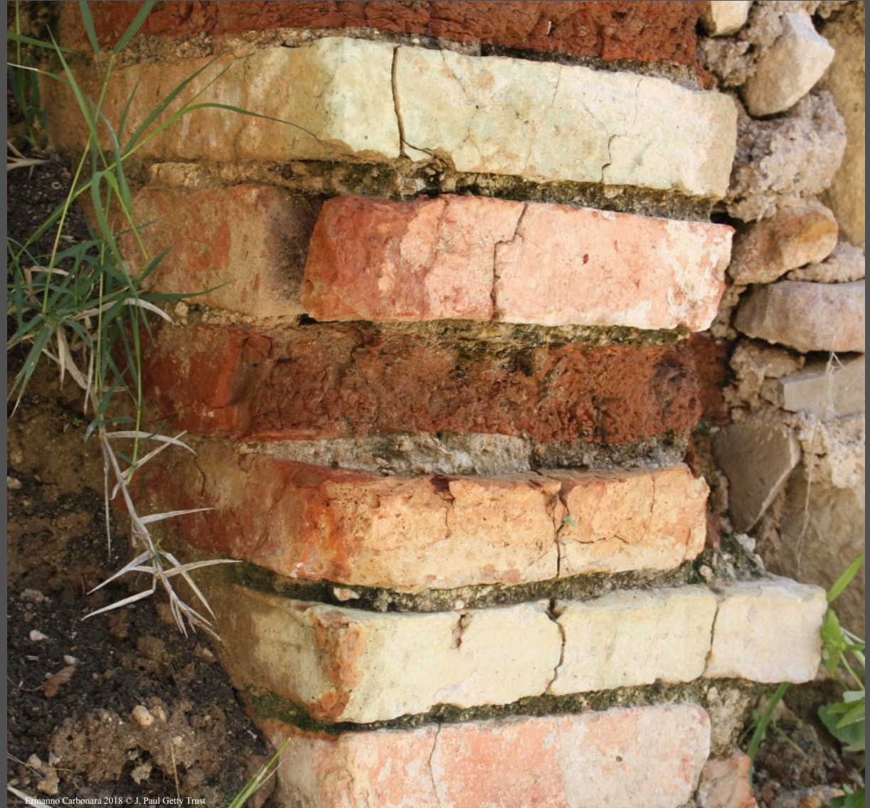
Deteriorated elements of the construction (stones and bricks)
