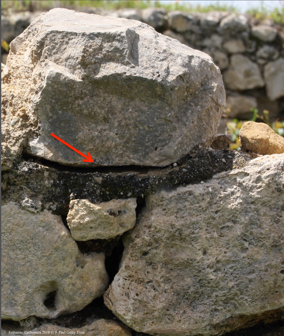
Detachment of elements of the construction
