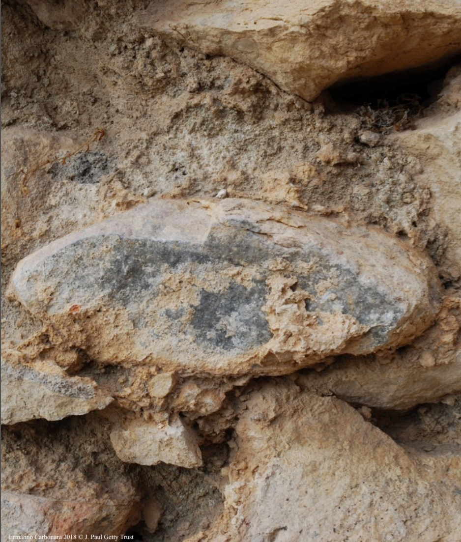
Deteriorated mortar of the construction and decorative surface
