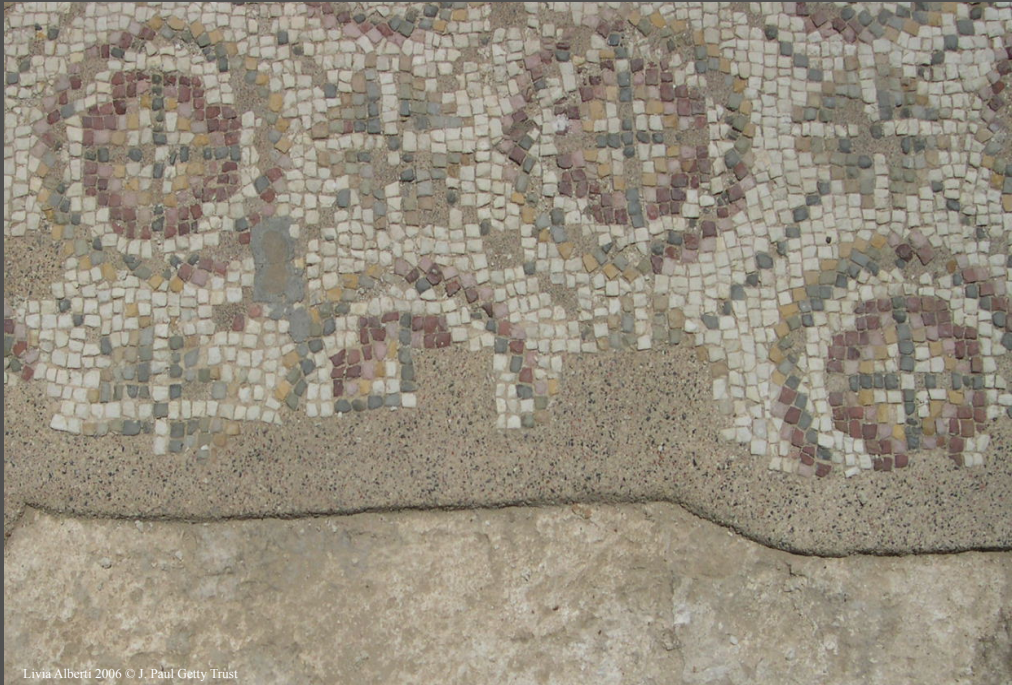
Mosaic edges protected with mortar
