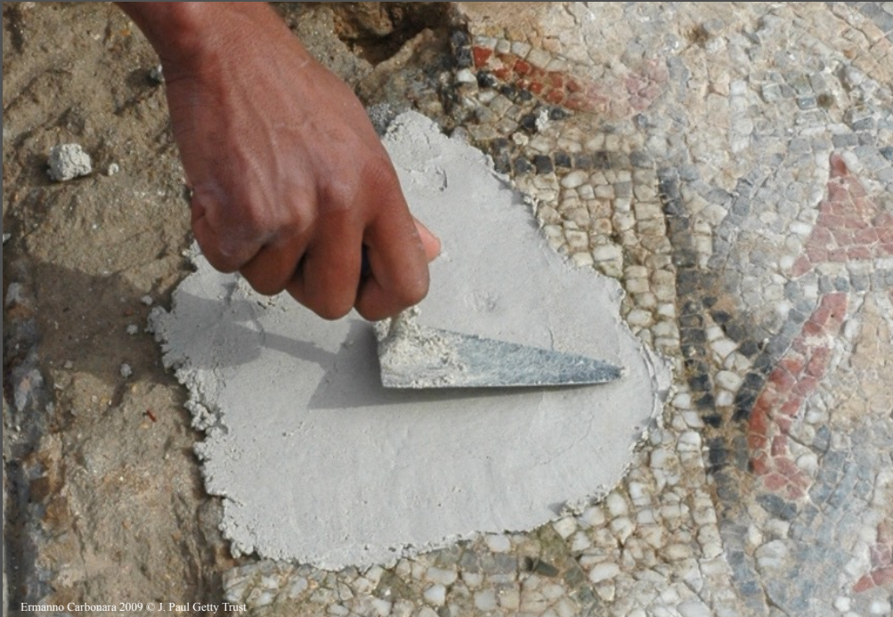
Application of surface layer of mortar
