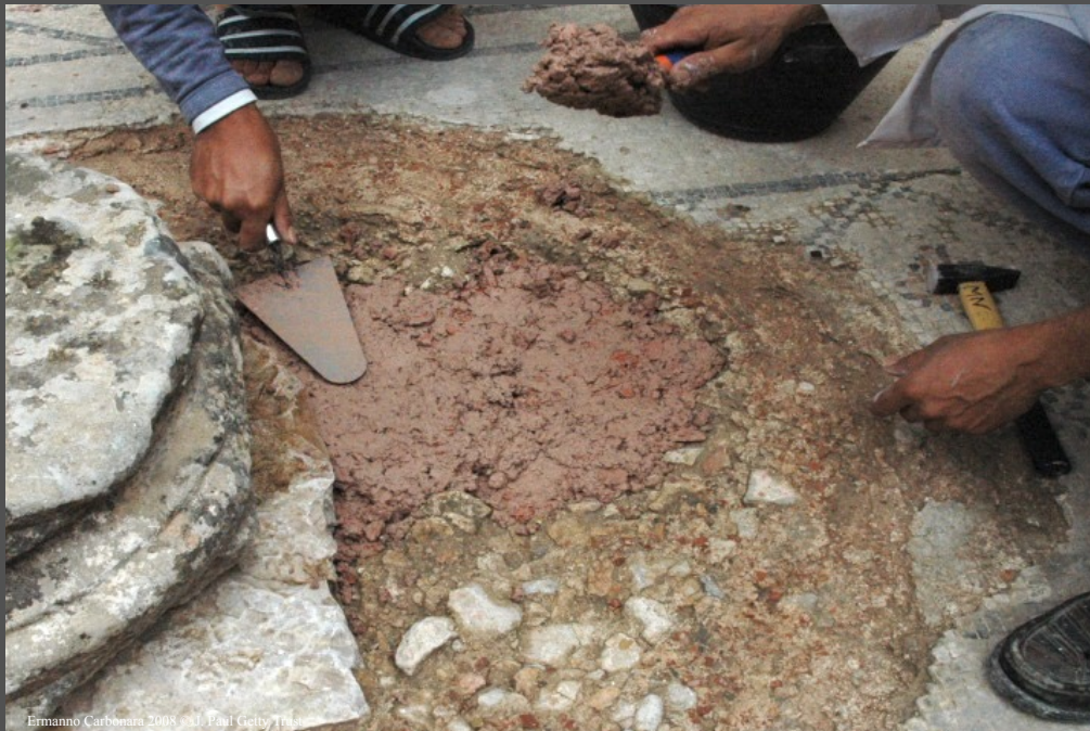
Applying the first layer of mortar
