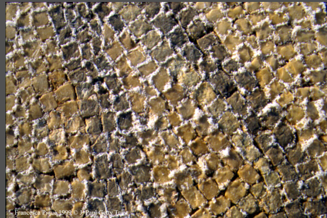
Efflorescence
