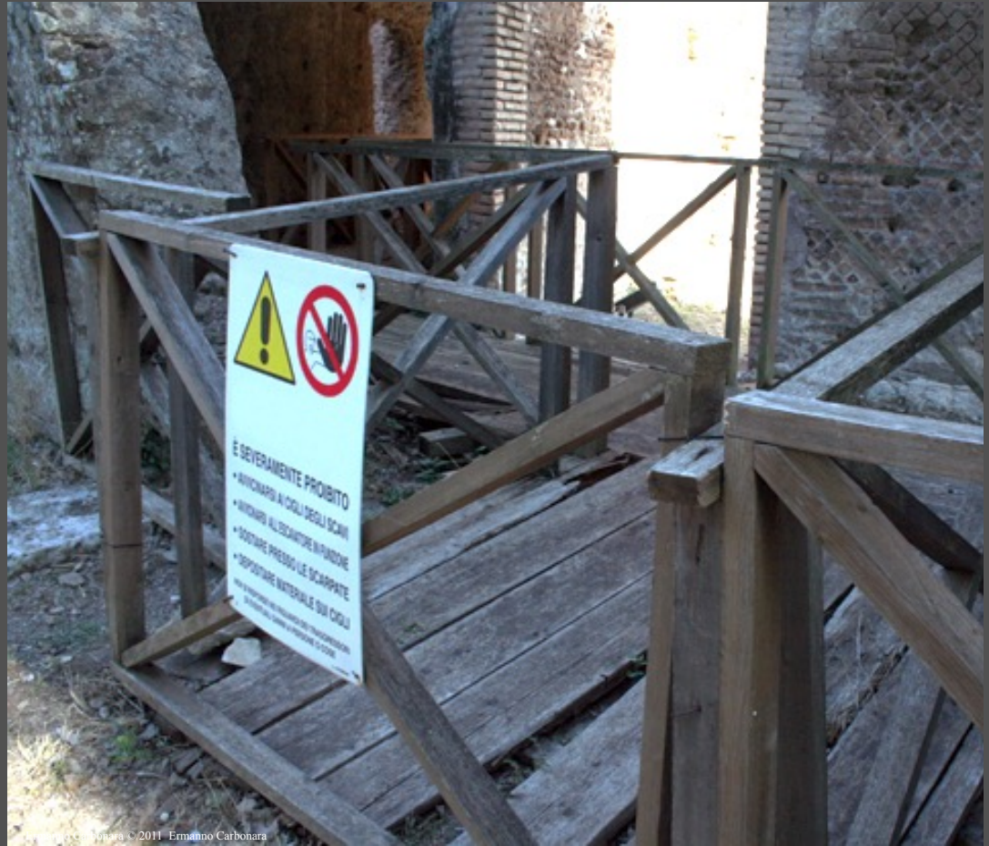
Damaged footbridge
