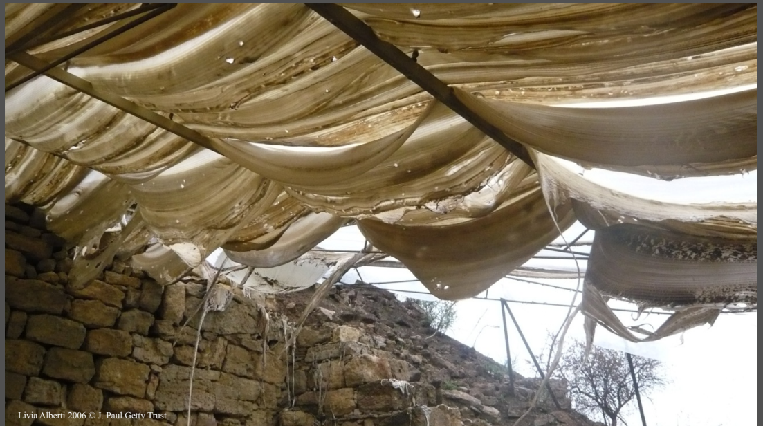
Deteriorated cover or shelter
