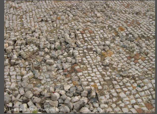
Bulges, Detachments, Cracks, Lacunae, Detached Tesserae
