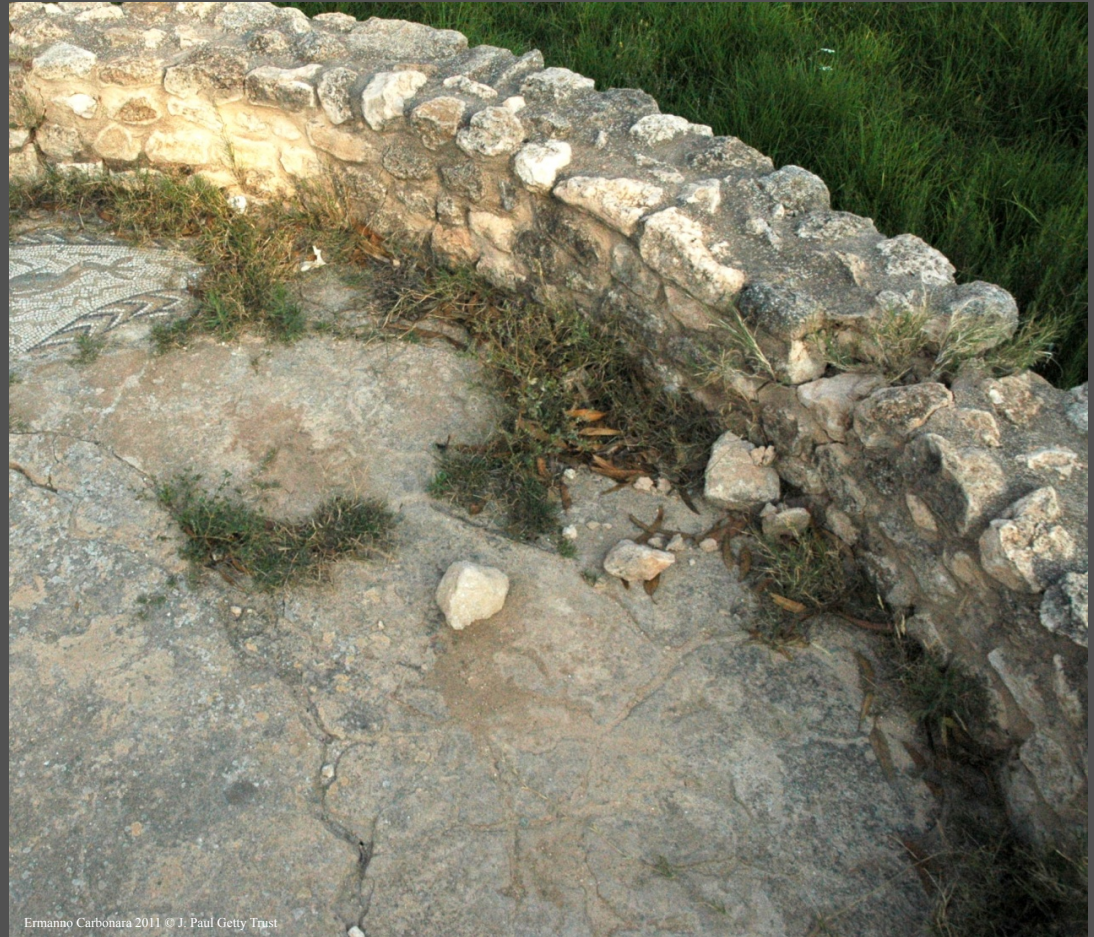
Stabilized walls with new deterioration
