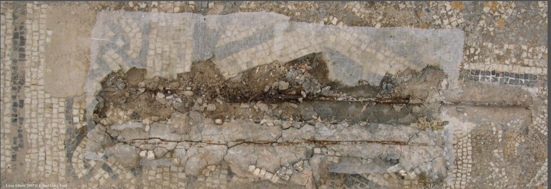
Temporary removal of the section of tessellatum located above the corroded bar
