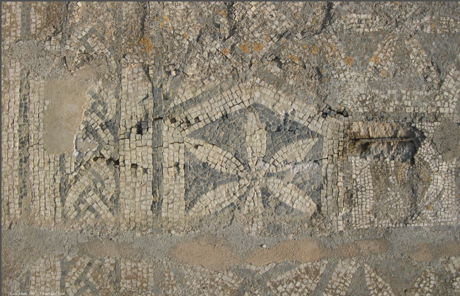
Complete cleaning of the area of the mosaic panel affected by corrosion of rebar
