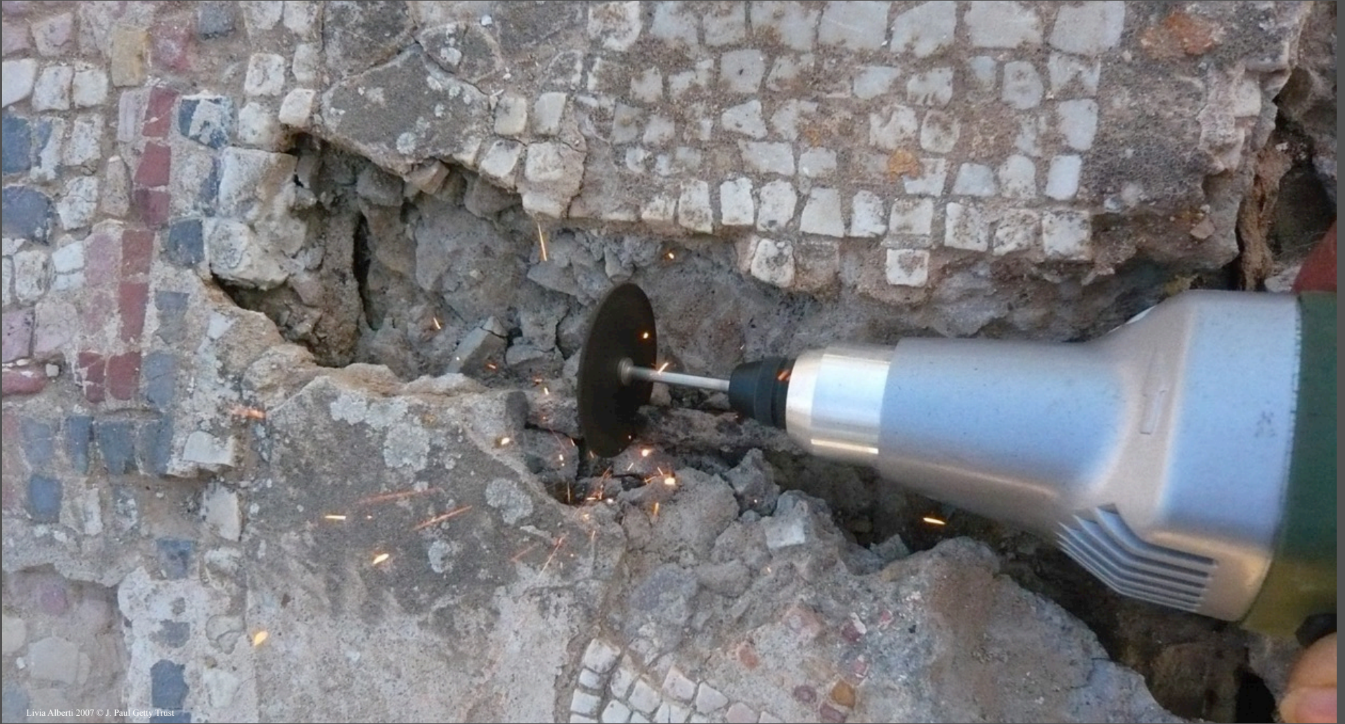
Cutting the steel bar
