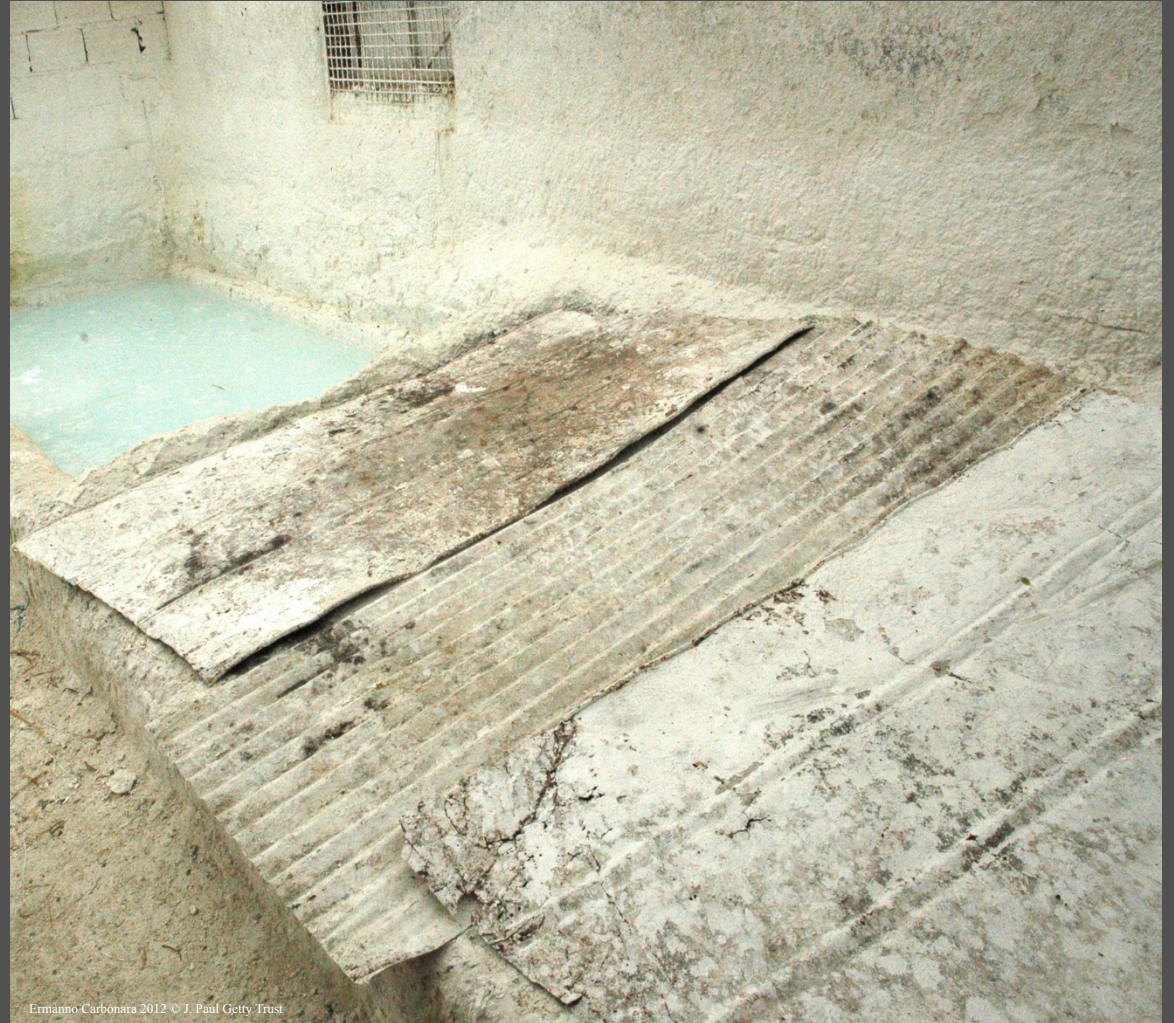
Basin for slaking and aging the lime putty
