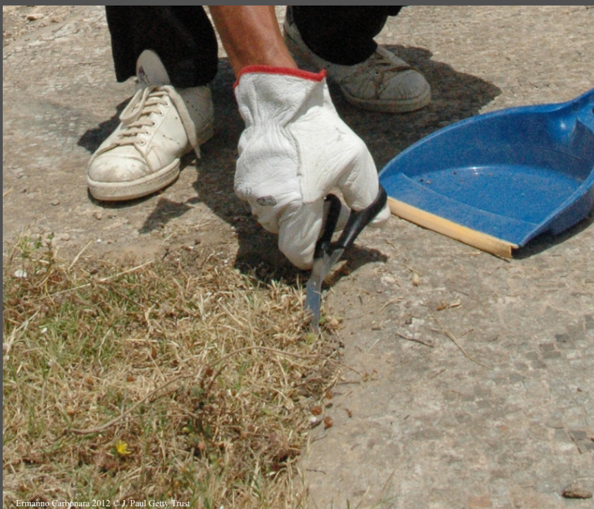
Removal of soil and vegetation with scissors
