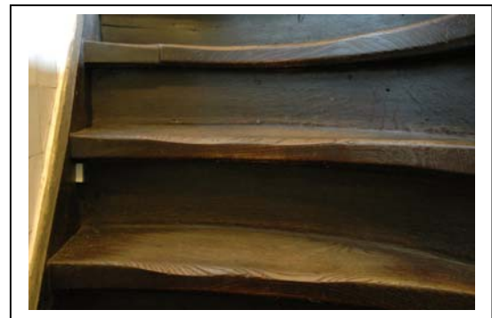
Detail of wear and tear on the steps.
