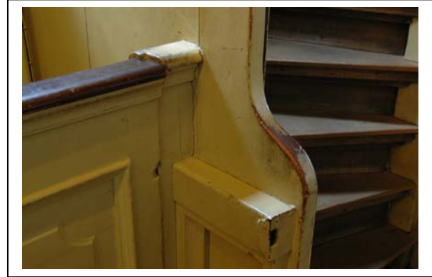
Detail of abrasion of posts of the stairs in the church
