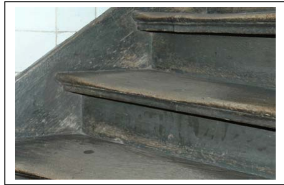
Detail of wear and tear on one of the steps. (photos: Paul Ryan)
