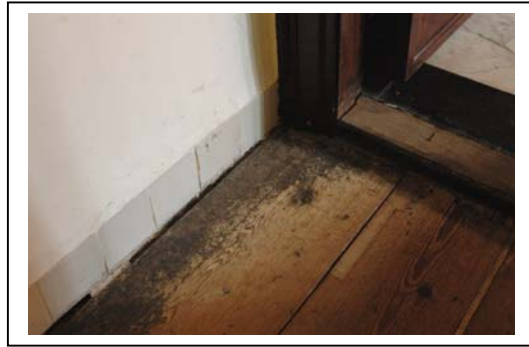
Floorboards showing shrinkage in width Darker area around edge of floor (photos: Paul Ryan)
