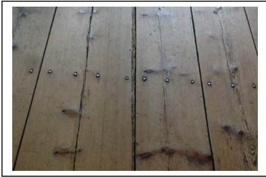
Floorboards showing shrinkage in width Darker area around edge of floor (photos: Paul Ryan)
