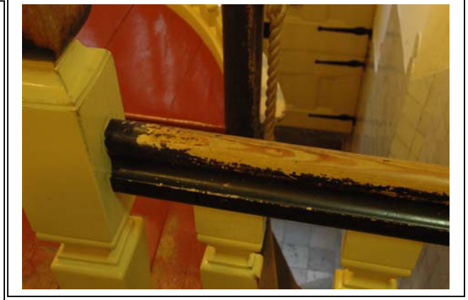
Damage to railing of balustrade on top of the stairs
