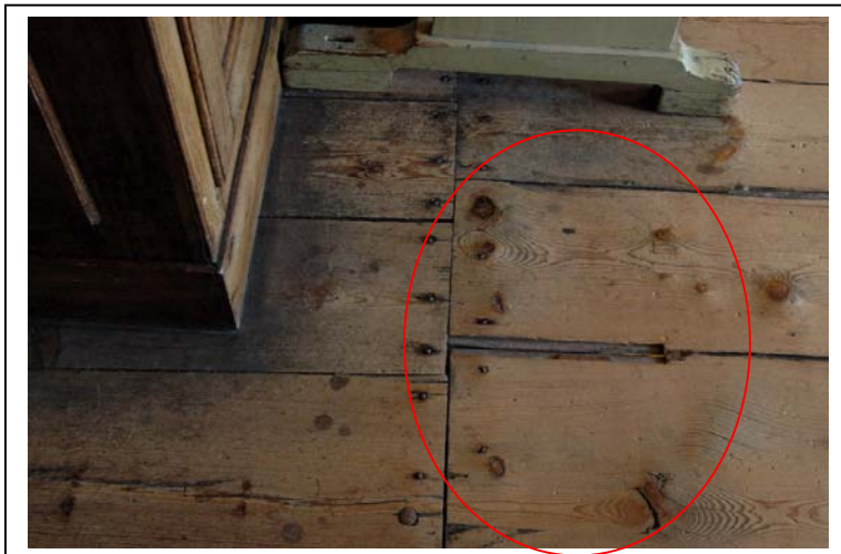
Area next to the organ that is more abraded. Loss of spring. (photo: Paul Ryan)
