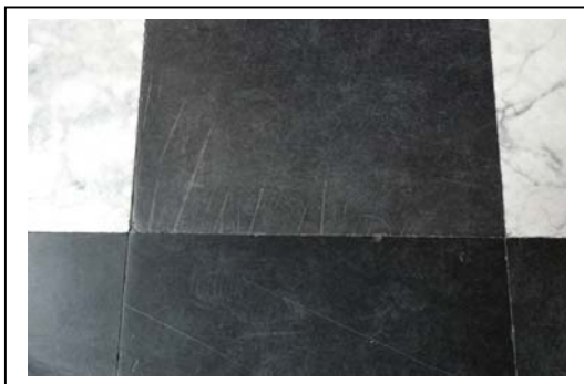
Details of damage to the Sael floor (scratching; chipping). NB: right photo shows white vein in black tile, easily mistaken for fracture . (photos: Paul Ryan)
