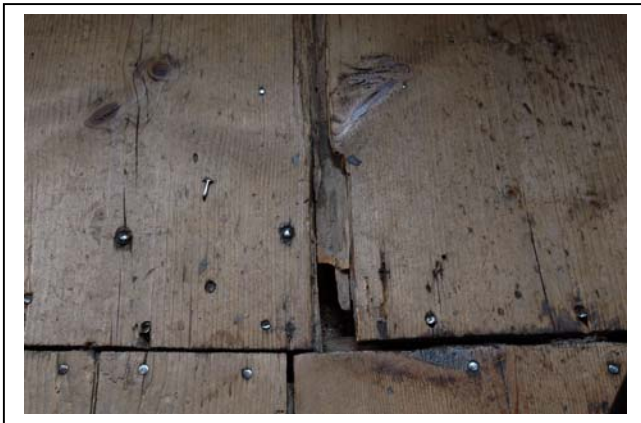
Details showing an exposed spring and related wood chipping (photos: Paul Ryan)
