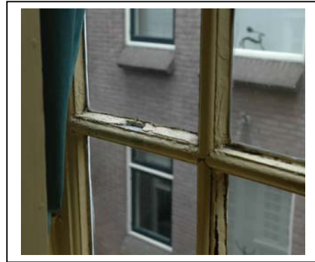
Damage to window sills, accelerated by condensation (photo: Paul Ryan)
