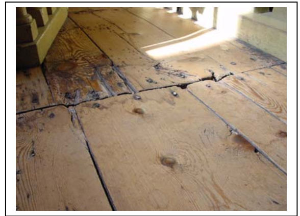
Details showing an exposed spring and related wood chipping (photos: Paul Ryan)
