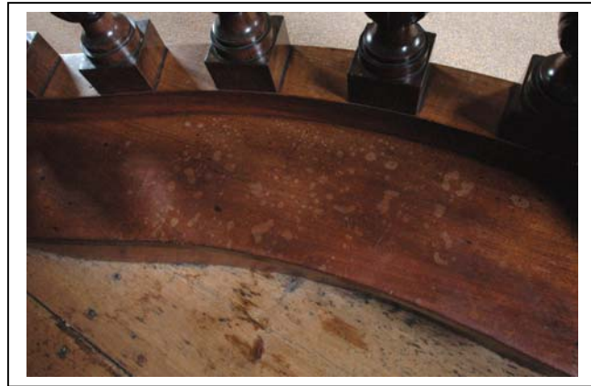
Detail of the water stains caused during baptism.
