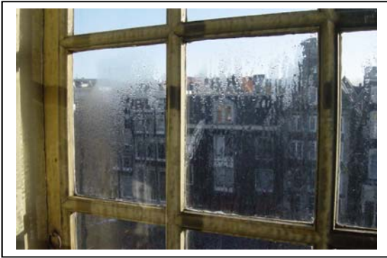
Condensation on the inside of window in the church (photo: TU/E)
