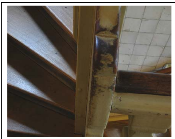
Detail of railing (photos: Paul Ryan)
