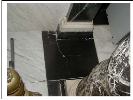
Details of damage to the Sael floor (deformation; cracking due to structural pressure of chimney piece). (photos: Paul Ryan)
