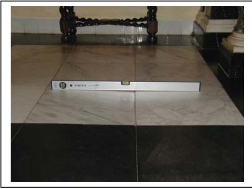
Details of damage to the Sael floor (deformation; cracking due to structural pressure of chimney piece). (photos: Paul Ryan)
