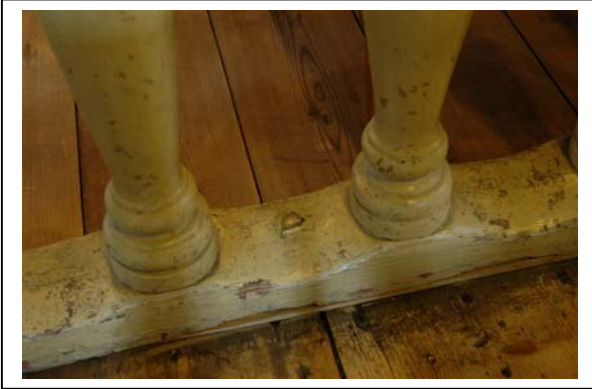
Detail of severe abrasion of the balustrade, caused during the time this was still a church (photos: Paul Ryan)
