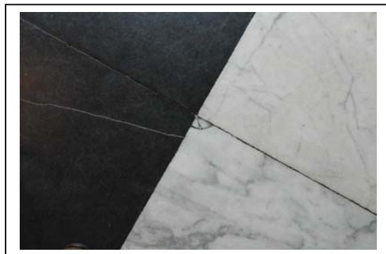
Details of damage to the Sael floor (scratching; chipping). NB: right photo shows white vein in black tile, easily mistaken for fracture . (photos: Paul Ryan)
