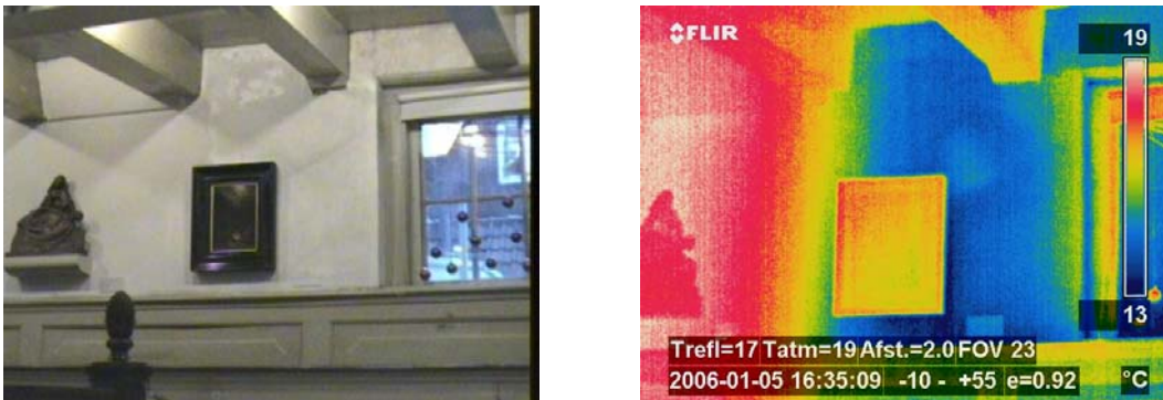
The south west wall in Church, partly and outer wall and inner wall (photos: TU/E)
