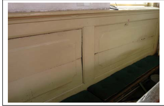
Detail of the dislodged back
