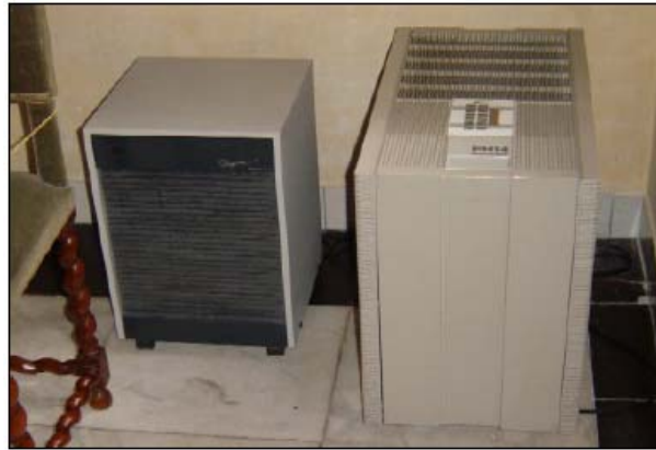
Fig. 12 Humidifier and dehumidifier in the Sael.
