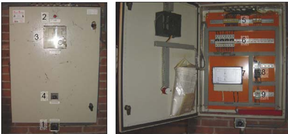
Fig. 10 Switchboard cupboard for central heating boiler
