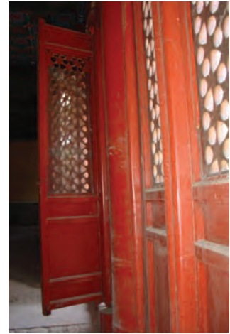
普仁寺重新油漆的门扇。 Restored architectural paint on the doors at Puren Temple.
