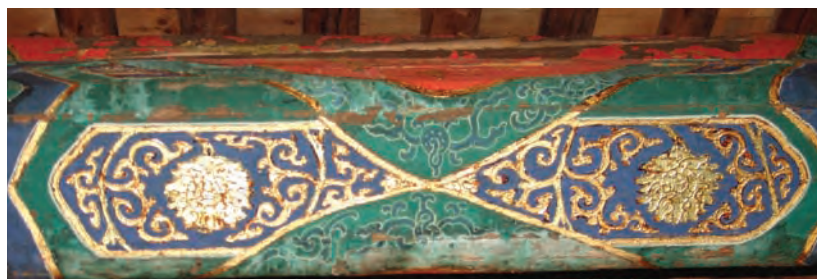
枋底的纹饰 Pattern on the underside of the ridge architrave.
