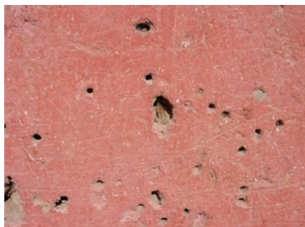
会乘殿，东立面 红色抹灰 凿及子弹造成的小坑 Huicheng Hall, E Facade Red- colored stucco Holes caused by gouging and projectiles
