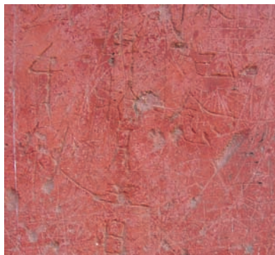
会乘殿，西立面 红色抹灰 涂写及凿痕 Huicheng Hall, W Facade Red-colored stucco Graffiti and gouging
