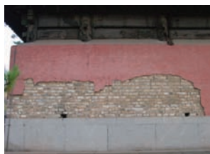
会乘殿，西立面，北端 红色抹灰 脱落区域 Huicheng Hall, W Facade, N end Red-colored stucco Area of loss
