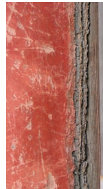
会乘殿，南立面，西端 红色抹灰 凿痕及划痕 Huicheng Hall, S Facade, W end Red-colored stucco Gouges and scratches
