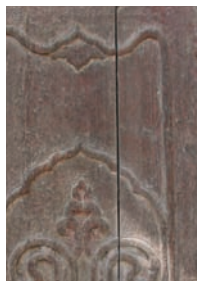
会乘殿，南立面 隔扇门 劈裂 Huicheng Hall, S Facade Door baffleboard Split
