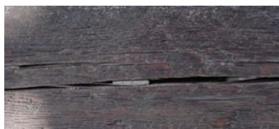
会乘殿，南立面 大额枋 裂缝中有地仗填充物 Huicheng Hall, S Facade Architrave Crack with original plaster infill
