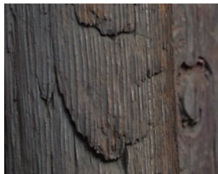
会乘殿，南立面 柱 片状开裂及腐朽 Huicheng Hall, S Facade Column Splintering and ero- sion
