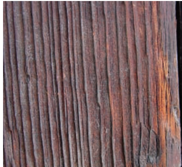
会乘殿，南立面 纹理凸起 Huicheng Hall, S Facade Raised Grain
