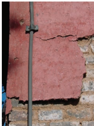
会乘殿，西立面 红色抹灰 空鼓与附近的裂缝 及脱落 Huicheng Hall, W Facade Red-colored stucco Detachment with adjacent cracking and loss
