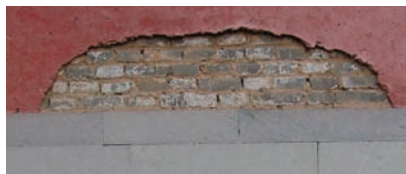
会乘殿，西立面，南端 红色抹灰 脱落区域 Huicheng Hall, W Facade, S end Red-colored stucco Area of loss
