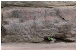
会乘殿，南侧台阶 红砂岩 外表侵蚀 Huicheng Hall, S Stair, riser Red Sandstone Surface erosion
