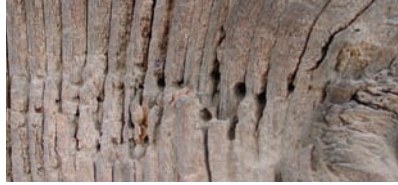
会乘殿，南立面 柱 虫蛀洞（与腐朽） Huicheng Hall, S Facade Column Exit holes of insects (and erosion)
