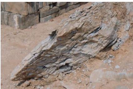
清凉楼 鸚鵡岩 粉碎的石墙 Qingliang Building Tuff ( yingwuyan ) Fissuring wall
