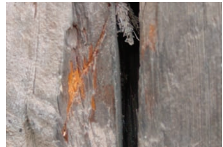
会乘殿，北立面 抱框及门扇 凿口痕迹及蚀洞 Huicheng Hall, N Facade Enclosure frame and door Gouge marks and scoring
