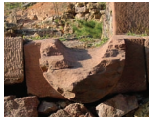
吐水嘴 红砂岩 边缘脱落及被侵蚀 Scupper Red Sandstone Eroded edges following loss
