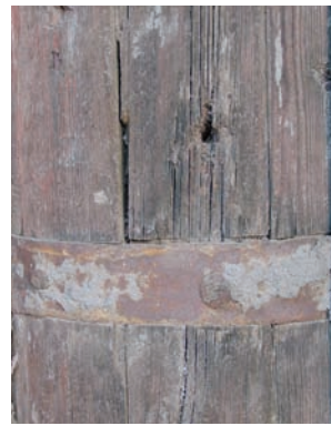
会乘殿，南立面 铁箍 退色 Huicheng Hall, S Facade Enclosure frame Greying
