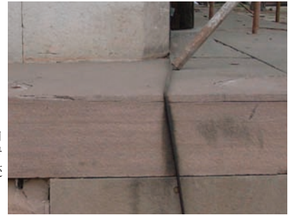
Huicheng Hall, W Facade, S corner of platform Red Sandstone Rusting of lightning rod resulting in staining
