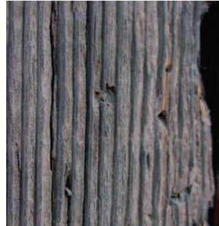
会乘殿，南立面 纹理凸起 Huicheng Hall, S Facade Raised Grain
