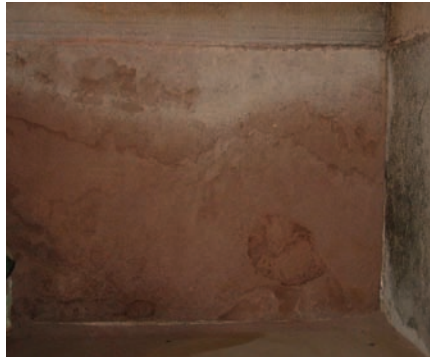
Shanmen, W Interior sill wall Red Sandstone Staining attributed to rising damp
