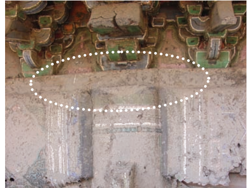
Huicheng Hall, E Facade, Lower Eave Flat tie beam Warping
