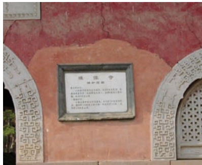
山门，南立面 红色抹灰 名牌周围不和谐 的重新抹灰 Shanmen, S Facade Red-colored stucco Incompatible replastering around new sign
