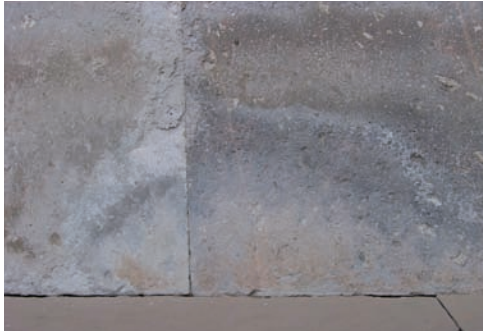
会乘殿，室外东北槛墙 鸚鵡岩 盐霜凝结 Huicheng Hall, NE Exterior sill wall Tuff ( yingwuyan ) Salt efflorescence
