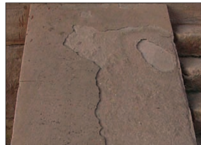
会乘殿，南侧台阶垂带石 红砂岩 起甲并剥落 Huicheng, S Stair splay Red Sandstone Scaling with loss
