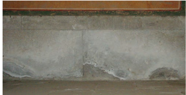
会乘殿，室内东北角槛墙 鸚鵡岩 盐霜凝结 Huicheng Hall, NE Interior sill wall Tuff ( yingwuyan ) Salt efflorescence
