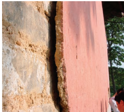
会乘殿，西立面 红色抹灰 从邻近的脱落部分看空鼓 Huicheng Hall, W Facade Red-colored stucco Detachment, as seen through adjacent loss
