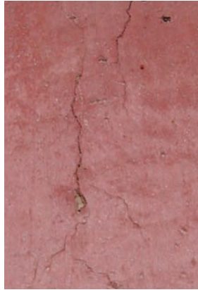
会乘殿，西立面 红色抹灰 开裂 Huicheng Hall, W Facade Red-colored stucco Cracking
