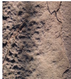
会乘殿，南侧台阶，细部 红砂岩 侵蚀及不均匀表面侵蚀 Huicheng Hall, S Stair, Tread Red Sandstone Differential erosion
