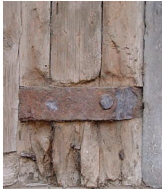
会乘殿，北立面 柱脚 腐朽 Huicheng Hall, N Facade Base of Column Erosion
