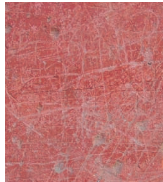
会乘殿，西立面 红色抹灰 涂写及凿痕 Huicheng Hall, W Facade Red-colored stucco Graffiti and gouging
