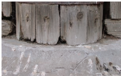
会乘殿，北立面 鸚鵡岩 鸟粪 Huicheng Hall, N Facade Tuff ( yingwuyan ) Bird droppings
