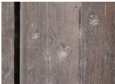
会乘殿，北立面 柱及门抱框 凿口痕迹及蚀洞 Huicheng Hall, N Facade Column and enclosure frame Gouge marks and scoring
