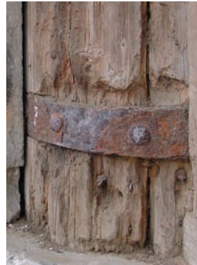
会乘殿，北立面 柱脚 腐朽 Huicheng Hall, N facade Base of Column Erosion
