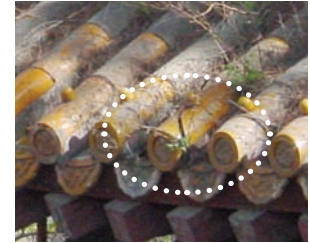
Huicheng Hall, N facade, W side Lower eave Glazed roof tiles Cracking and Breakage (in two areas)
