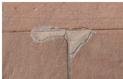
山门，南立面，墙 红砂岩条石 水泥填充 Shanmen, S Facade, sill wall Red Sandstone ashlar blocks Cement infill
