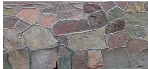
围墙，南立面 虎皮石墙 使用水泥做不和谐的重新勾缝 Perimeter Wall, S Facade Rubble "tiger skin" masonry Incompatible repointing with cement
