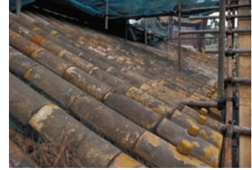
会乘殿，东立面 下檐 琉璃瓦 脱釉 Huicheng Hall, E facade Lower eave Glazed tile Loss of glaze
