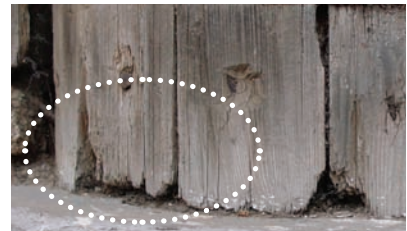
会乘殿，南立面 柱脚及其邻近的门 抱框 片状开裂及腐朽 Huicheng Hall, N Facade Base of column and adjacent door frame Splintering and erosion
