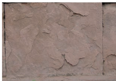
会乘殿，台基西台帮 红砂岩 起甲及剥落 Huicheng Hall, W Platform Red Sandstone Flaking and scaling
