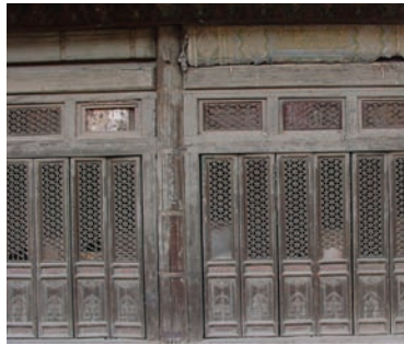
会乘殿，北立面 门、窗、枋 木质暴露 Huicheng Hall, N Facade Doors, windows, architrave Exposed wood
