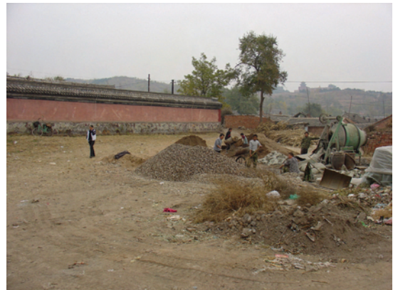
5. 殊像寺，南墙东边 修道路的器具与材料放置于庙地。 Shuxiang Temple, south wall, east side Equipment and materials for road construction adjacent to temple grounds
