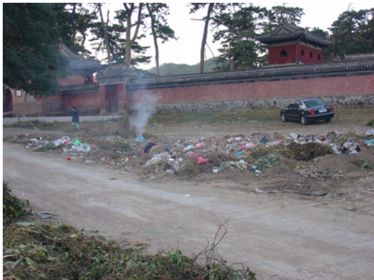
4. 殊像寺，南墙与山门 靠近围墙有新修的村道路与烧垃圾。 Shuxiang Temple, south wall and Shanmen New village road and trash burning adjacent to perimeter wall
