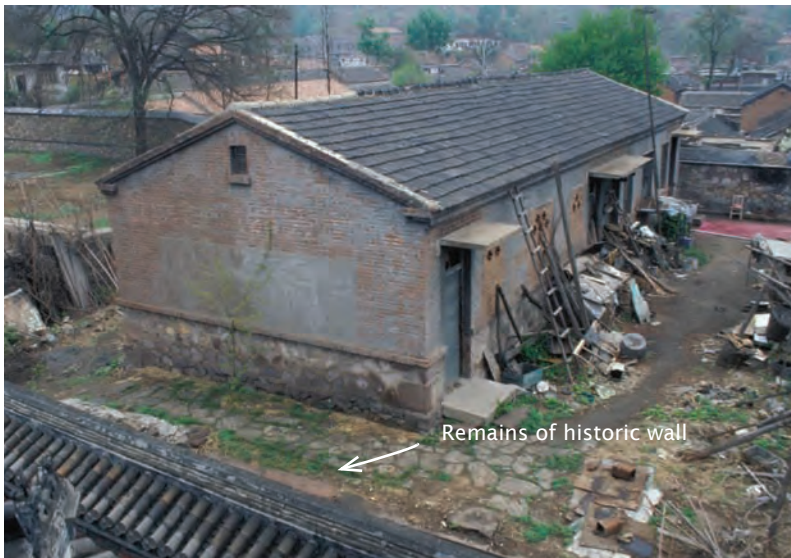
132. 文保所，前景为古墙基址 Custodian's building with remains of historic walls in foreground
