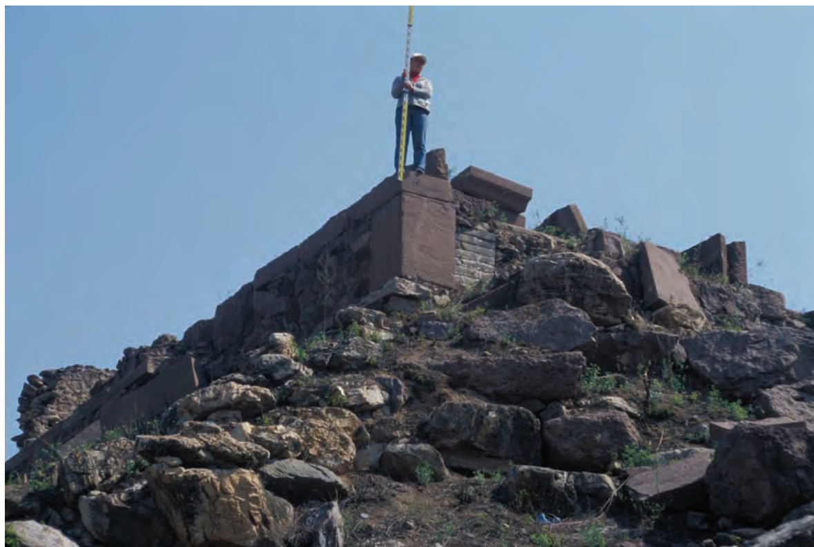
109. 慧喜殿西南角的南墙局部坍塌情景 SW corner of Huixi Hall showing partial collapse of south wall
