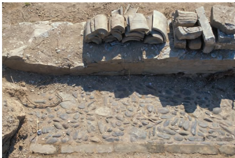
119. 建筑周围的卵石散水 Pebbled drip-line pavement surrounding buildings
