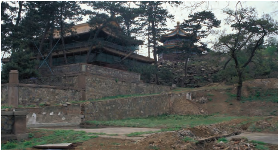
129. 2004年五号区内南北随墙，现在为机动车道的护坡墙 N-S running wall in center part of Area 5, now serving as a retaining wall for access road (2004)
