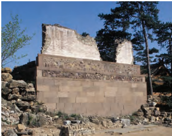
95. 雪净殿西侧陡峭的高台 Steep platform of the west side of Xuejing Hall
