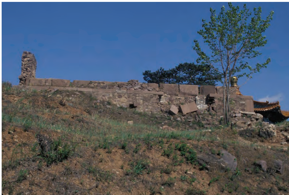
108. 慧喜殿西墙局部坍塌情景 Partially collapsing west wall of Huixi Hall
