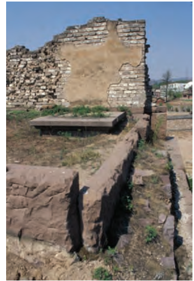
94. 槛墙、塑像底座、石砌墙 Sill wall, statue base, and masonry wall
