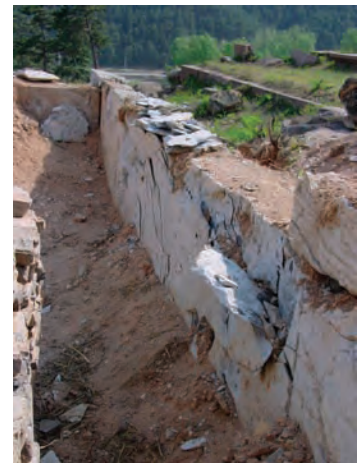
103. 鸚鵡岩檻牆石裂隙情景 Fragmentation of tuff sill walls
