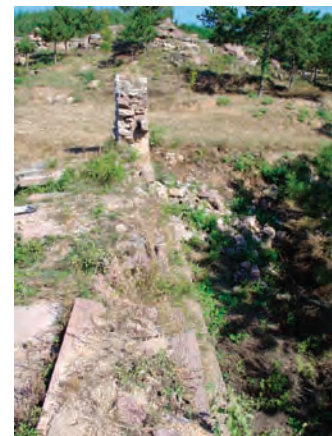
100. 东墙，朝北 Close-up of east wall, looking N
