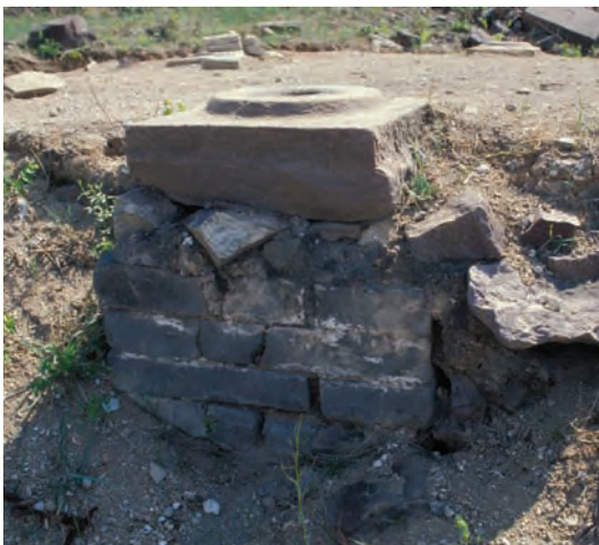
112. 柱顶石、礅墩 Brick support for column bases
