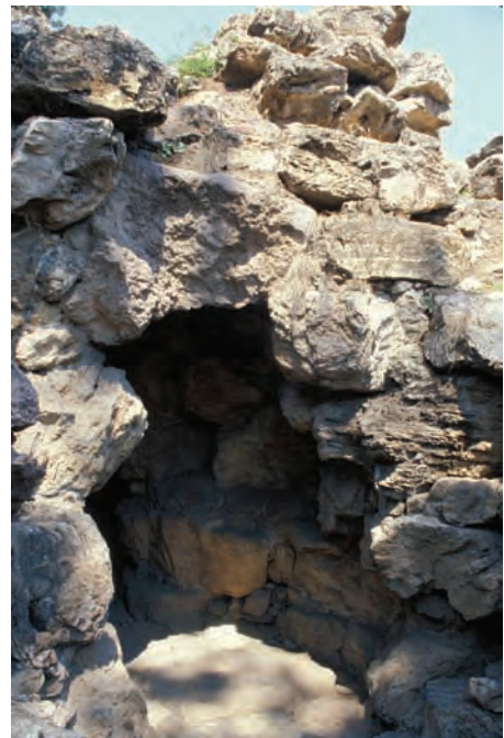
84. 假山涵洞 Tunnel through rockery
