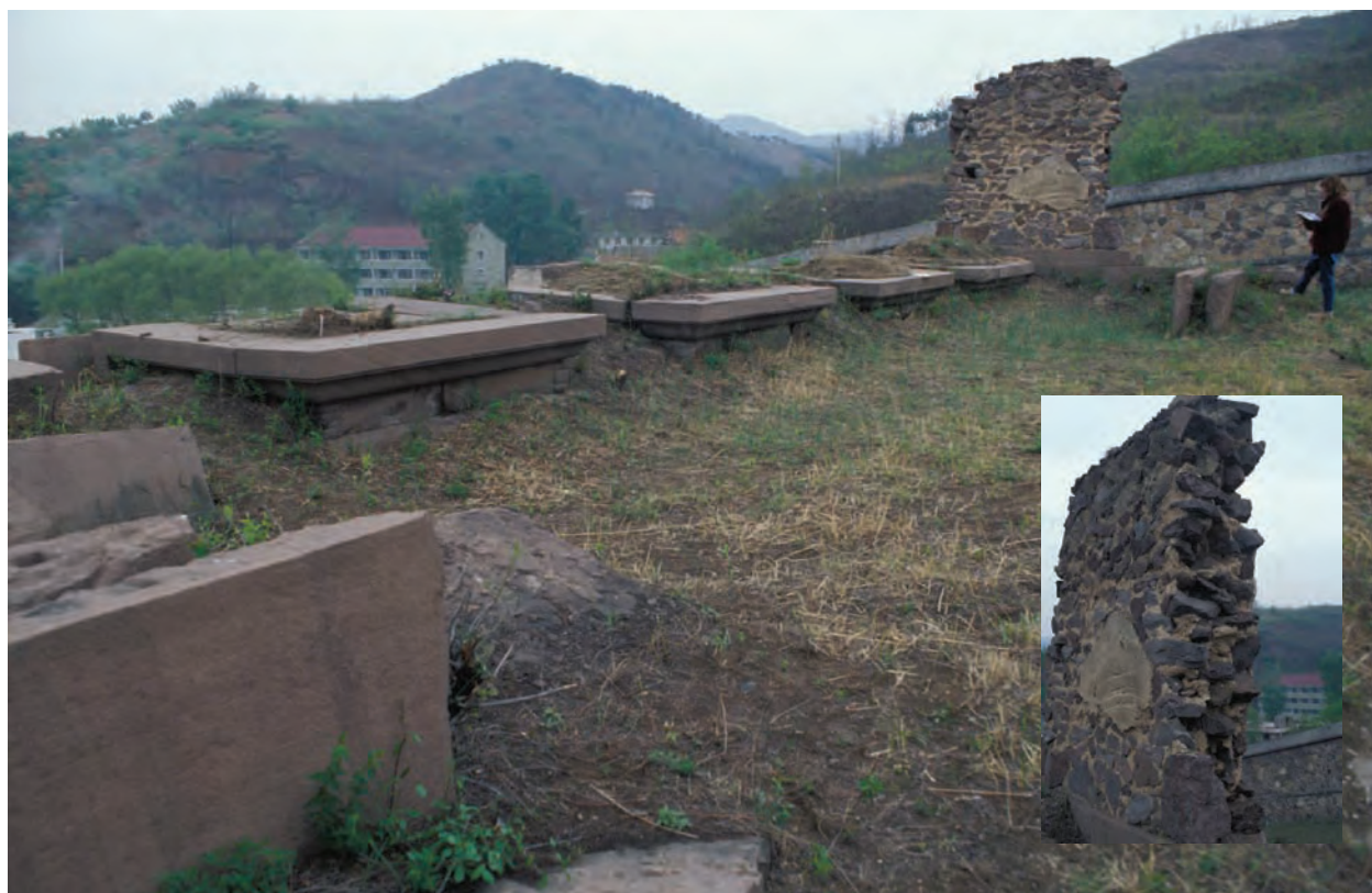
107. 慧喜殿及其毛石砌筑墙的细部（朝西北） Huixi Hall, looking NW, with detail of rubble masonry wall
