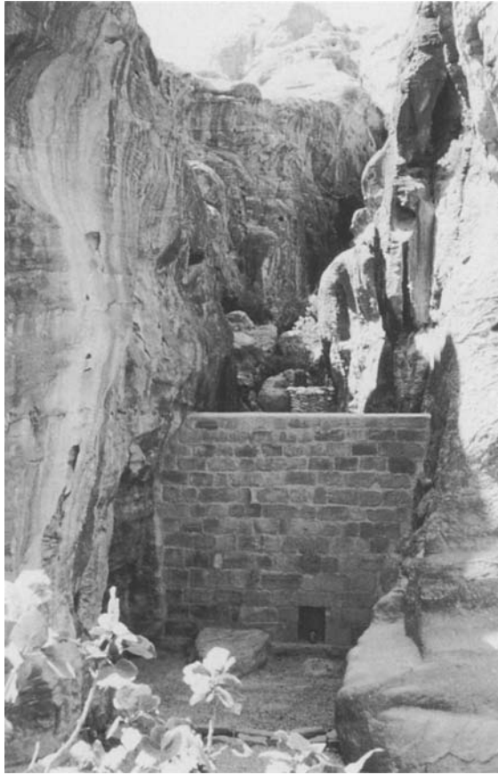
Figure 7 The Wadi Madrass Dam, which flanks the Siq in Petra.
