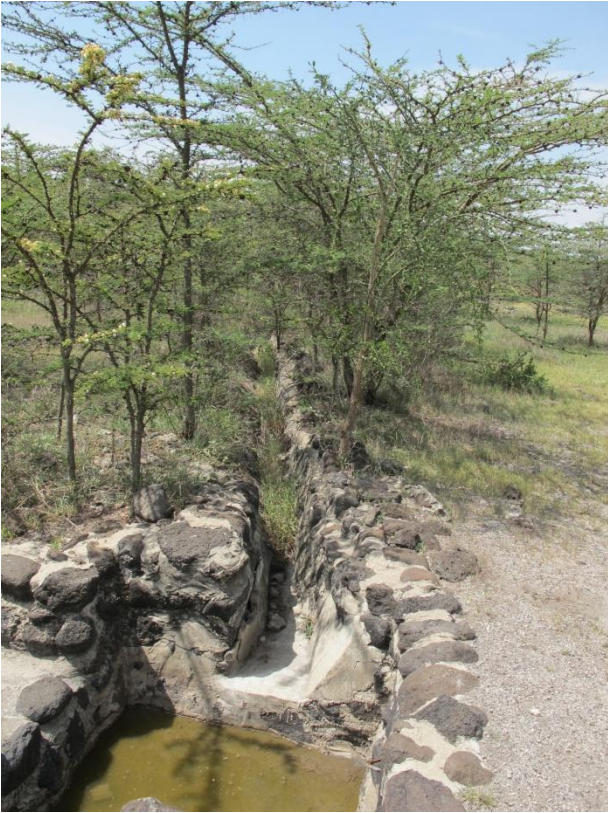
Extensive growth of acacia trees adjacent to drainage channel, which is clogged with vegetation. Catchment sump in foreground.
