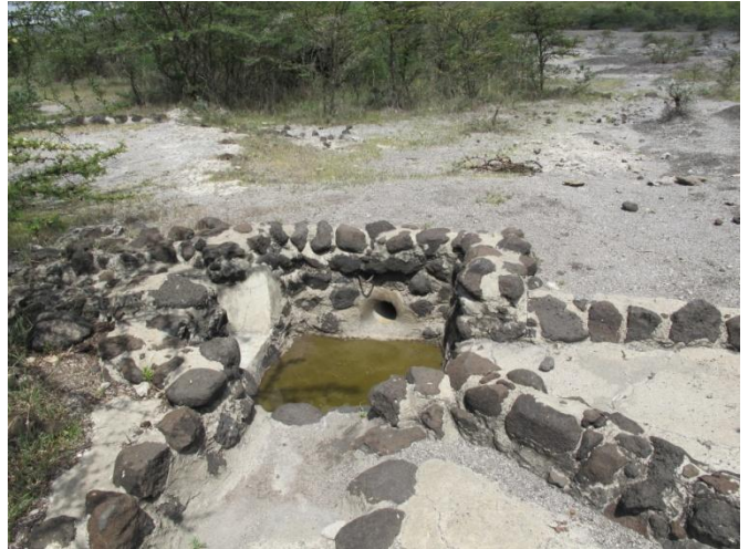
Catchment sump. Steel grill to prevent outflow pipe from clogging with vegetation is missing.
