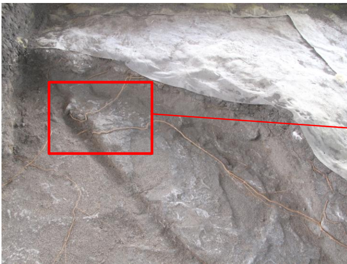
Roots penetrating tuff at edge of Fault 1. Root penetration in conjunction with excavation dislodged a piece of the tuff.
