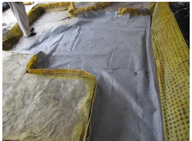
Geotextile in place over Layer 1.
