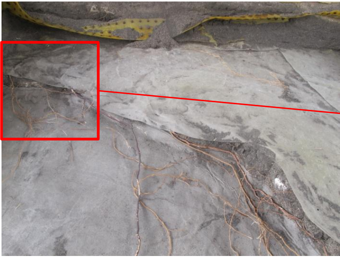
Roots running above geotextile along the Augite Biotite scarp. Roots found easy access below geotextile where 2 pieces of geotextile met at the top of the Augite Biotite scarp.
