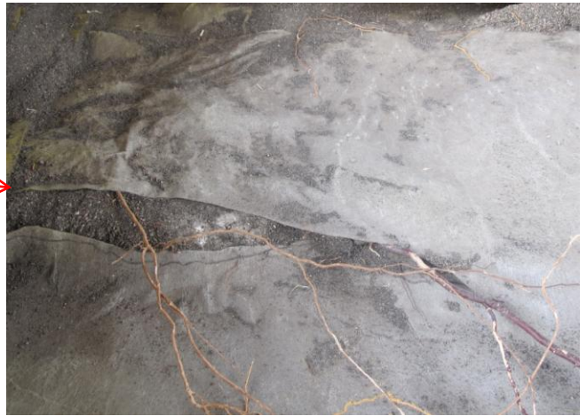
Roots running above geotextile along the Augite Biotite scarp. Roots found easy access below geotextile where 2 pieces of geotextile met at the top of the Augite Biotite scarp.
