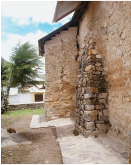
FIGURE 8 A perimeter stone walkway diverts water from the foundation walls.
