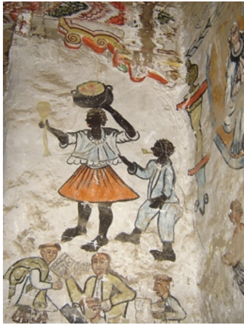
FIGURE 7 Typical vertical seismic cracks at the wall intersections, Church of Rapaz.
