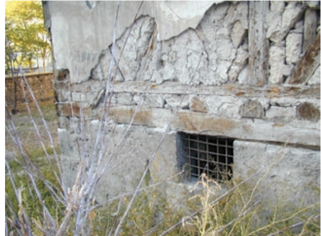
FIGURE 2 Detail of a hımiş building with earthen block construction.
