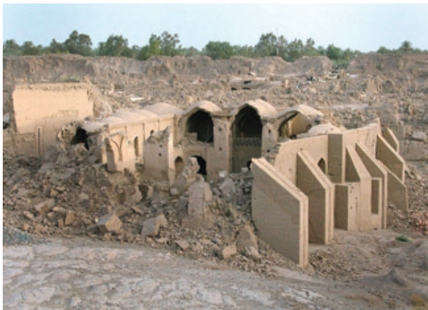
FIGURE 14 Building collapse due to earthquake, Bam, Iran, 2003. Photo: © Randolph Langenbach, 2004.
