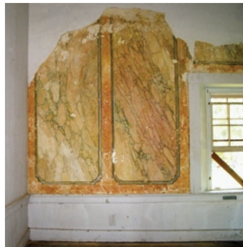
FIGURE 7 Conserved sala wall, de la Ossa Adobe, Los Encinos State Historic Park. This decorated surface was discovered beneath later paint layers. Photo: Courtesy of Karen Hildebrand, California State Parks.
