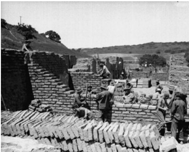
FIGURE 9 The Convento of La Purisima Mission, under reconstruction in 1935. The Civilian Conservation Corps documented building materials and structural work photographically. Photo: Courtesy of California State Parks, 2007.
