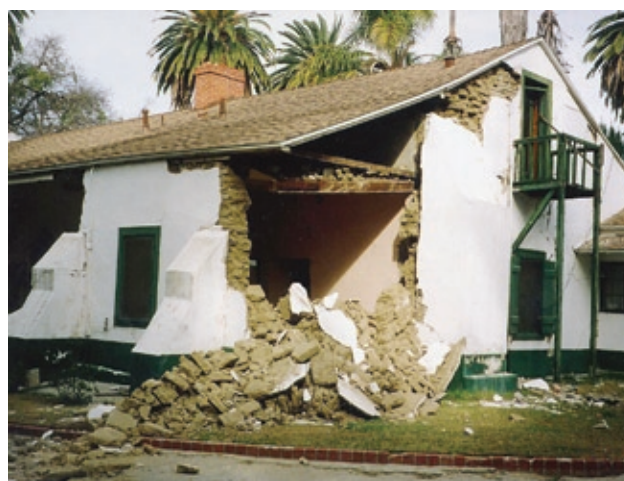
FIGURE 1 Main House, Rancho Camulos, damaged during the 1994 Northridge earthquake. Photo: E. Leroy Tolles, ELT and Associates.
