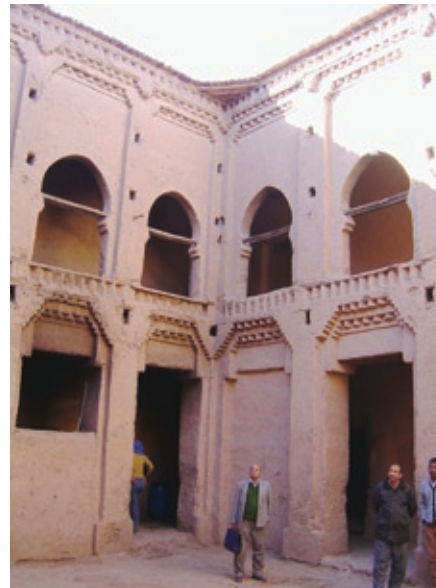
FIGURE 8 Interior of a house, Tanmougalt.
