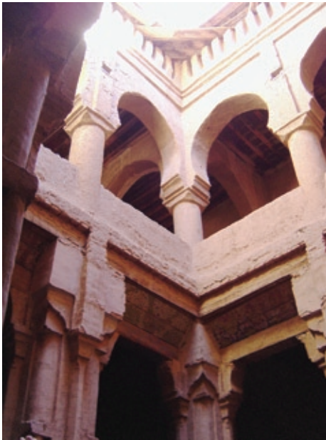
FIGURE 7 Interior of a house, Tanmougalt.
