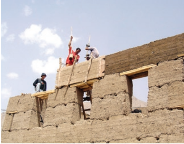
FIGURE 12 Building a rammed earth wall today, Ait Bouguemmaz (notice joint defects).
