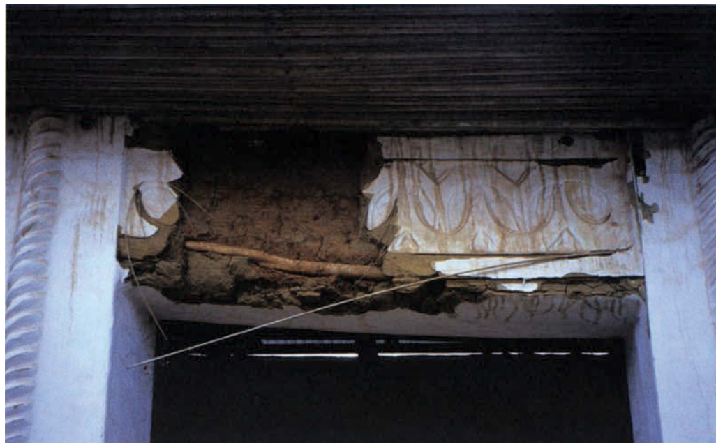
FIGURE 3 Decorated beam, damaged after the displacement of a roofing sheet during a rainstorm (Patakro shrine). Photo: Sébastien Moriset, CRATerre-EAG.
