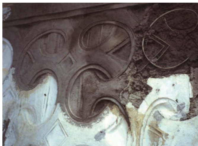
FIGURE 6 White wall during restoration, showing the palm stick reinforcements inserted in the clay (Edwenase shrine). Photo: Sébastien Moriset, CRATerre-EAG.
