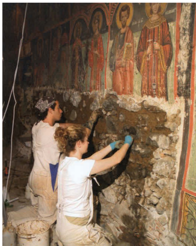
FIGURE 6 Repointing of the stone plinth using the tested repair mortar. Photo courtesy of the Courtauld Institute of Art, Conservation of Wall Painting Department, 2002.
