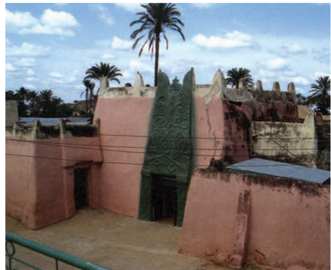
FIGURE 6 View of the Babban Gwani in 2003. Note the cracked plaster to the right of the decorated panel. Photo: Ishanlosen Odiaua.
