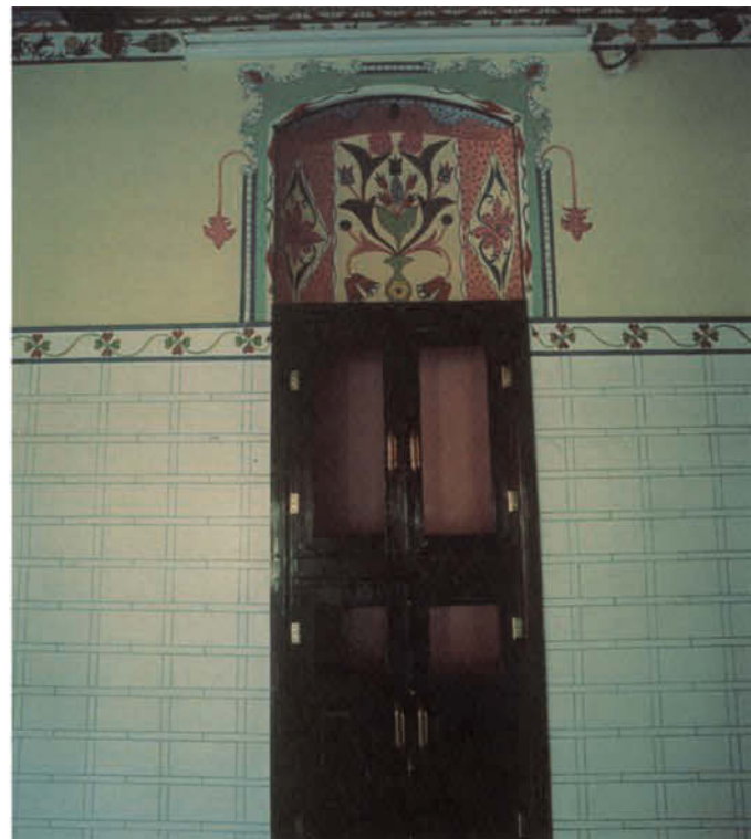
FIGURE 6 Malas , a form of highly burnished lime plaster, is a labor-intensive interior finish. In this contemporary example from the ba-Zaraah house in Khoreiba, Wadi Do’an, the malas has been scored to resemble ceramic tiles.
