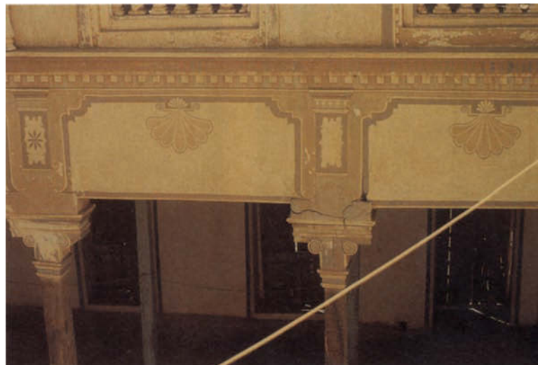
FIGURE 2 Lime-plaster decorations are sometimes applied directly to mud-plastered surfaces, as in this example of the water tower from the al-Hawta Palace Hotel, Wadi Hadhramaut.
