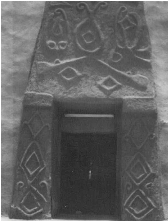
FIGURE 5 Babban Gwani in 2002. Note the detached cement plaster at the base of the left pillar. Photo: Ishanlosen Odiaua.
