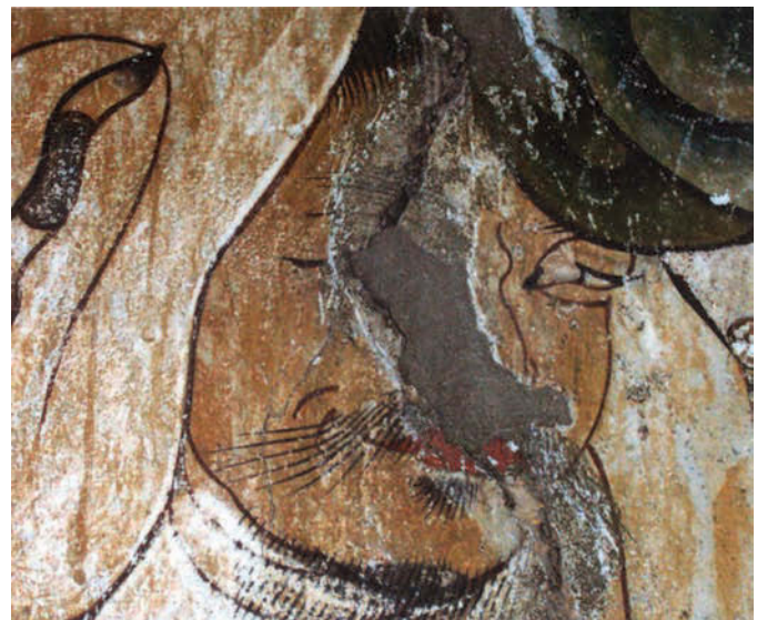
FIGURE 5 Yong'an Temple. Cement fills added by nonprofessionals in the 1970s have caused deterioration of the wall paintings. Photo: Jun Zheng, 2000.
