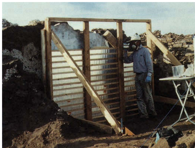
FIGURE 5 The rectangular timber frame in place, supported by an A-frame at each end (February 2003). The process of building up the shuttering and pouring in the polyurethane foam is two-thirds complete. Courtesy of the Egypt Exploration Society.
