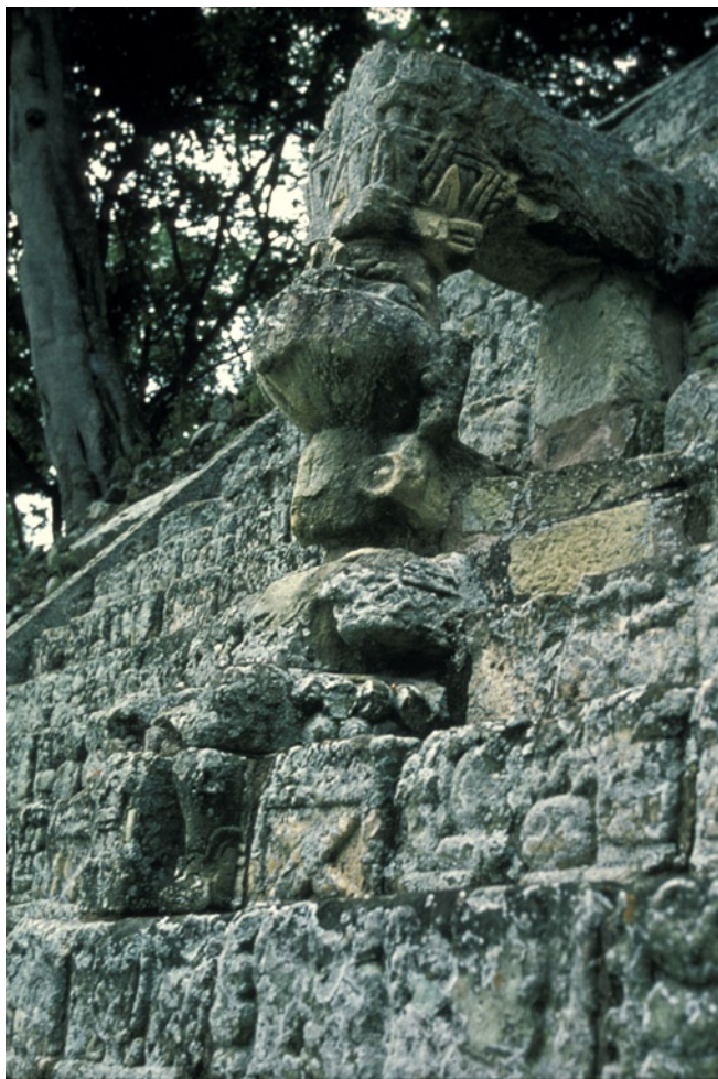
Figure 52 Hieroglyphic Stairway Seated Figure 5 before biocide treatment, showing heavy biological colonization. 1975.
