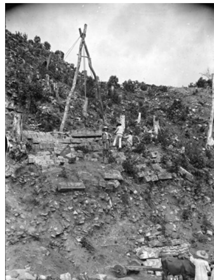
Figure 18 Fallen section of the Hieroglyphic Stairway being lowered to the Plaza block by block. George B. Gordon, director of the Peabody Museum expedition, is seen in center. 1895.
