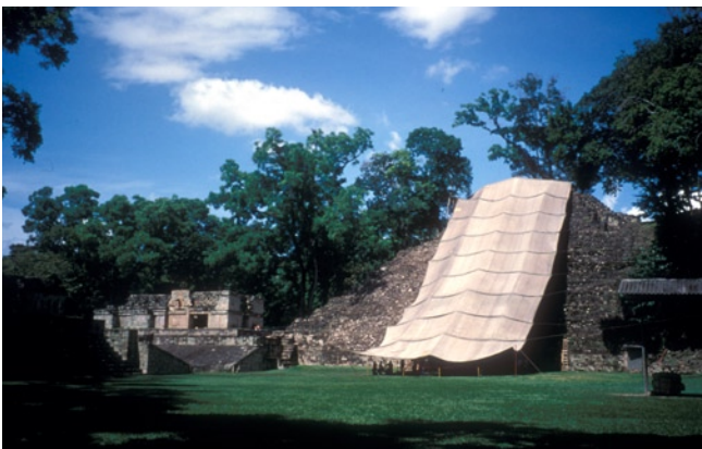
Figure 37 Structure 26, showing the extension of the larger tarpaulin over the Hieroglyphic Stairway. 2000.
