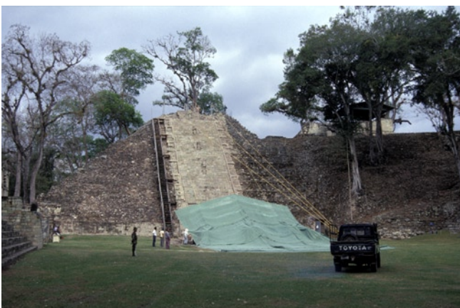
Figure 38 Replacement of the tarpaulin above the Hieroglyphic Stairway. 2005.
