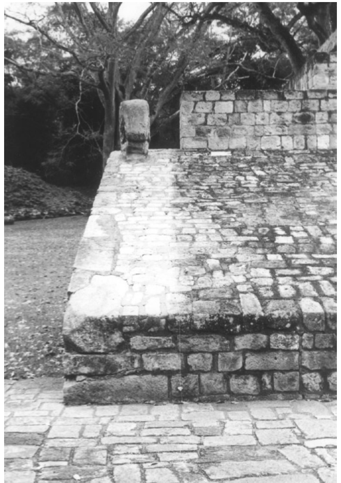
Figure 31 A one-meter-wide test strip at the south end of the Ballcourt, after treatment by Mason Hale. Note the loss of black algae. Ca. 1978.
