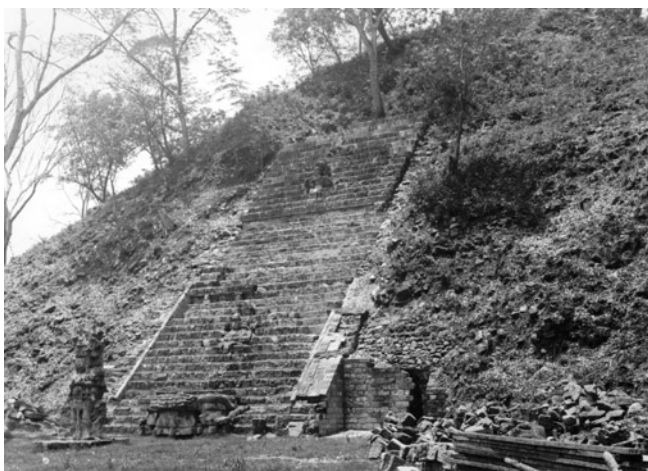
Figure 27 The Hieroglyphic Stairway looking northeast during reconstruction, showing the few hieroglyphic blocks that were reset on the north side of steps 18–21 during this season. 1958.
