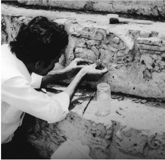
Figure 34 Reattachment of fallen stone flakes with Paraloid B-72, block 28, step 7. April 1982.
