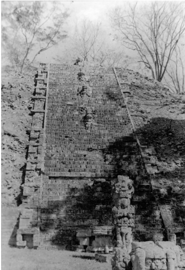
Figure 28 The Hieroglyphic Stairway looking east, after its complete reconstruction. 1942.
