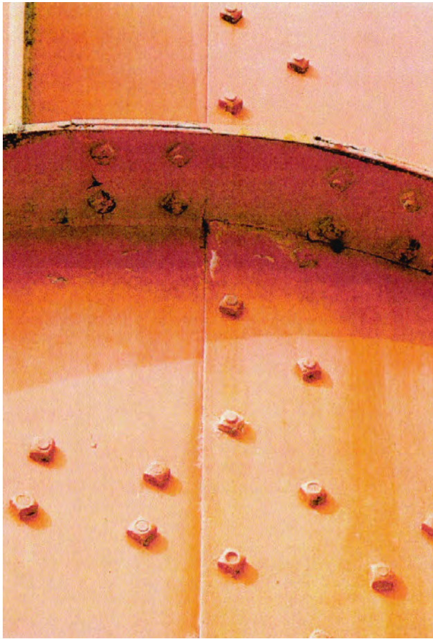
Figure 7 Photo of the west-facing side, showing rust and runs. © 2014 Calder Foundation, New York / Artists Rights Society (ARS), New York. © ZMK, Hannover 2003.
