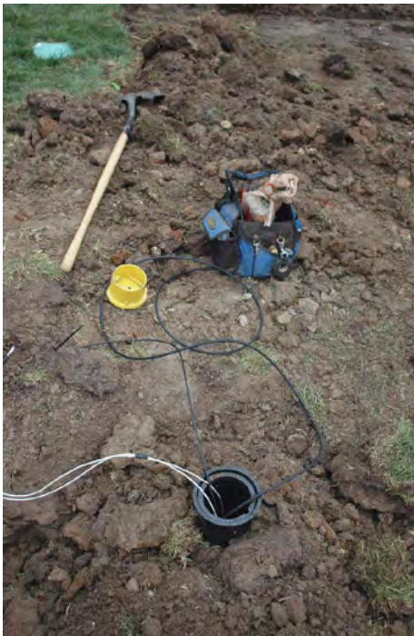
Figure 12a The test station, consisting of a PVC tube buried in the ground near the sculpture. The cables are attached to a circuit board and placed inside the tube.
