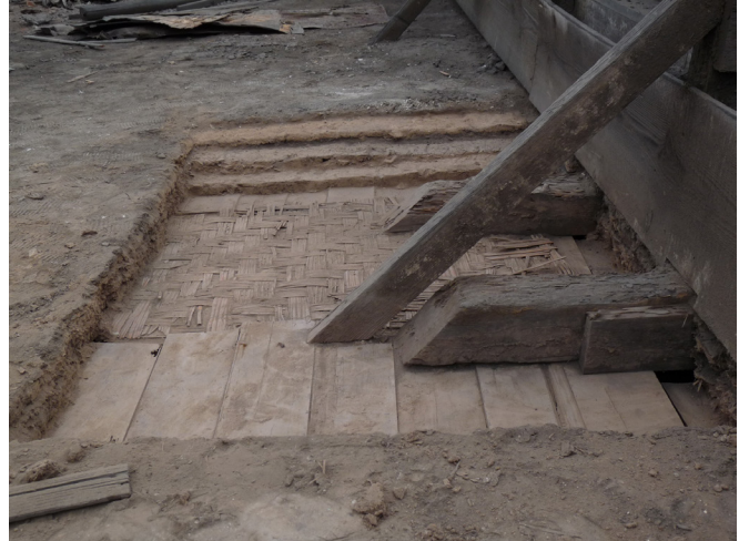
FIGURE 3.42 Prospection IVR-1, showing the roof construction at the northwest façade. Image: Mirna Soto, for the GCI.
