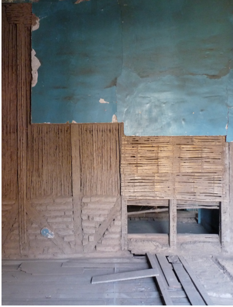
FIGURE 3.25 (ABOVE) Typical quincha wall at the second floor, showing the mud and fired brick infill at the bottom of the frame (prospection IIS-2). The horizontal canes at the right have been used to infill an earlier door opening. Image: Mirna Soto, for the GCI.
