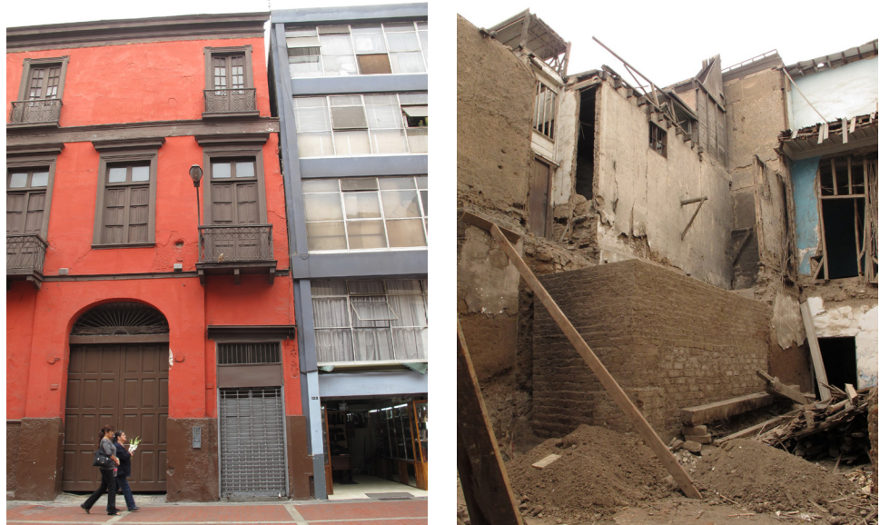
FIGURE 3.10 (LEFT) Northwest façade of Hotel El Comercio along Jirón Carabaya, and adjacent concrete structure, 2010. Image: Amila Ferron.
