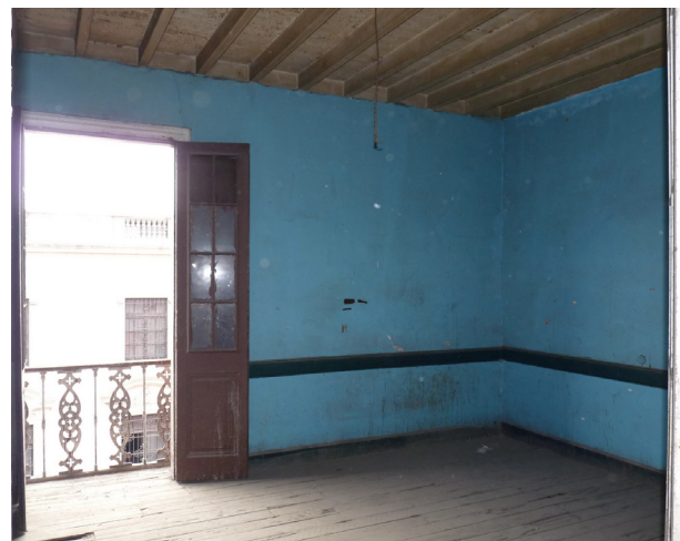
FIGURE 3.17 Typical third floor room (room 306), with doors providing access to the balcony. Image: Mirna Soto, for the GCI.
