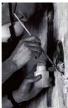
FIGURE 13. REMOVAL OF OLD GAUZE FACINGS.
