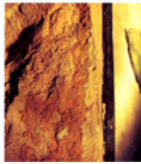
FIGURE 2. STRATIGRAPHY OF CLAY-STRAW PLASTER LAYERS ON THE SOUTH FACE OF COLUMN II. THE LEVELING PLASTER IS COARSER AND DARKER THAN THE UPPER LAYER.
