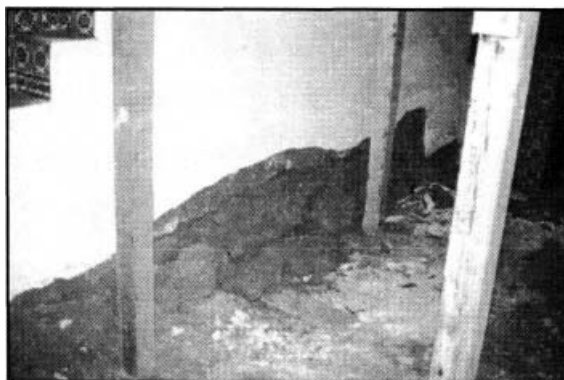
Figure 10.5. Slumping at the base of the east wall. The east wall also suffered considerable water damage that resulted in slumping and bulging of the wall at the base.
