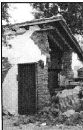
Figure 3.29. Andres Pico Adobe garage structure. Failure was defined by cracks at the door and window openings. Also see Figure 3.23.
