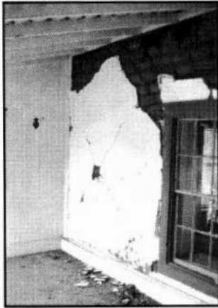
Figure 7.3. Crack damage in the south second-floor wall near the southwest corner. X-shaped cracking across this panel indicates shear failure.
