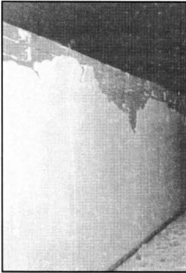
Figure 5.15. Interior of the east wall at the second-floor level. Damage to the plaster on the upper section of the wall, but there was no evidence of slippage between the wall and the roof framing.
