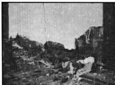
Figure 5.16. Base of west wall. Wall has suffered strength loss due to repeated wet-dry cycles. Plaster and adobe have spalled, but the wall has not slumped, nor has the stability of the wall been threatened.
