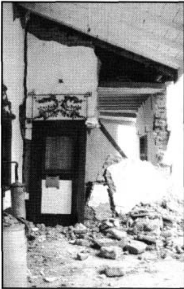
Figure 4.8. West wall of Ramona's room. The majority of this wall collapsed leaving only the section of wall that is above the door.
