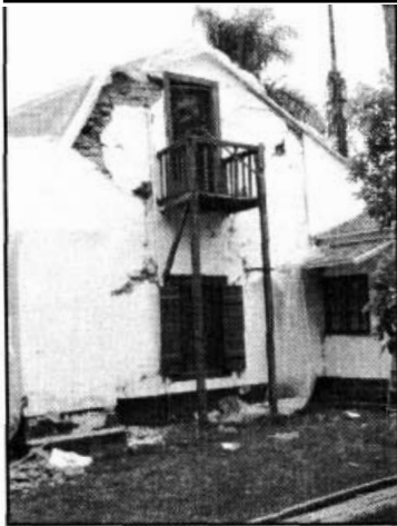
Figure 4.10. Gable-end wall of the south wing. The crack damage to this wall was extensive with cracks emanating from the corners of the door and window. Some restraint is provided on the inside of the wall by interior paneling.
