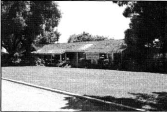
Figure 12.17. Front elevation of the Centinela Adobe.
