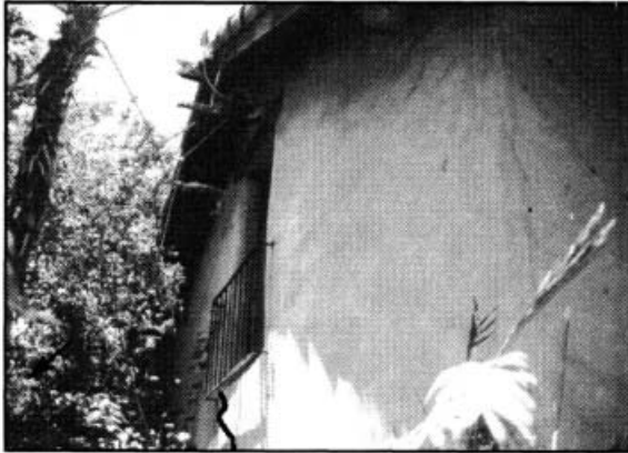
Figure 12.14. Rocha Adobe. Minor cracking in the south gable-end wall visible below the balcony railing.
