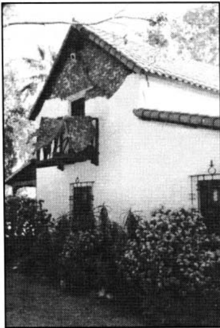
Figure 5.12. North gable-end wall. The north gable wall suffered some damage but not as severe as the south end. A large diagonal crack extends from the peak of the gable down to the intersection with the lower roof on the right in the photograph. A large section of the plaster fell and damaged the balcony
