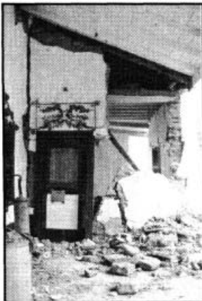
Figure 3.36. Collapsed wall of Ramona's room at Rancho Camulos. This thin, 12-inch-thick wall collapsed downward rather than falling outward. Moisture damage at the base of the wall contributed to the failure.
