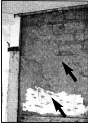
Figure 7.11. Southeast corner at the first-floor level. The damage is significantly more severe on the second-floor level directly above (Figure 7.7). The photograph shows a vertical crack at the interface of the two perpendicular walls and a diagonal shear crack that extends down to the right.
