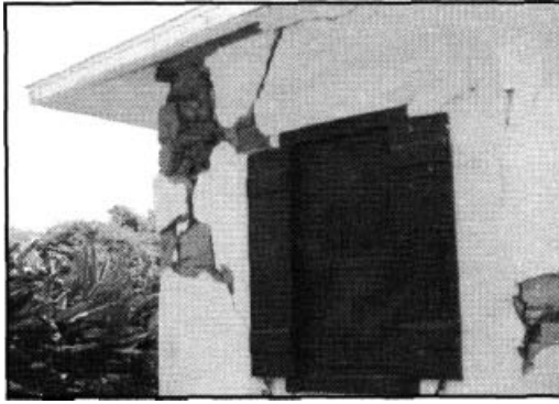
Figure 4.2. Northwest corner of the west wing. Damage at the corner of the stone wall.
