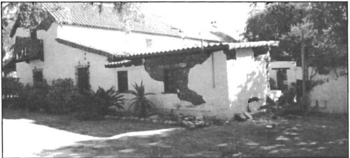
Figure 5.14. Collapsed garden wall on the north side of the courtyard, plaster damage along the north wall, and damage to the north gable-end wall.
