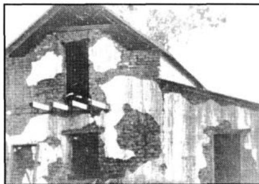
Figure 5.2. The Andres Pico Adobe north wall before reconstruction, approximately 1930 (source: San Fernando Valley Historical Association).
