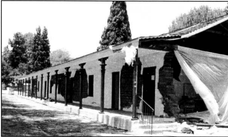
Figure 6.6. Southeast corner of the De la Osa Adobe. Collapsed gable-end wall is visible on the right.
