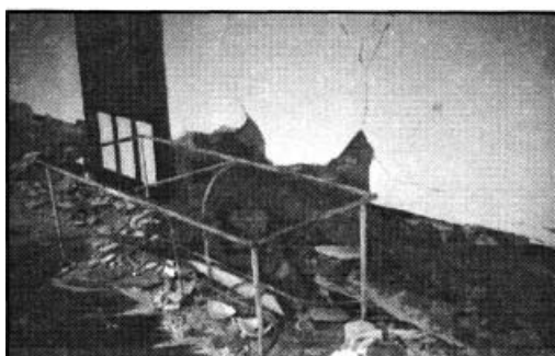
Figure 3.38. A similar spalling of adobe and stucco on the exterior wall at the Del Valle Adobe at Rancho Camulos.
