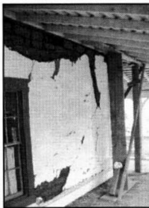
Figure 7.4. Crack damage in the south, second-floor wall near the southeast corner. The diagonal crack indicates a probable shear failure.
