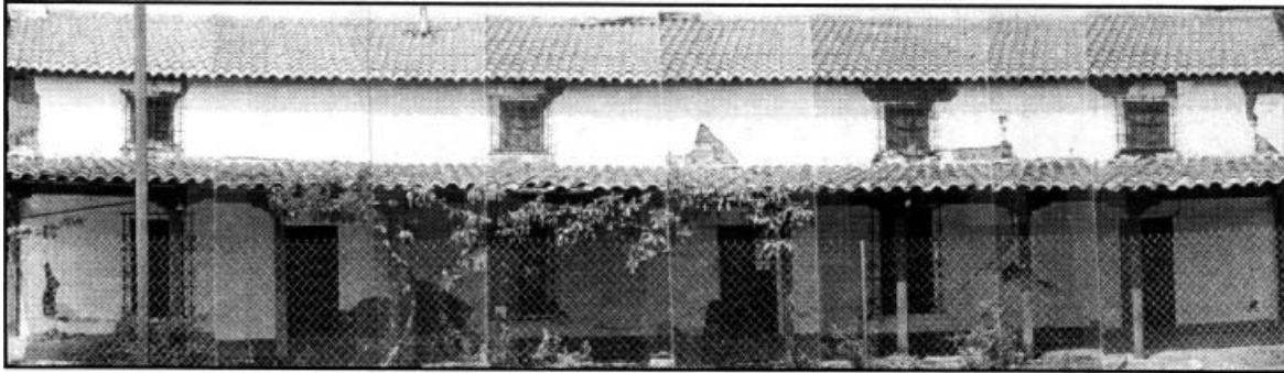
Figure 5.7. East elevation. The damage to the east wall was largely defined by out-of-plane flexure of the walls. Cracks developed vertically at the end walls at the two interior cross walls (cracks highlighted in Figure 3.8).
