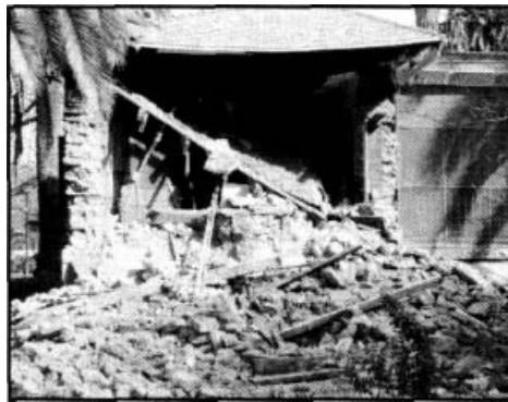
Figure 4.6. Southwest corner bedroom. The south wall collapsed and the east and west walls of this room were also seriously damaged with large cracks and permanent offsets.
