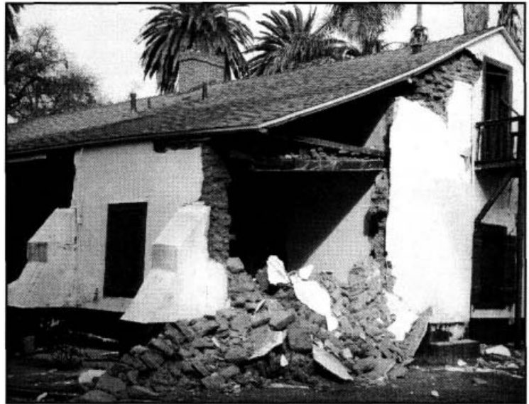
Figure 4.9. Southeast corner of Ramona's room. The buttresses on the south wall prevented collapse of that wall. The east wall of Ramona's room collapsed during the earthquake. The gable-end wall did not collapse but suffered serious damage (more details are shown in Figure 4.10).
