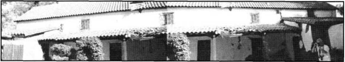
Figure 5.4. West elevation. The chimney collapsed and fell through the porch roof. There is damage to the west wall at the reentrant corners where the lower roofs intersect the west wall.
