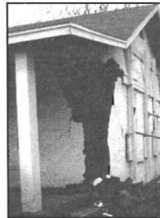
Figure 12.22. Sepulveda Adobe. Vertical cracks at the corner led to collapse of the corner section.
