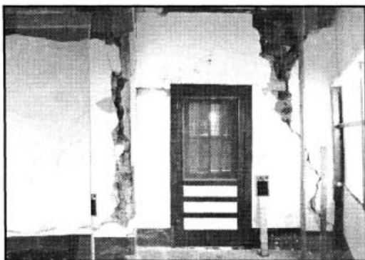
Figure 4.1. Northeast corner of west wing. Damage at the corner of the stone wall and at the interface between the stone and the adobe.
