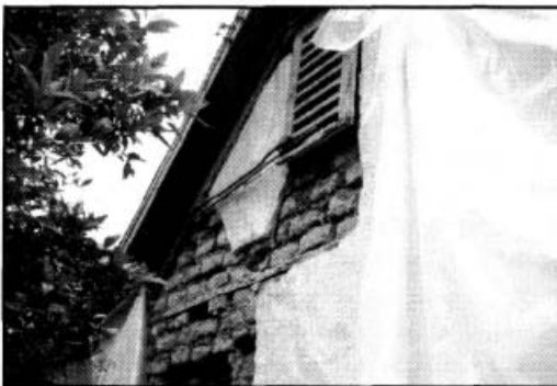
Figure 10.2. North gable-end wall. Plaster spalled from the exterior surface. A crack extends along the horizontal wood plate embedded in the adobe at the ceiling level. The roof rafter at the top of the wall provides some restraint against overturning of the upper section of the gable end.
