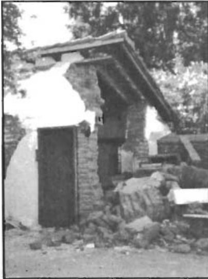
Figure 5.13. Collapsed section of garage in the southwest corner of the courtyard.
