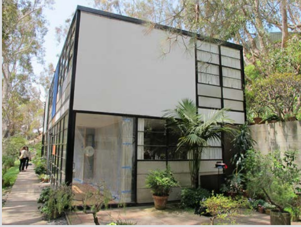
FIGURE 2.8A Eames House paint excavation location: House_north.
