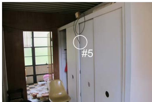
FIGURE 4.11D Top of stairs sensor location, 2012. Photo: Shin Maekawa
