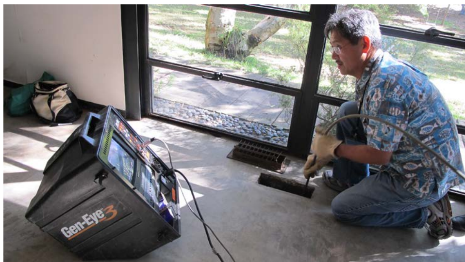
FIGURE 4.25 Shin Maekawa inspecting the heating ducts, 2011. Photo: Ana Paula Arato Gonçalves
