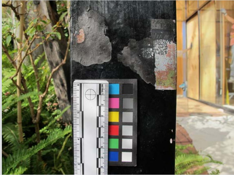
FIGURE 2.10B An additional excavation was performed on beam 4D. A cross section sample was taken but was not imaged in 2013, at the time this report was prepared.
