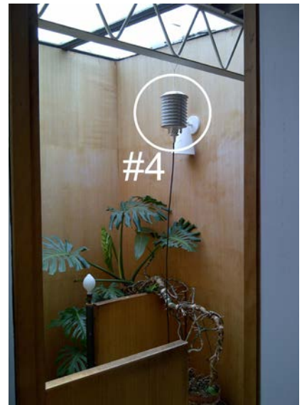
FIGURE 4.11E North closet on the second floor location, 2012. Photo: Shin Maekawa
