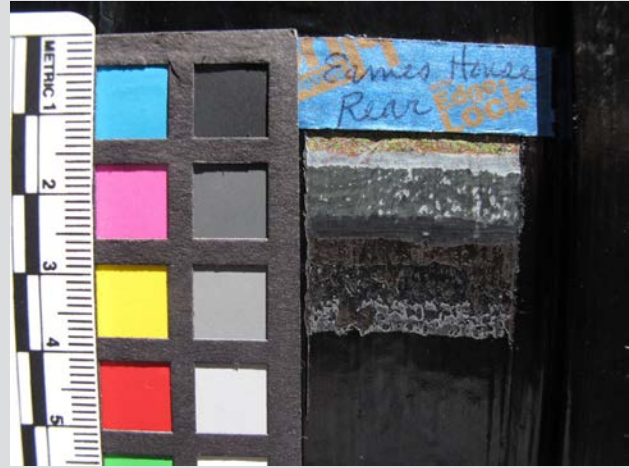
FIGURE 2.11B House_north, in situ paint excavation exposure window.
