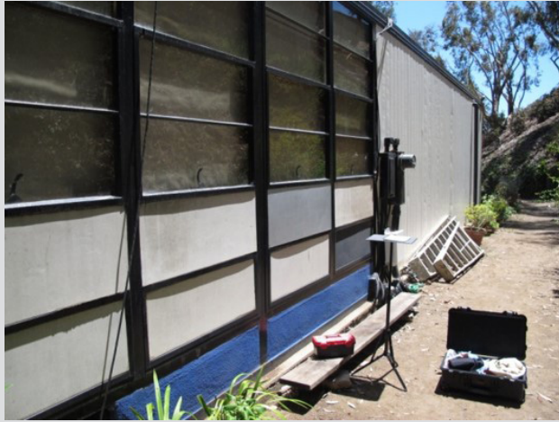
FIGURE 2.11A Eames House paint excavation location: House_west.
