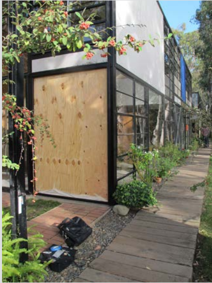
FIGURE 2.10A Eames House paint excavation location: House_east_2
