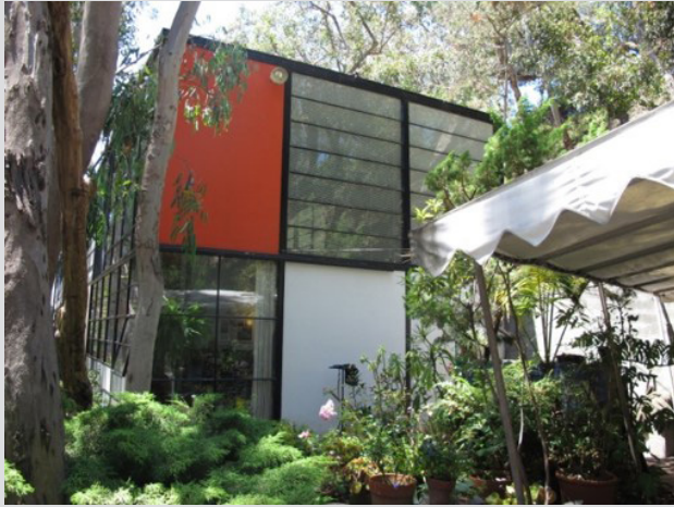
FIGURE 2.12A Eames House paint excavation location: Studio_north.
