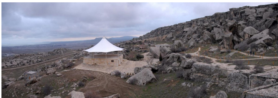
FIGURE 6. Gobustan in Azerbaijan. Left: toilet facilities. Right: part of the walkway system.
