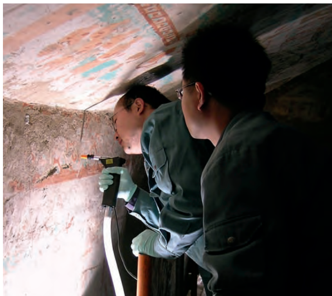
FIGURE 6 An ultrasonic humidifier being used to dissolve surface salts on the treated area of a wall painting. Photo: S. Rickerby
