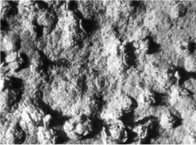
FIGURE 8 Salt eruption on the unpainted clay plaster.
