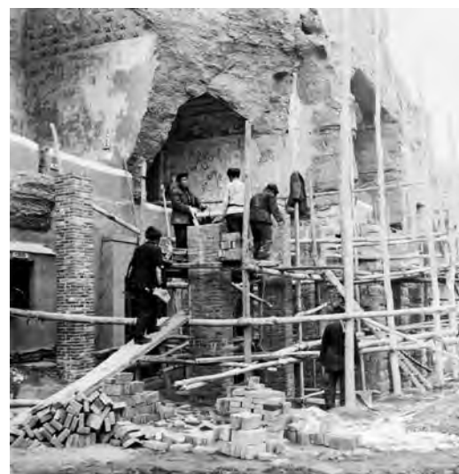
FIGURE 3 Cave 85 during construction of facade and walkways (1957–58). Pillars were built in front of the cave to support a wooden walkway and provide support to the fronts of caves 242 and 243.
