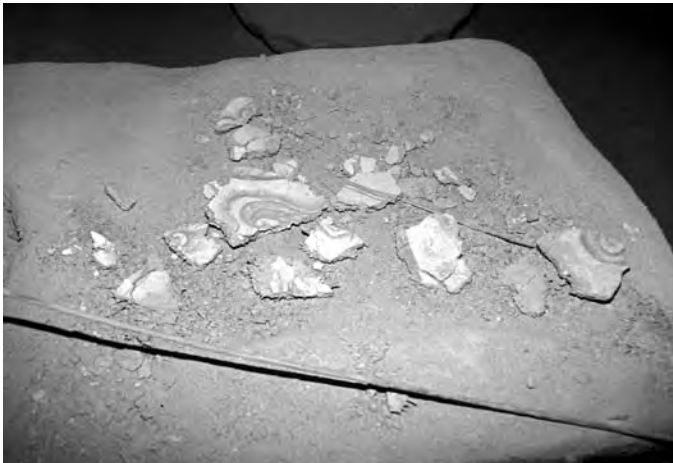
FIGURE 5 Detachment, followed eventually by collapse, is a widespread problem. Here, fragments of painted plaster lost from the west slope in 1996 near an anchor installed in the 1970s. Credit: J. Paul Getty Trust
