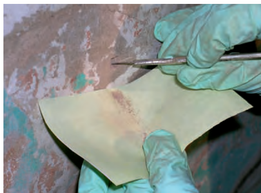
FIGURE 6 Plaster microcores being sampled as part of a comprehensive salt survey. Each core was taken at four or five incremental depths into the upper 10 millimeters of the wall where paint has been lost. The samples were analyzed to identify ions of soluble salts present and their topographic and stratigraphic distribution throughout the cave.
