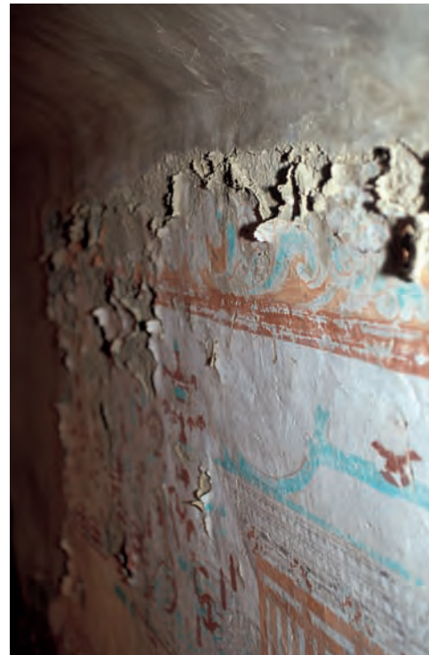
FIGURE 4 Exfoliation, the lifting of paint, ground, and upper plaster layers, apparently exacerbated by treatments for flaking (in the 1970s) using polyvinyl acetate and polyvinyl alcohol fixatives. The continued loss of painting indicates that this problem is ongoing, most notably at the northwest end of the cave.
