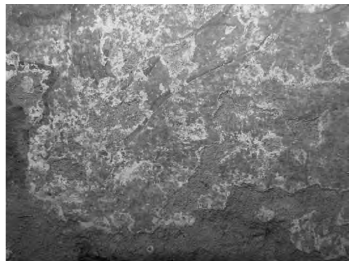
FIGURE 7 Flaking and paint loss.
