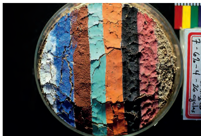
FIGURE 5 Clay coupon, simulating the structure, composition, and pigments of the wall paintings, showing typical salt-related deterioration after 26 cycles of high and low RH fluctuations in an environmental chamber. Photo: J. Paul Getty Trust
