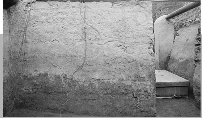
Structure 4 at the site. The earthen wall displays the effects of rising water—among them, the development of microgrowth, disintegration, cracking, and detachment. Photo: Urs Muller.
