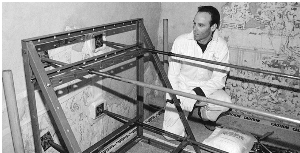
During the field campaign at Mogao, presses were installed on a temporary basis to hold in place fragile areas of detached plaster. The presses will also help during the injection of adhesive grouting by providing gentle pressure to re-adhere the plaster. Photo: Francesca Piqué.
