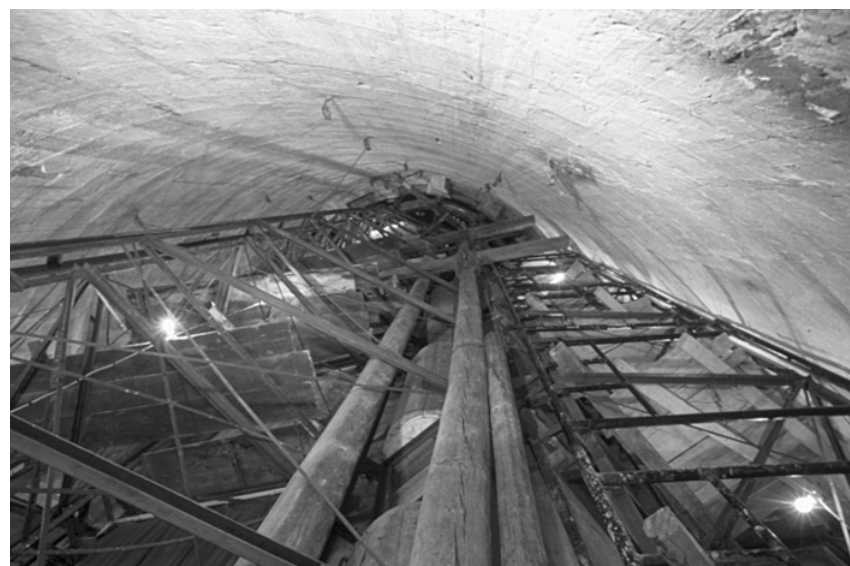
Rear view of the retablo and the interior stone wall of the apse, from the base looking upward. The large vertical poles are part of the original support system that no longer functions, due to the loss of base sections. Two of the three sections of the steel structure can be seen. (The horizontal boards on these structures provided temporary access for an initial inspection.) Photo: Lori Anglin.
