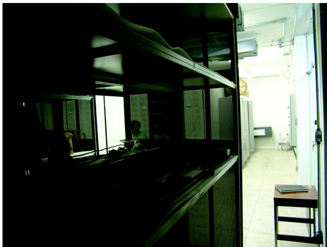
Figure 3 Side panels of a compact shelving system are made of perforated plate in order to allow air flow through the panel even in closed positions.
