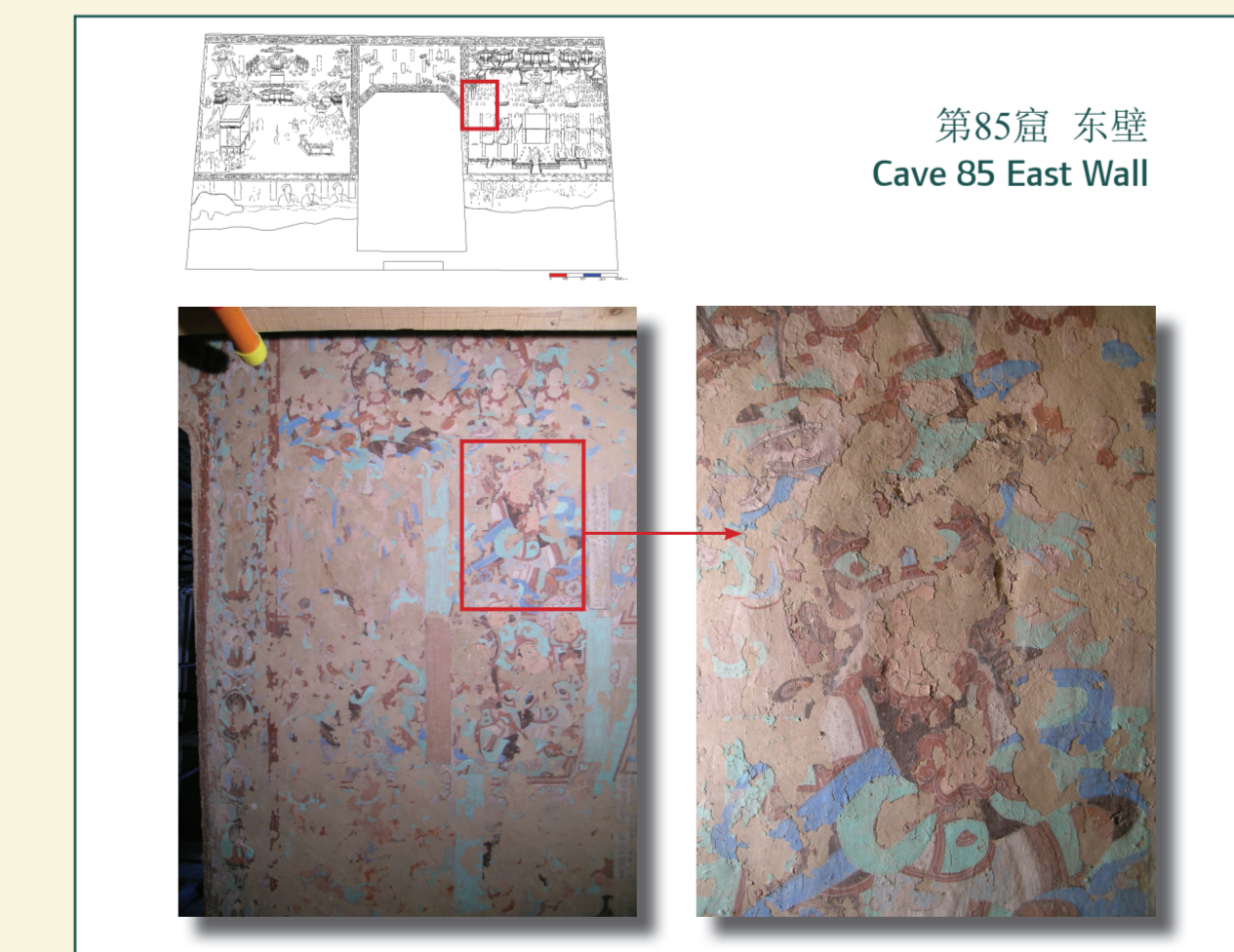
选择壁画区域进行定期现状监测。 Areas of the wall painting were selected for regular monitoring of condition.
