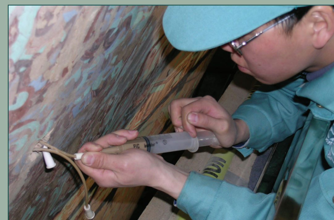
使用注射器和导管在壁画层后进行灌浆处理。 Injection of the grout mixture behind the painted plaster was done using syringes and catheter tubes.
