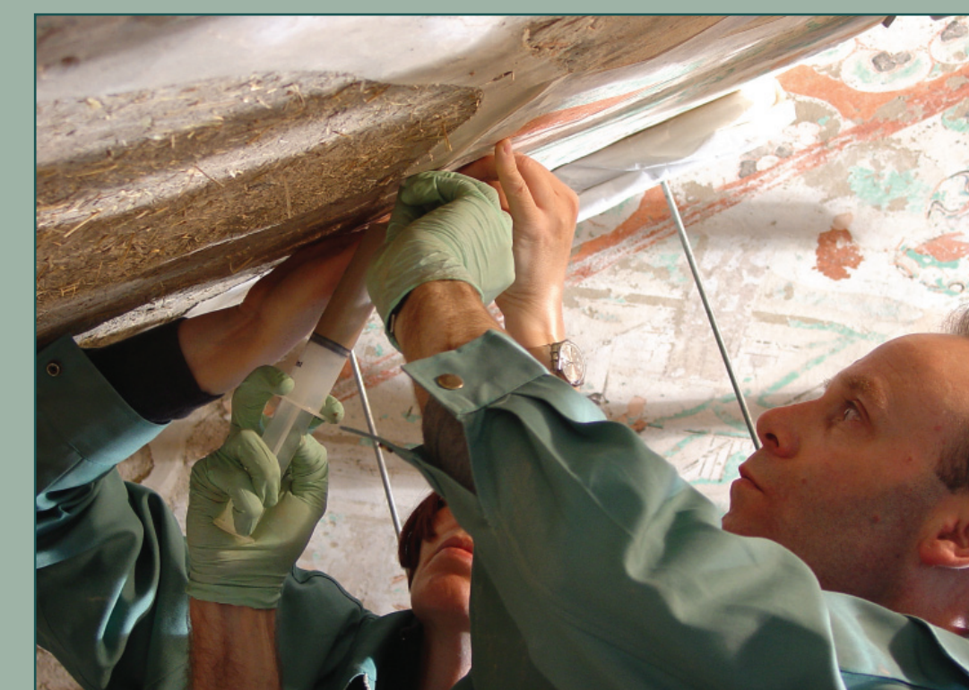
对整窟大面积的壁画层进行了灌浆处理。 Large areas of painted plaster were injected with the grout mixture throughout the cave.
