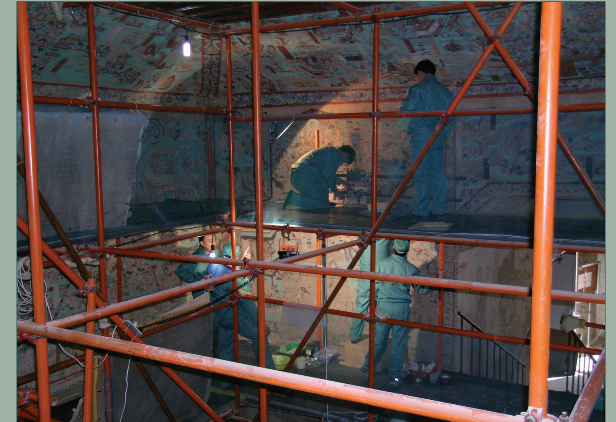
正在主室东壁进行保护工作。 Conservation work in progress on the east wall of the main chamber.
