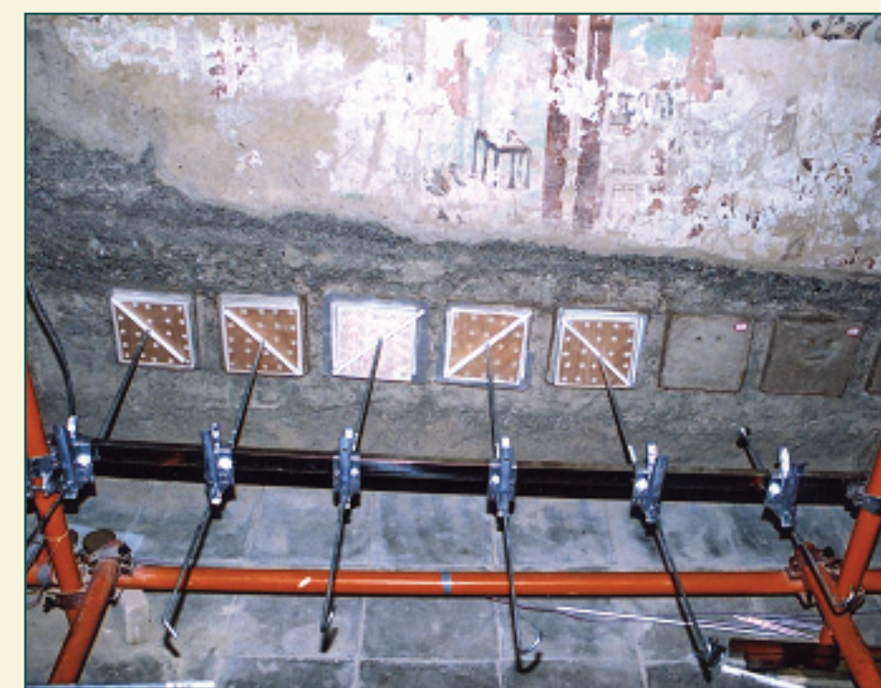
在第85窟内四壁下部的砂砾岩层（没有颜料层的区域）上粘结新的模拟地仗试块进行灌浆材料试验。 Testing of grout mixtures was undertaken in Cave 85 at the base of walls (in unpainted areas) by adhering modern plaster panels to the conglomerate.
