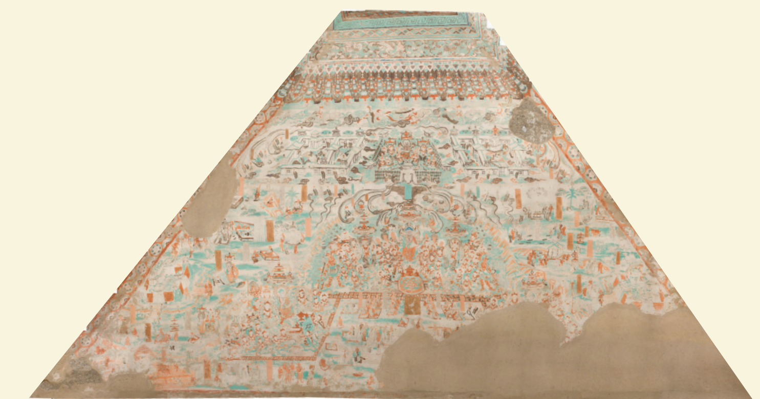
治理后的窟顶西披。没有对脱落的区域重绘，最大限度地添加新的地仗泥层，以避免人为增加水分（来自潮湿的地仗层），因为水分会造成可溶性盐在壁画层内运移。保留了早期保护工作中对地仗层的修复区域以及近年来因壁画脱落使砾岩裸露的区域（如1996年脱落的区域）。 The west ceiling slope after conservation treatment. Areas of loss were not repainted and new plastering was kept to a minimum in order to avoid the addition of water (from the wet plaster) which could redistribute soluble salts within the painted plaster. Instead, plaster repairs from earlier conservation work were left in place and recent areas of loss (such as the area of collapse from 1996) were left unfilled with the conglomerate exposed.
