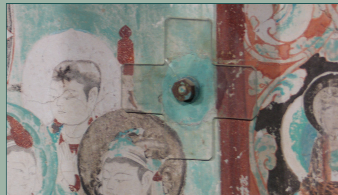
20世纪70年代，为防止壁画脱落进行了壁画锚固。上图显示仍然保留在主室北壁的锚固与垫板。 Anchors and bolts were inserted into the walls in the 1970's to secure areas of detachment. The anchor shown above was left in place on the north wall of the main chamber.
