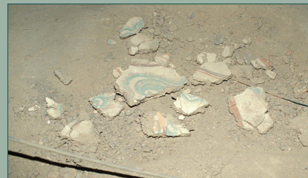
锚固只是用来对付壁画仍然继续脱落的一个权宜之计。1996年的残片脱落是在一段时间的高湿度之后发生的。 The anchors were only a temporary solution as areas of painted plaster continued to be lost. These fragments fell in 1996 after a period of high humidity.
