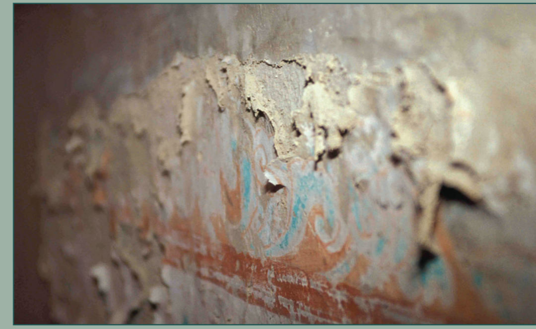
颜料层起甲与酥碱起甲。 Flaking and exfoliation of the paint layer.
