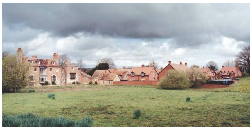
Fig. 3 The new constructions and the historic buildings of Henbury House, Dorset
