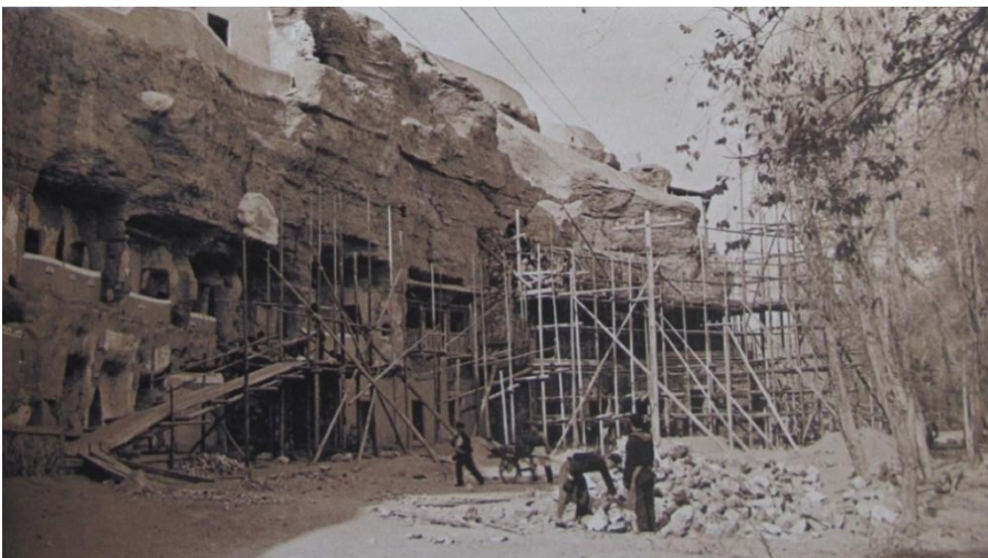
Fig. 4 Repair project at the Mogao Grottoes in the 1960s 8
