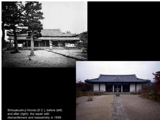
Shinyakushi-ji Hondo (8 C.), before (left) and after (right) the repair with dismantlement and reassembly in 1898
