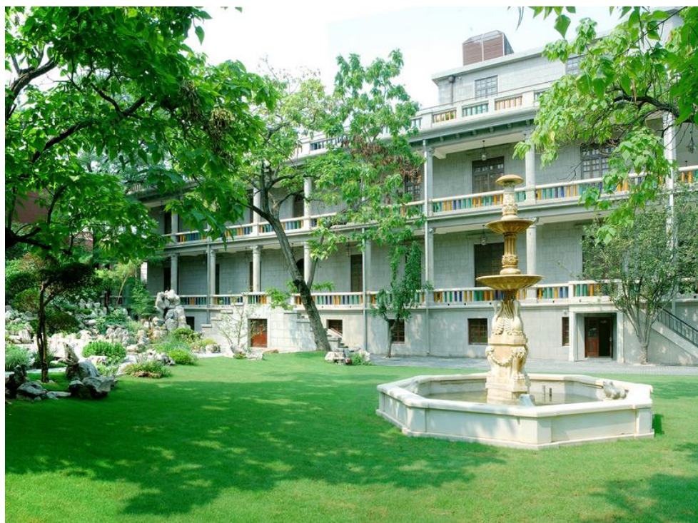
Fig. 4 Main building and garden of the former Prince Qing's Mansion ( http://www.tjhha.com/view_tjhha.asp?mod=15 )
