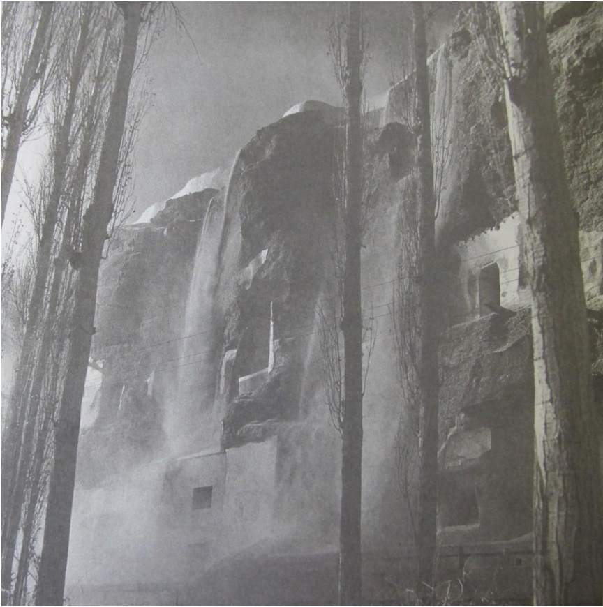
Fig. 3 Sand being removed from cliff edge in preparation at the Mogao Grottoes before the reinforcement project 7
