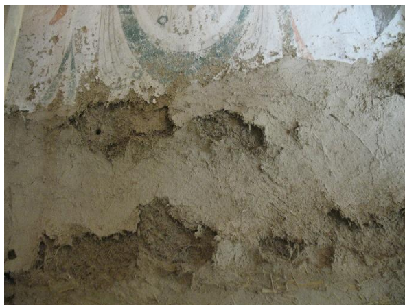
Fig. 1 Efflorescence (wall painting)
