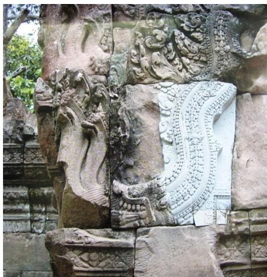
Fig. 9 Restored decoration on the southern entry tower of Chau Say Tevoda
