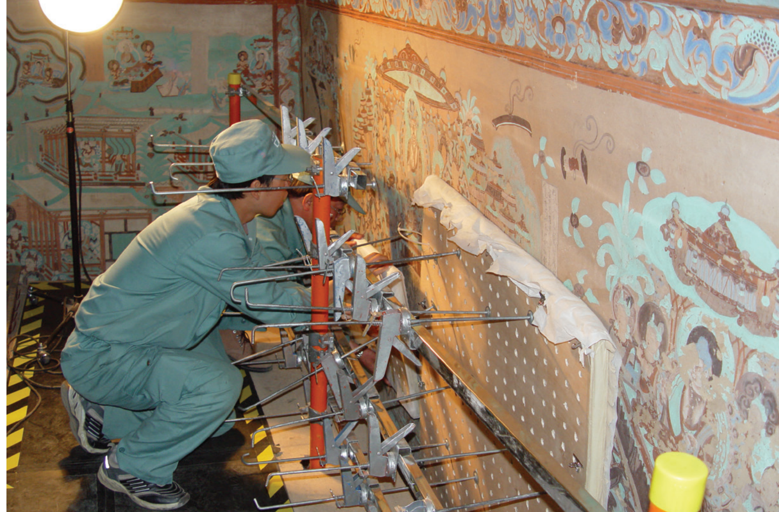
Top: After grouting, materials which absorb salts mobilized by water in the grout are applied to the surface of the painting and held in place with a press. The painting is monitored and the presses changed regularly until the grout has dried completely.
